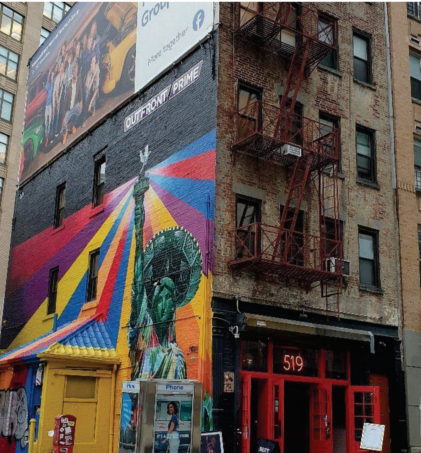
CURRENT VIEW OF EXTERIOR
