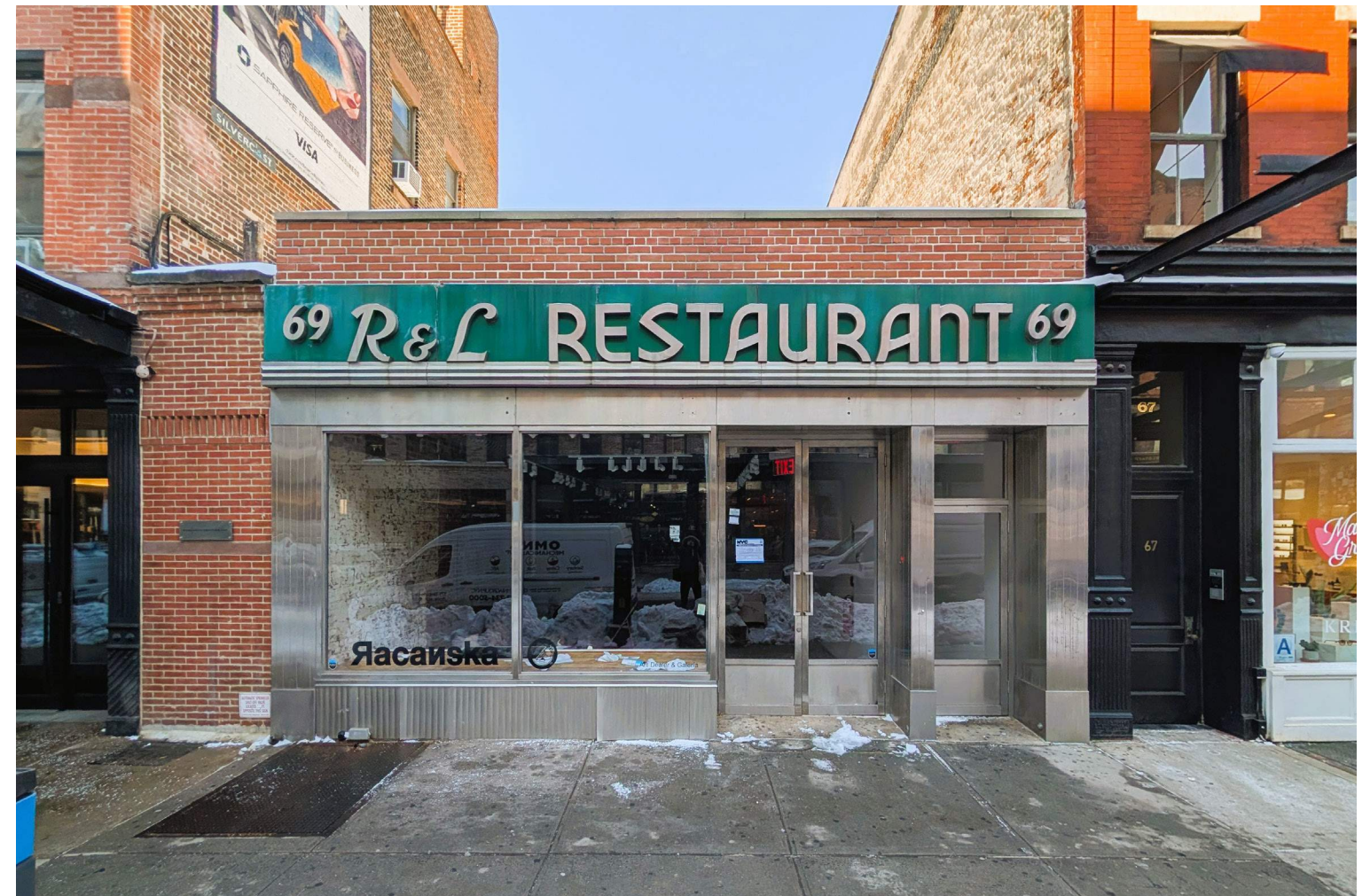
EXISTING SOUTH FACADE
