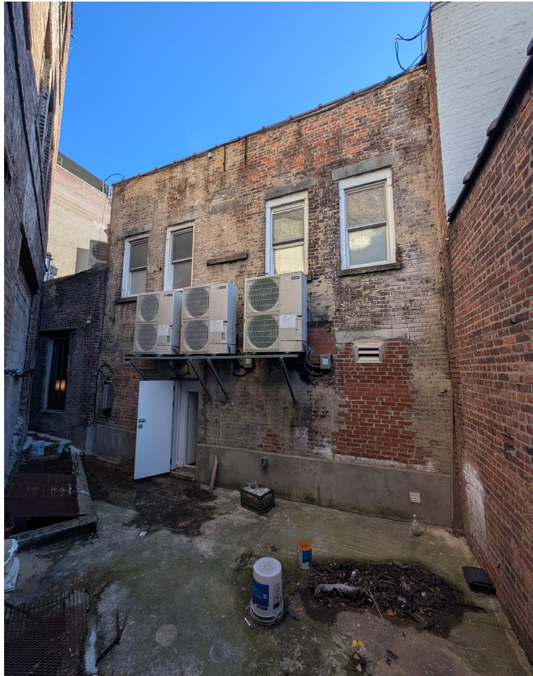
1 | NORTH ELEVATION - REAR FACADE
