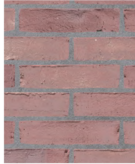
Beldin Belcrest 330 Brick at East and North Facade
