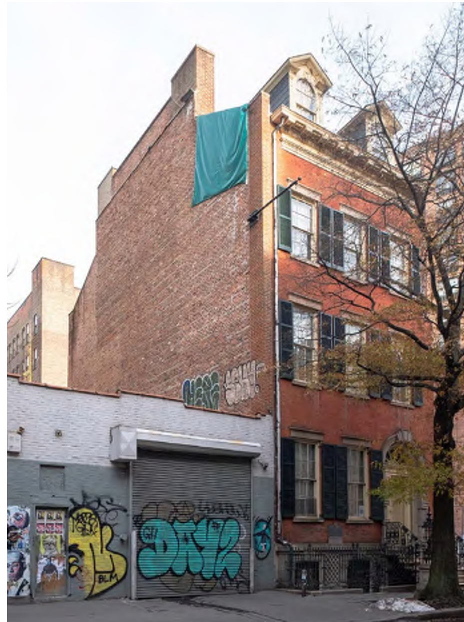
CURRENT LOT LINE WALL CONDITION
