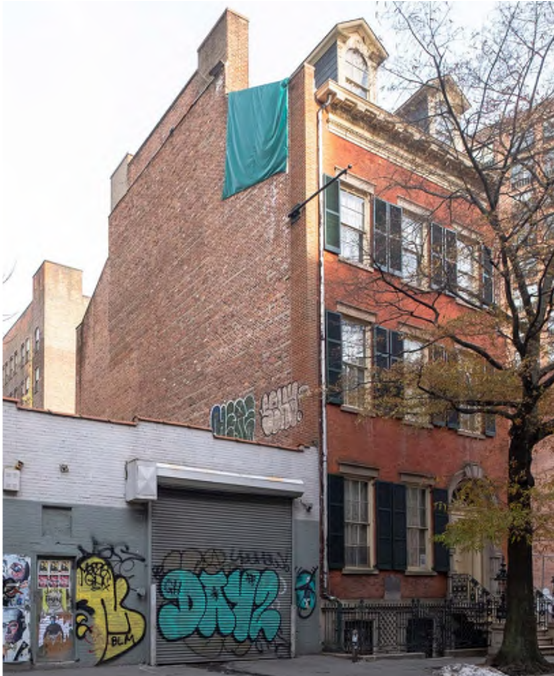
CURRENT LOT LINE WALL CONDITION
