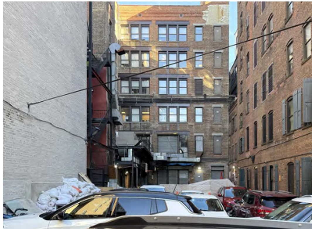
B. View looking North from 27 E. 4th Rear Facade.
