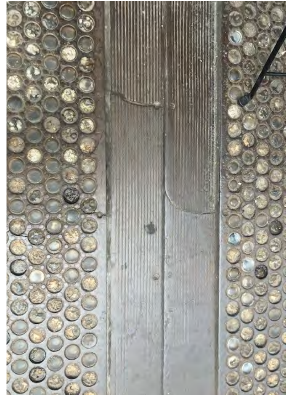
11 Damaged Frame and Glass Close-Ups Scale: NTS
