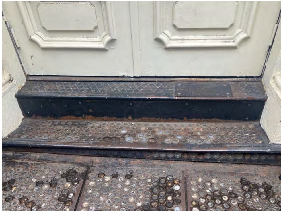
19 Broome Street Bullet Glass Step at Display Window Scale: NTS
