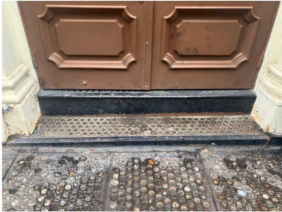
18 Broome St Bullet Glass Step at Egress Stair Scale: NTS
