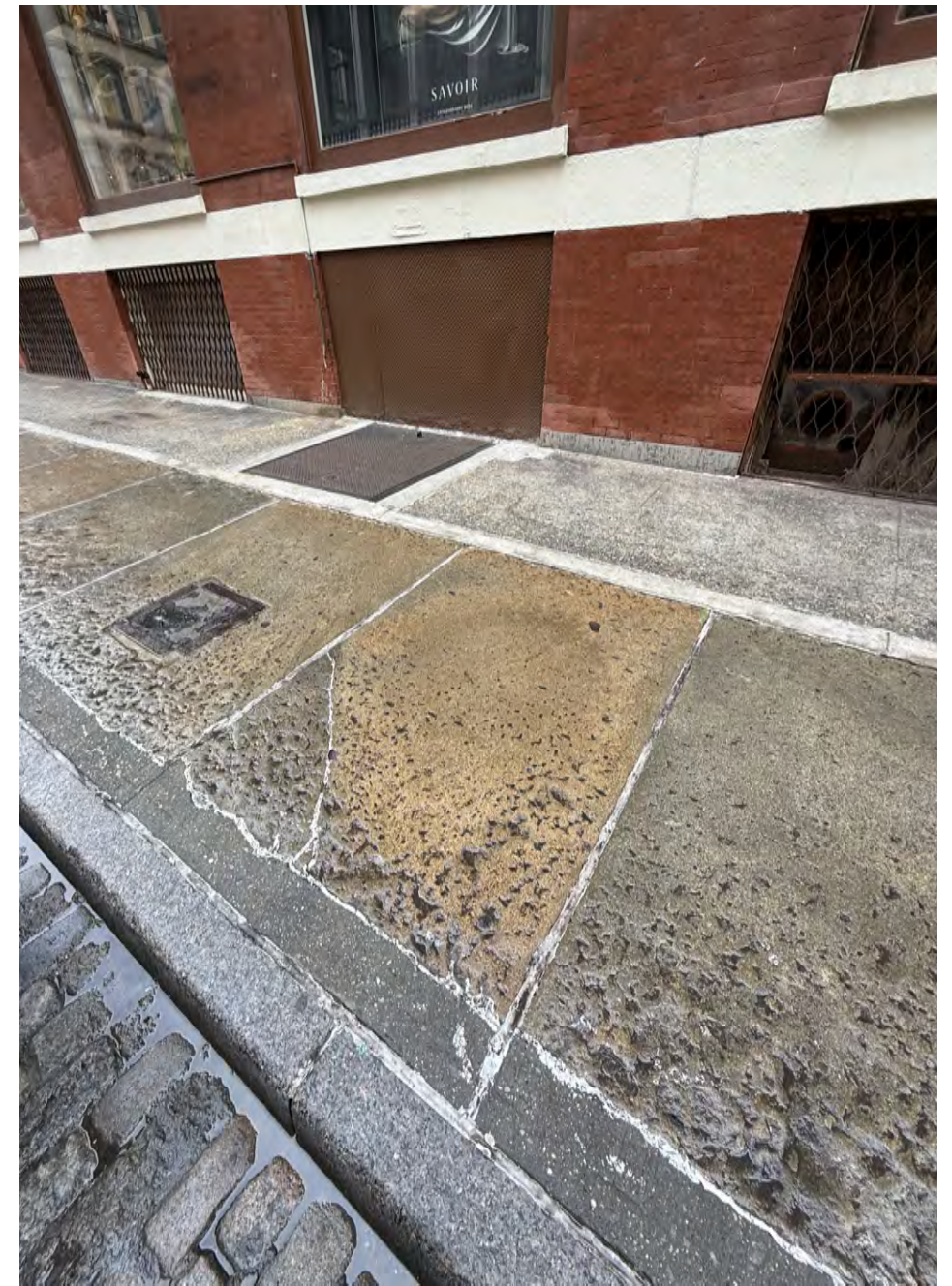
5 Concrete Sidewalk Greene St patched over the years Scale: NTS
