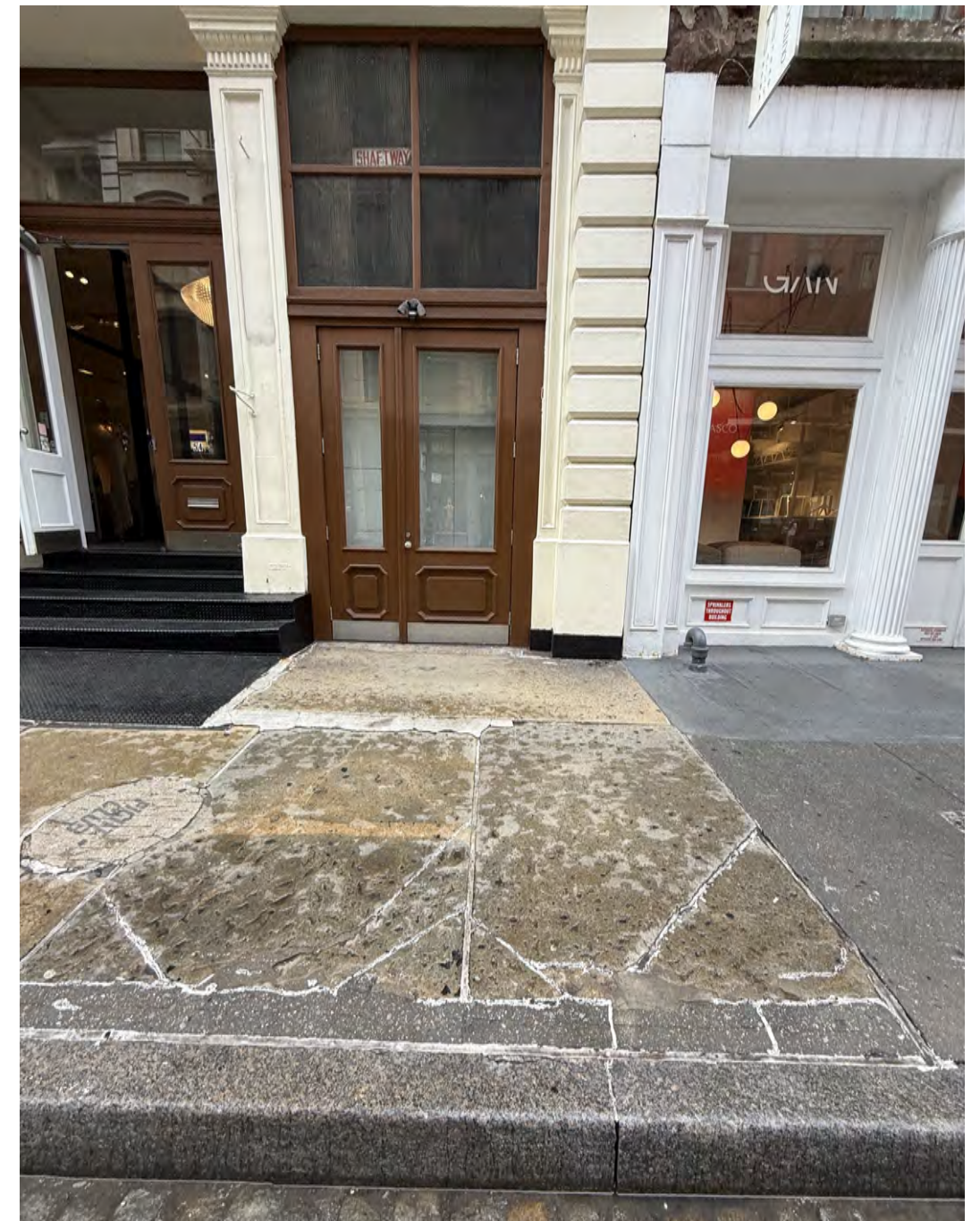
2 Elevator Entrance after 2019 Renovation by BKAA Scale: NTS
