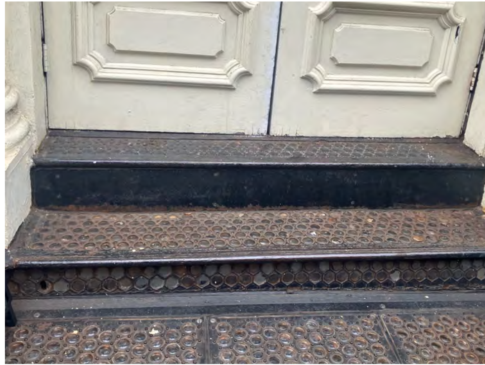
20 Broome Street Bullet Glass Step at Comm Entry Scale: NTS
