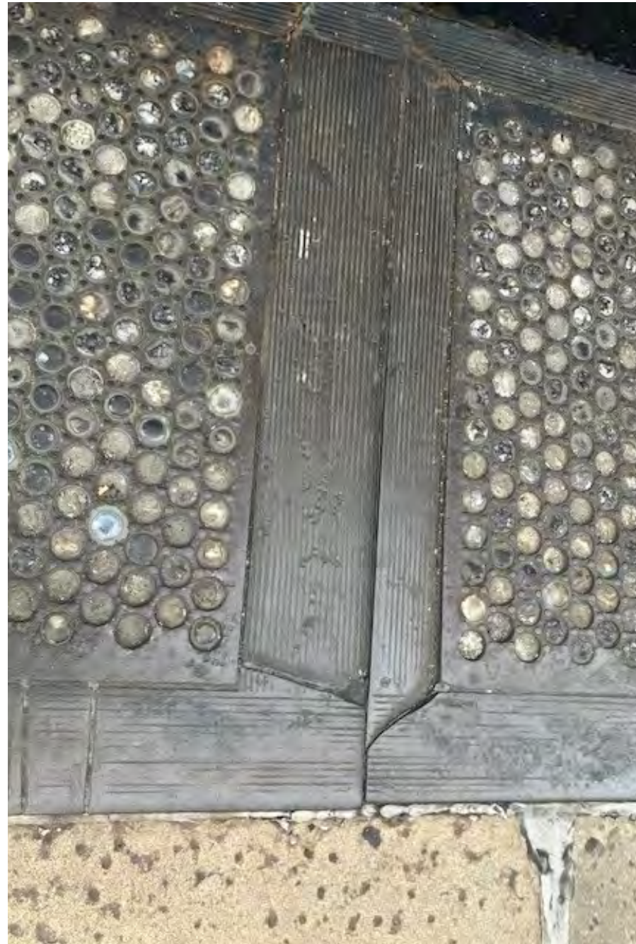
10 Damaged Frame and Glass Close-Ups Scale: NTS
