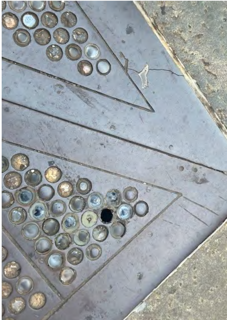
09 Damaged Frame and Glass Close-Ups Scale: NTS
