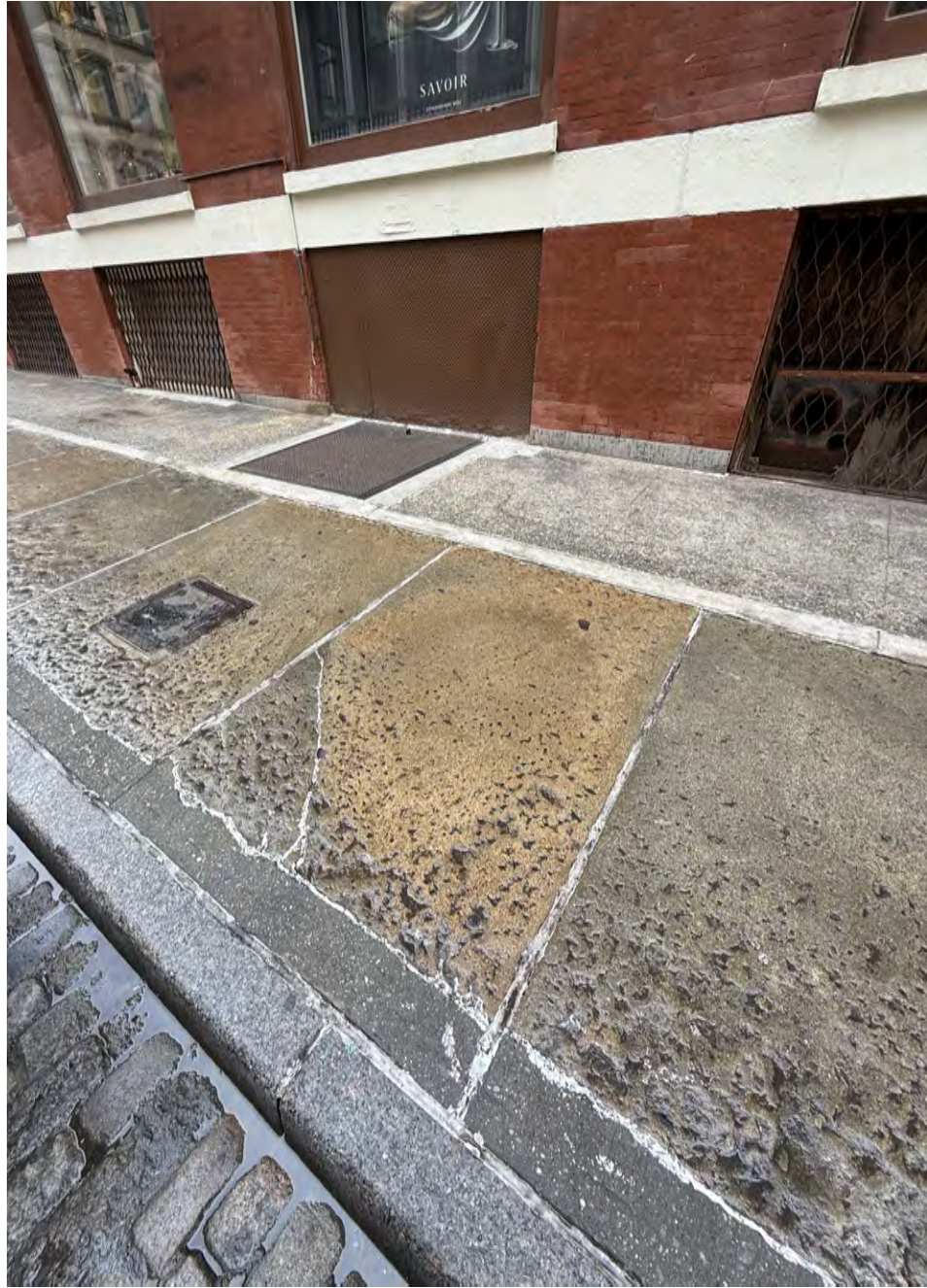
5 Concrete Sidewalk Greene St patched over the years Scale: NTS
