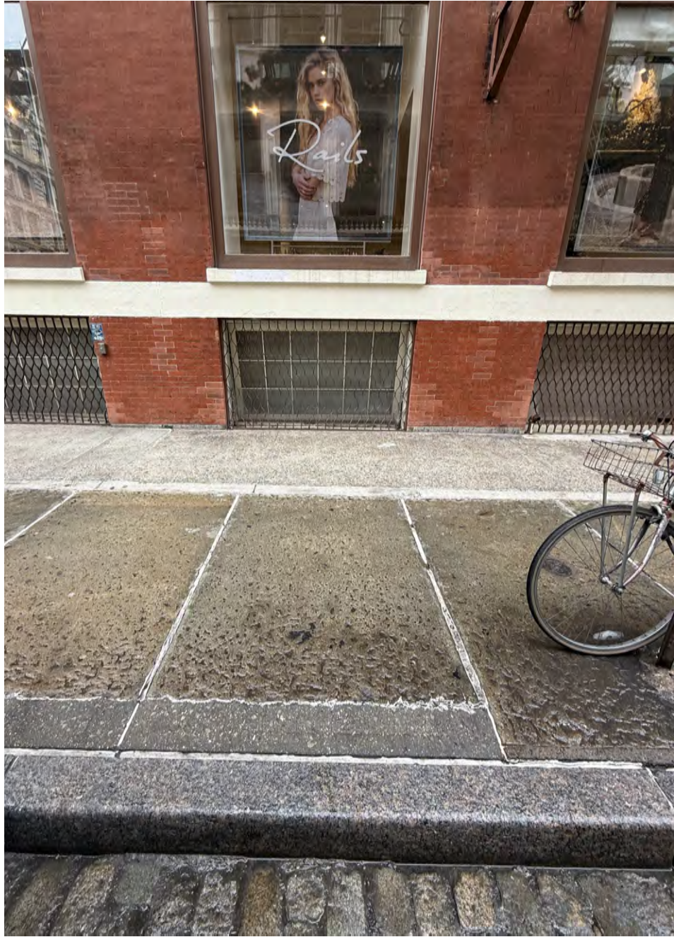
3 Granite Curb along Greene St Scale: NTS
