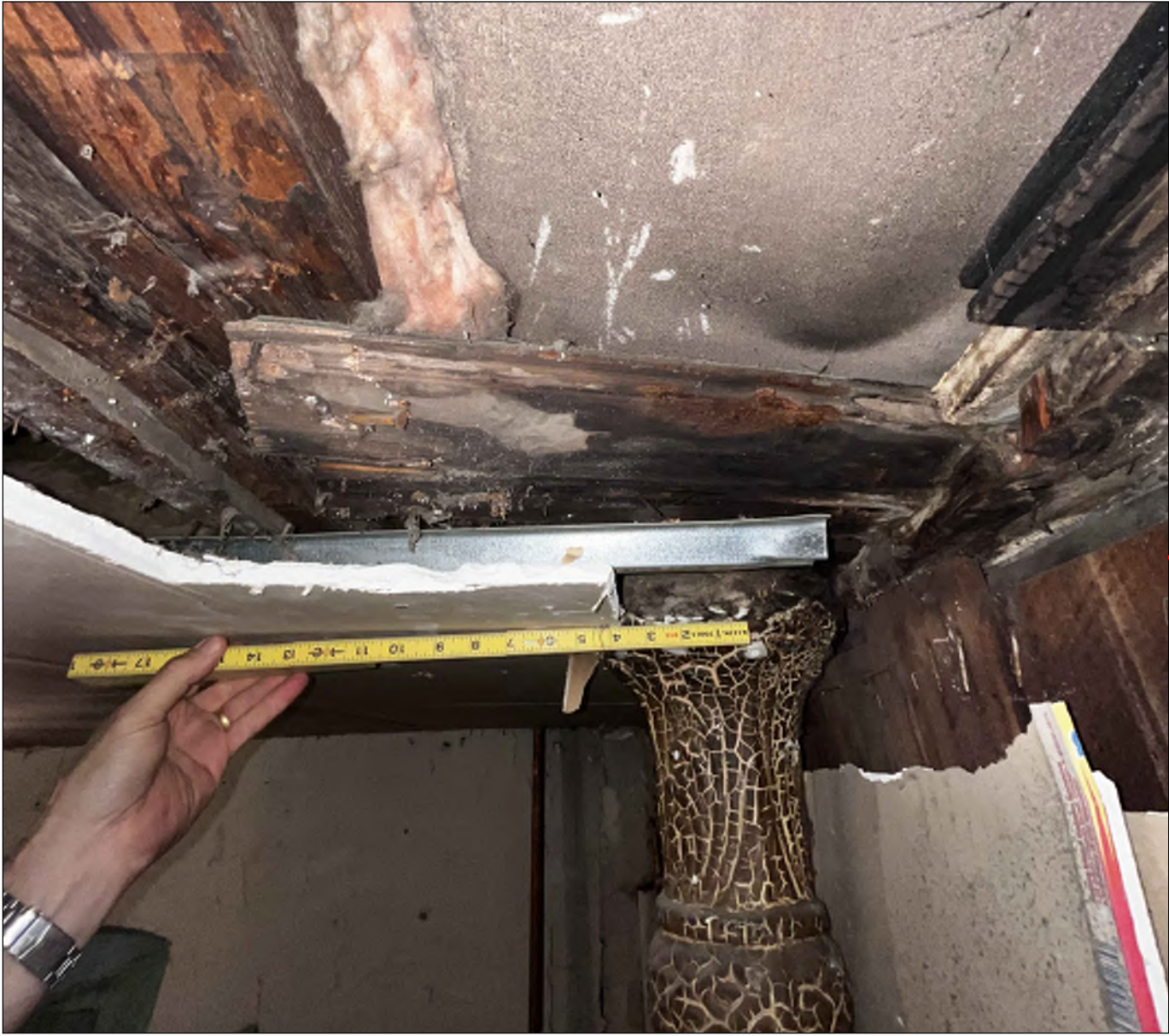
EXISTING CAST IRON COLUMNS SUPPORTING BROWNSTONE LINTEL BEHIND STUCCO FACADE
