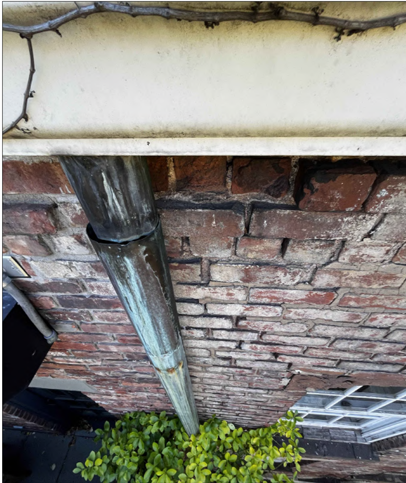
STEP CRACKS & OPEN JOINTS BELOW DOWNSPOUT LEADER
