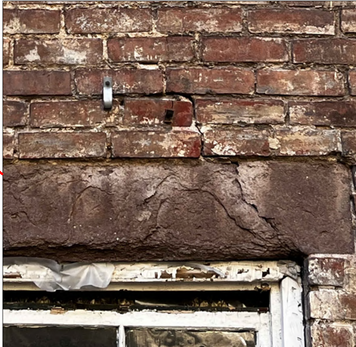
SPALLED AND ERODED BROWNSTONE LINTELS & SILLS
