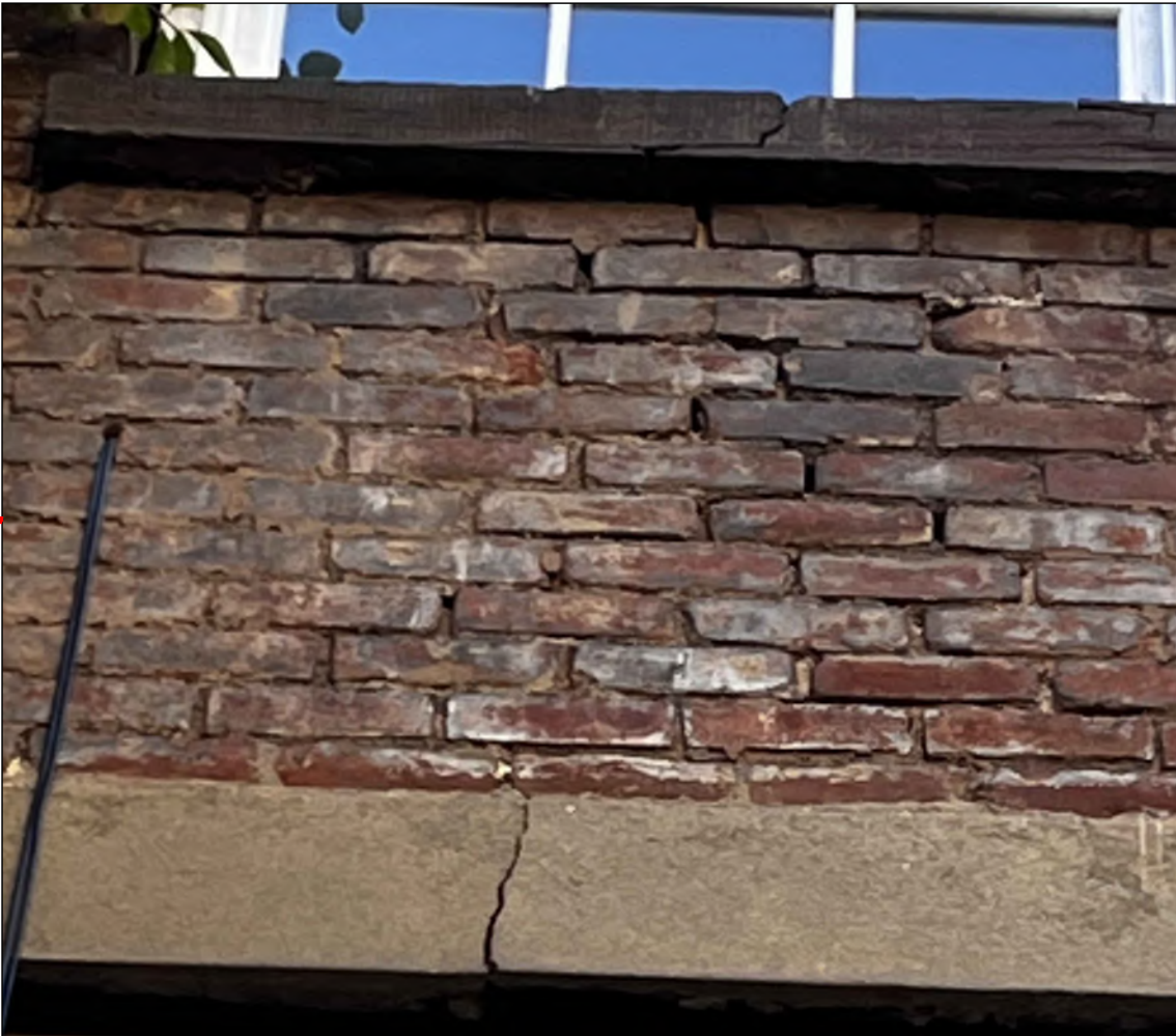
PARGED LINTEL CRACKED AT MID-SPAN CAUSING STEP CRACKING AT APRON WALL
