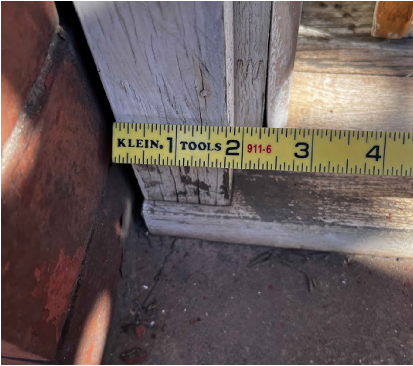
NON-ORIGINAL WINDOWS WITH NO BRICK MOULD OR CAULKING
