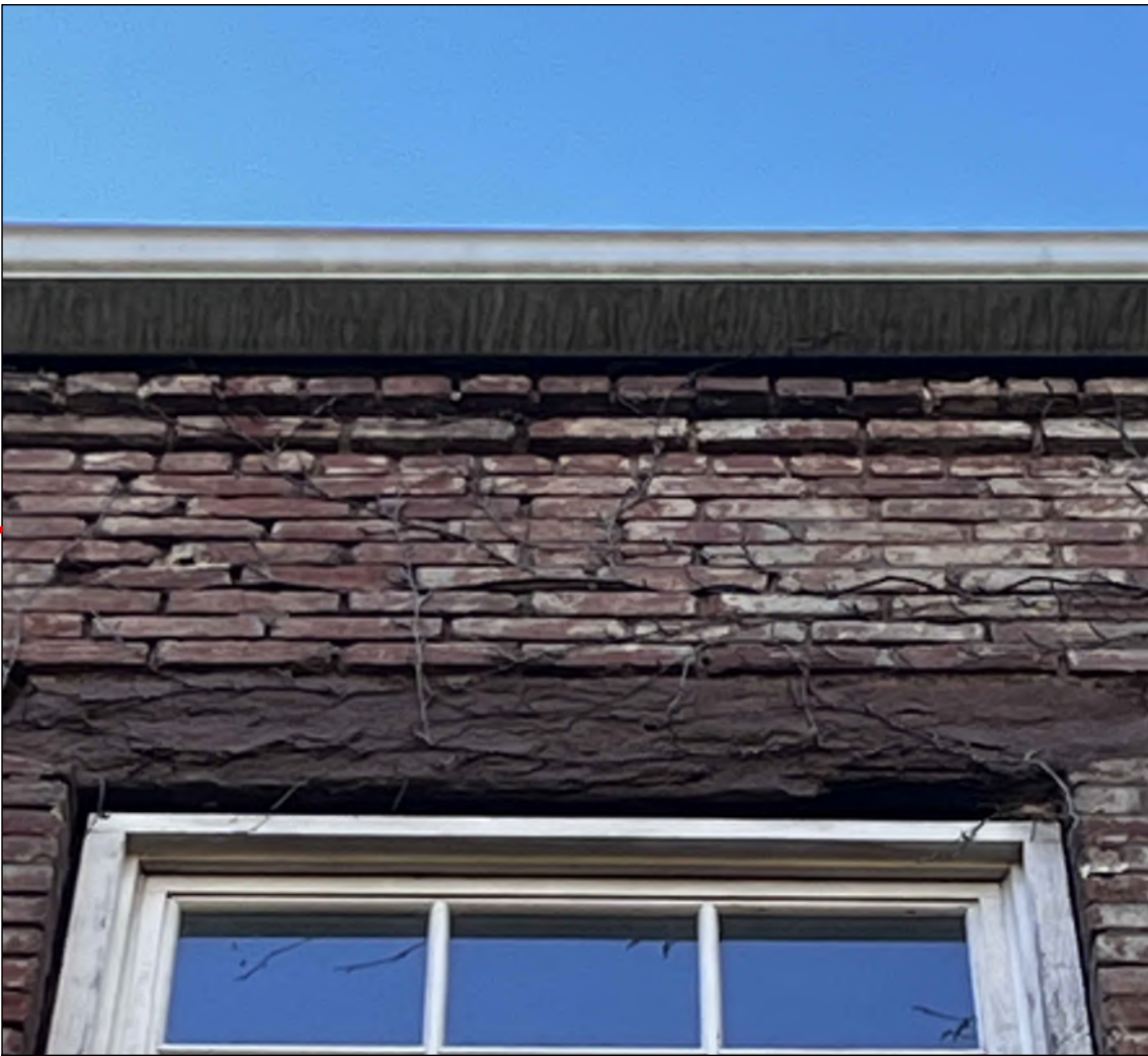
SPALLED BRICKS AND OPEN JOINTS BELOW EXISTING GUTTER
