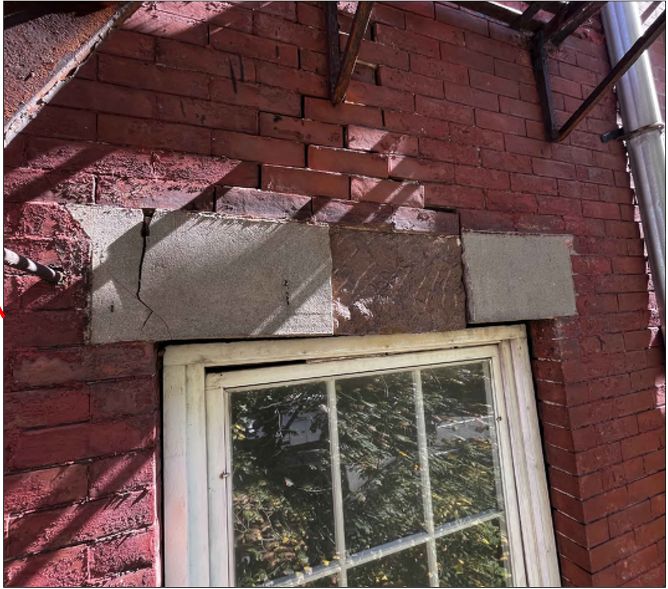
CRACKED BROWNSTONE LINTEL, DISPLACED BRICK, AND DELAMINATED PARGING
