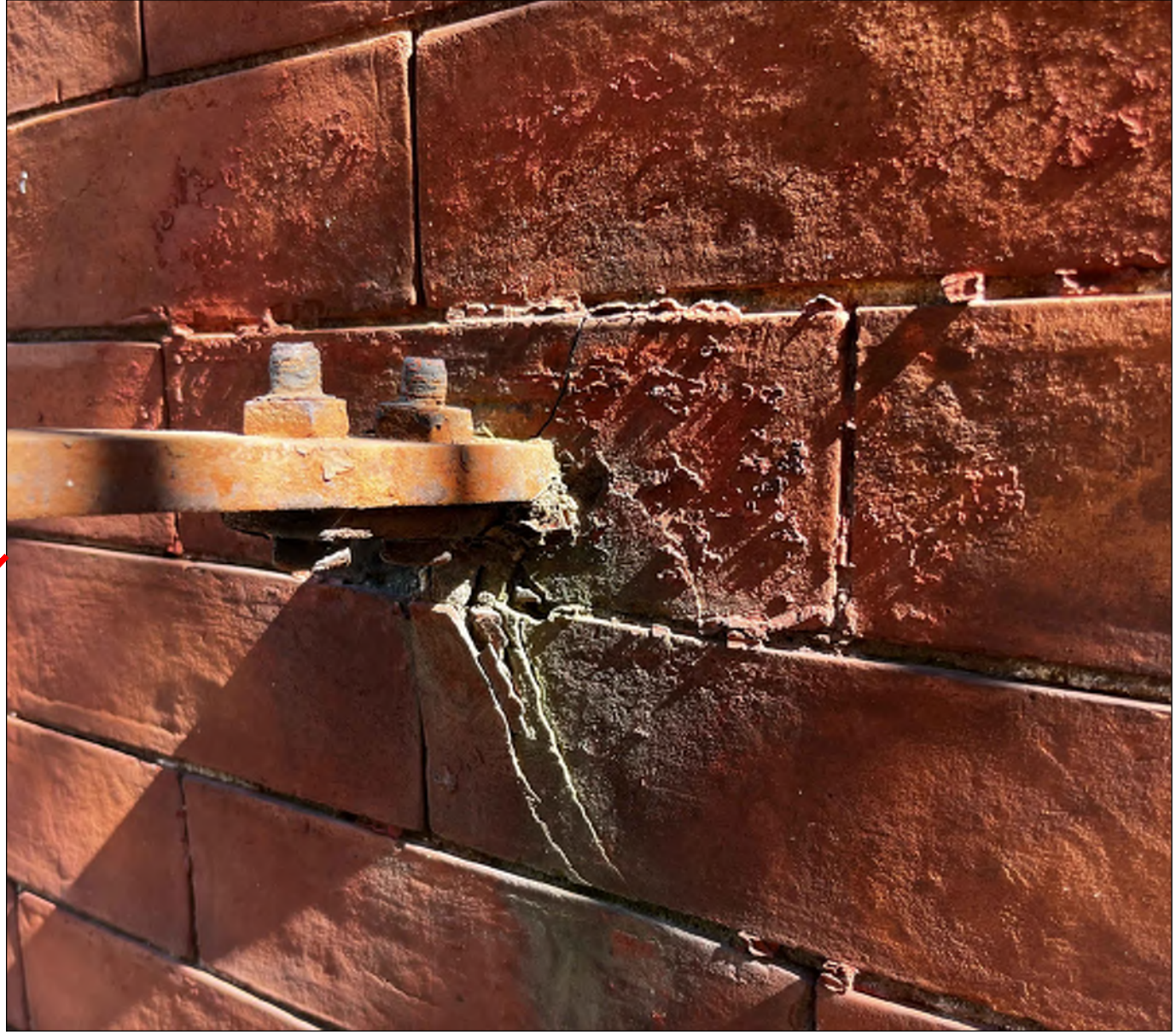
DAMAGED BRICK & RUSTING AT FIRE ESCAPE ATTACHMENT POINTS
