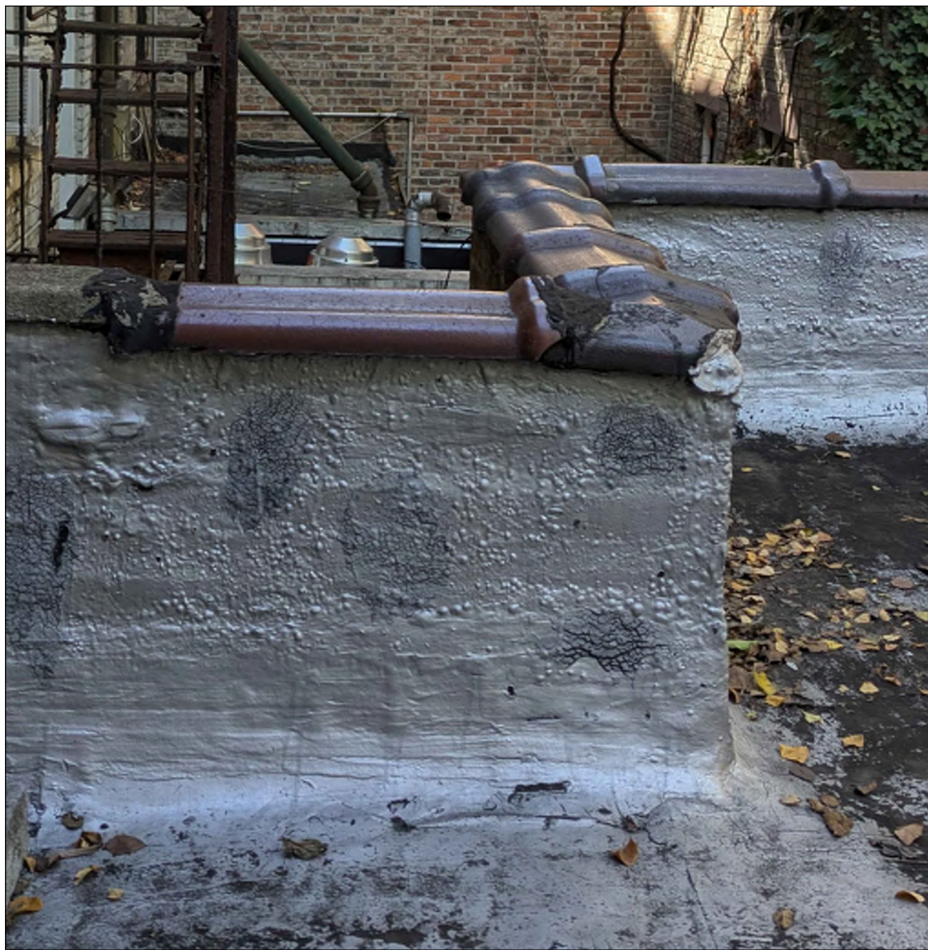
ROOFING & PARAPET IN POOR CONDITION
