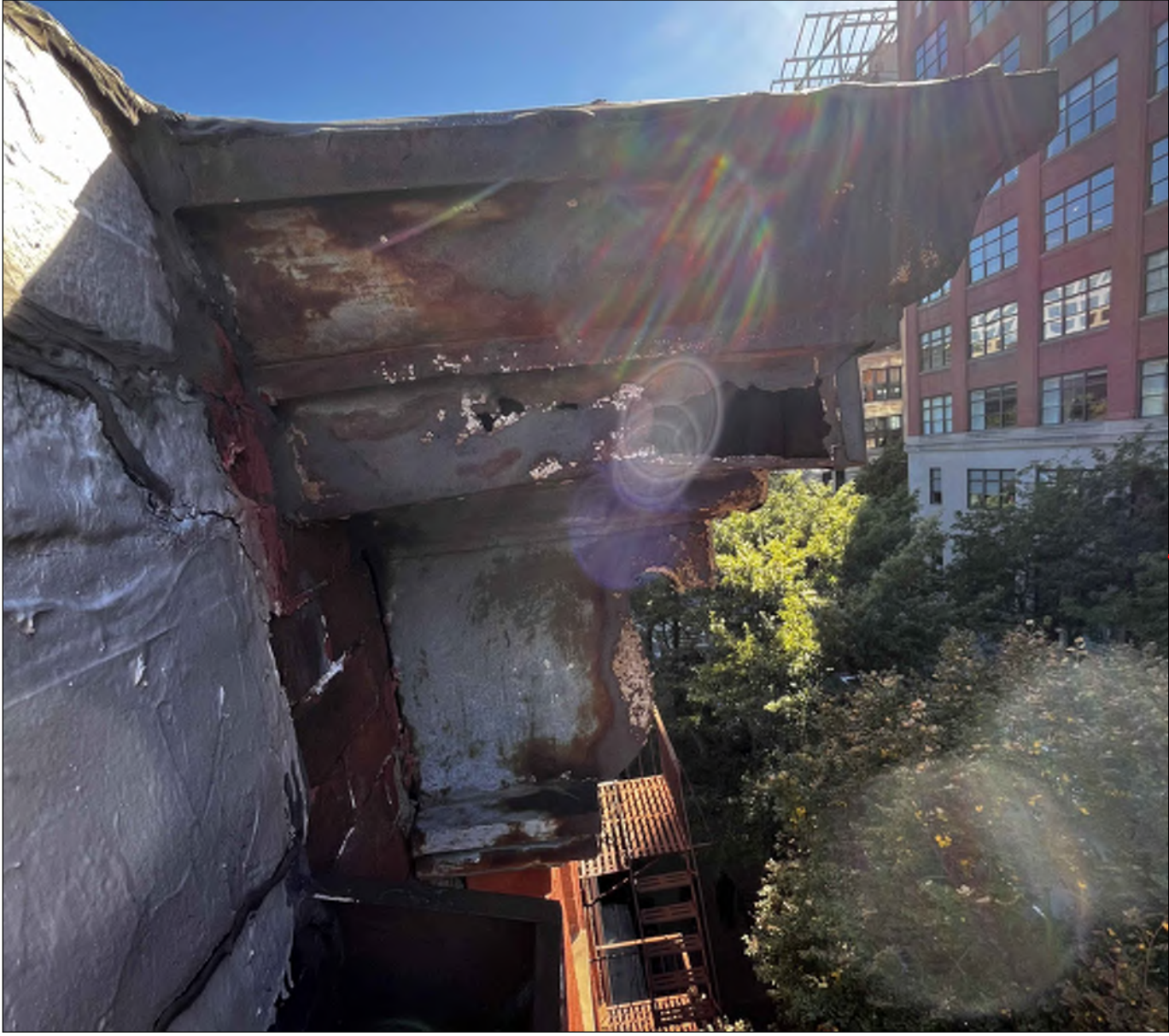
WIDESPREAD CORROSION & SECTION LOSS AT PAINTED GALVANIZED METAL CORNICE
