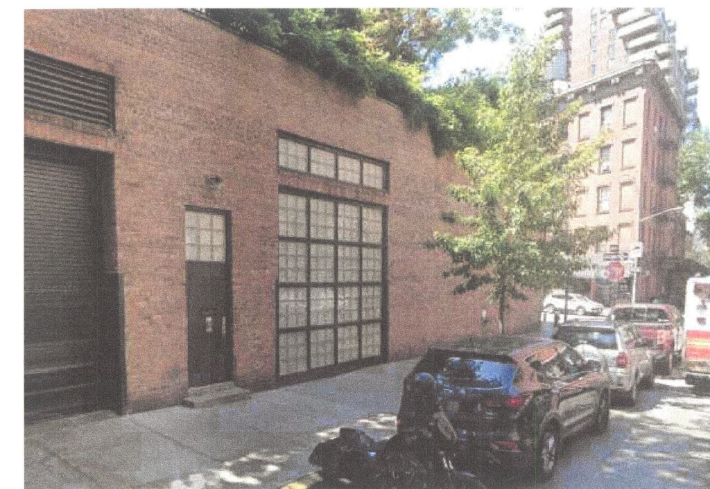
3 711 GREENWICH ST - FACADE FROM EAST
