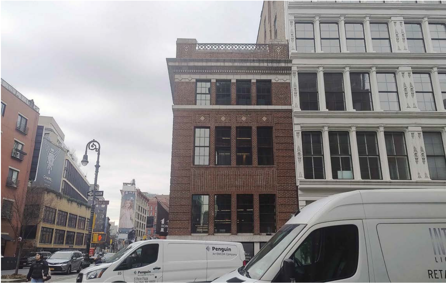
1. View from Bond St.
