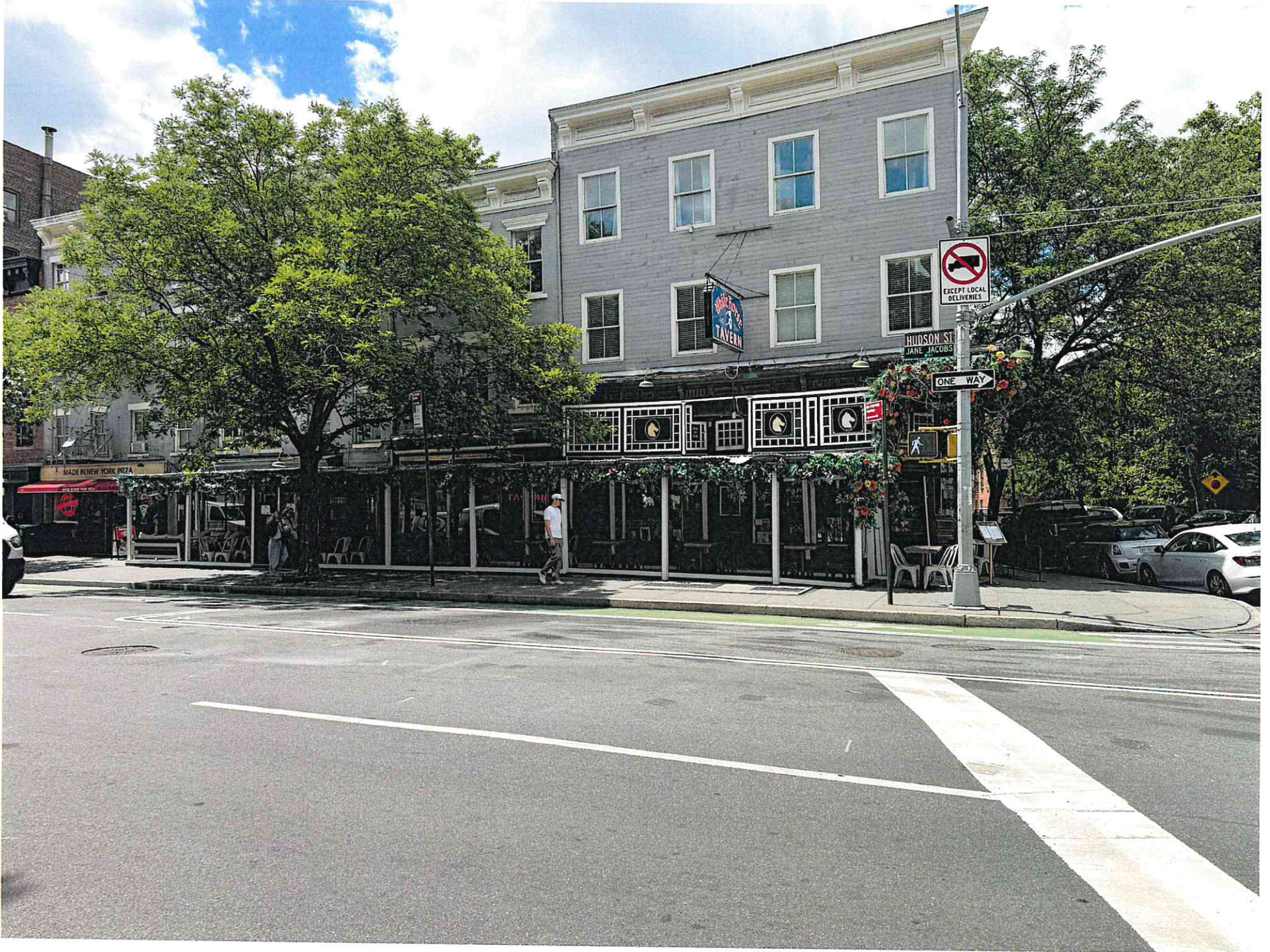
Photo from Summer 2024 - Enclosure has been deconstructed
