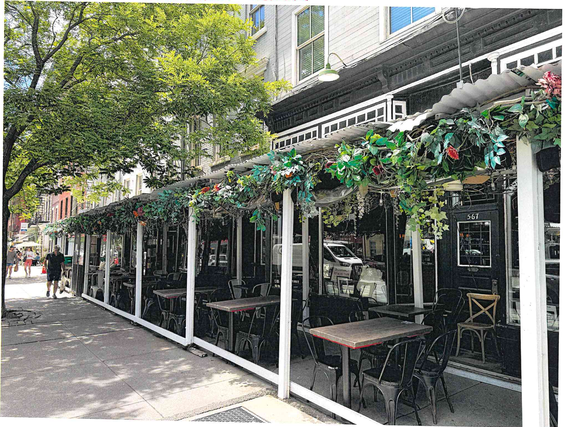
Photo from Summer 2024 - Enclosure has been deconstructed
