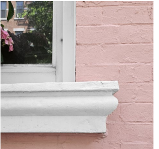
Existing detail to be restored
