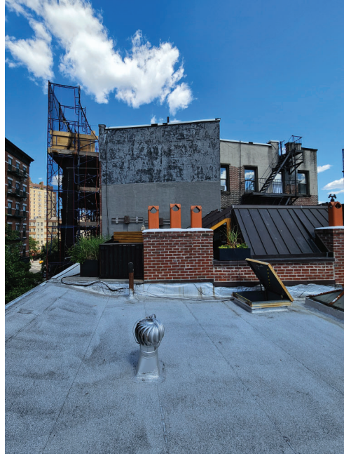
7 - East View from Roof
