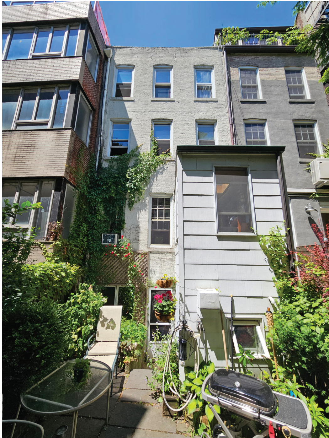
1 - North View at Rear Yard
