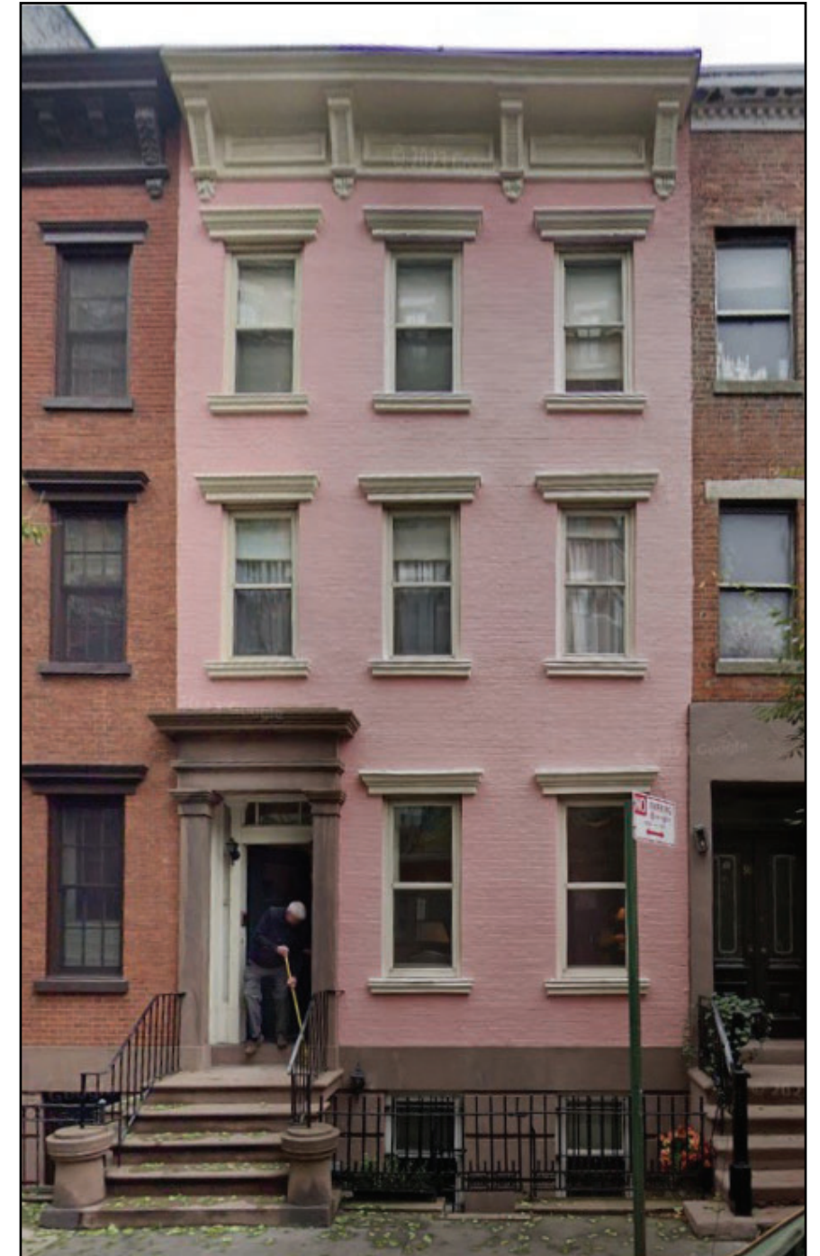
Existing North Facade Photo taken on 2024/02/28
