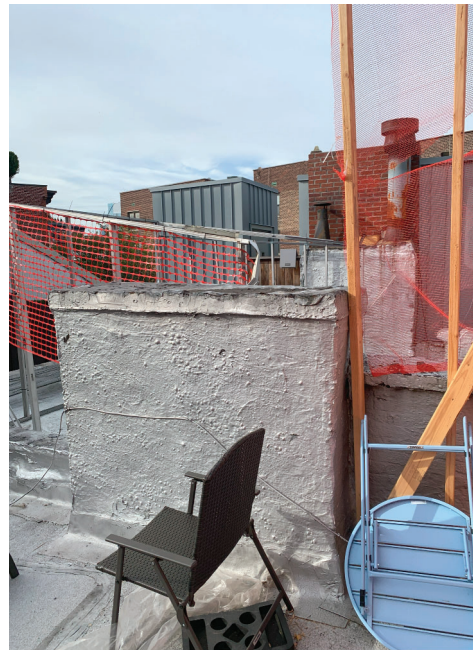
6 - West View from Roof
