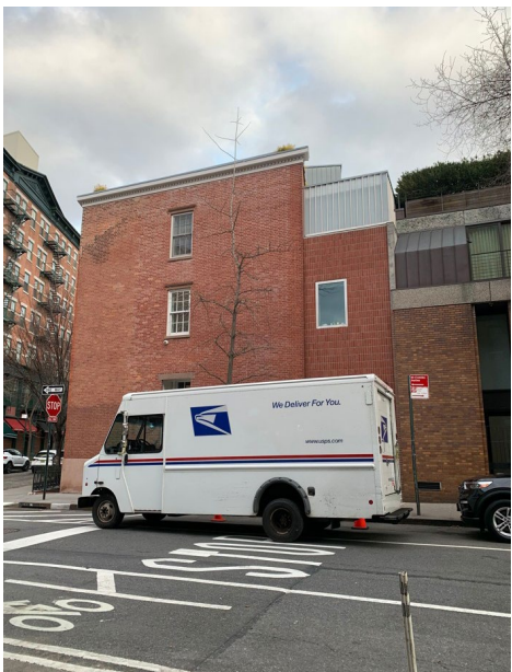
View from Greenwich St South of Bank St Intersection
