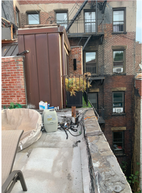
5 - East View from Roof
