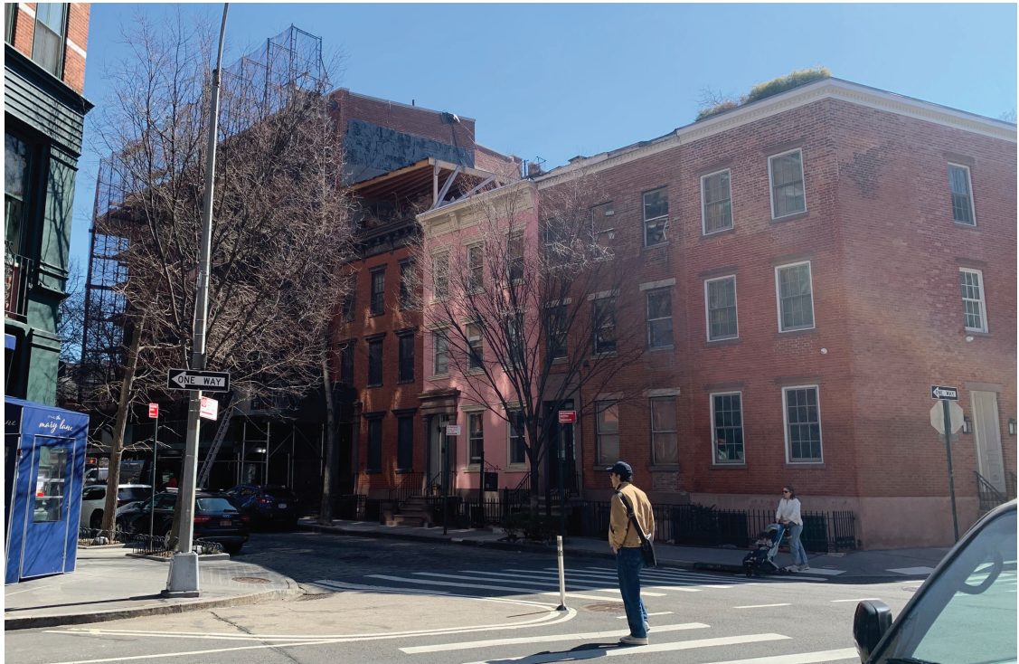
5 - View from Greenwich St (2025/03/11)
