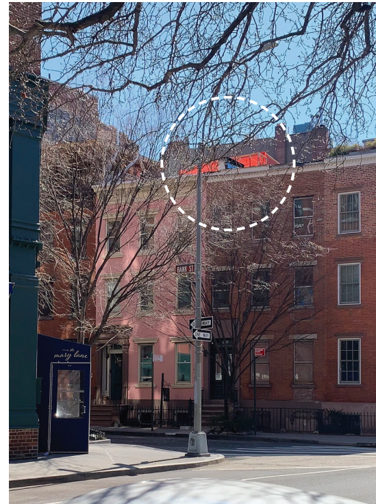
4 - View from Greenwich St (2025/03/11)
