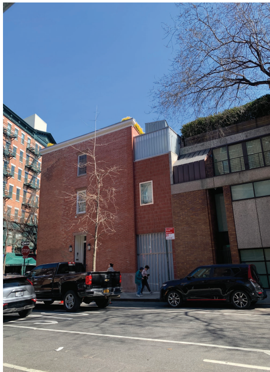
9 - View from Greenwich St (2025/03/11)
