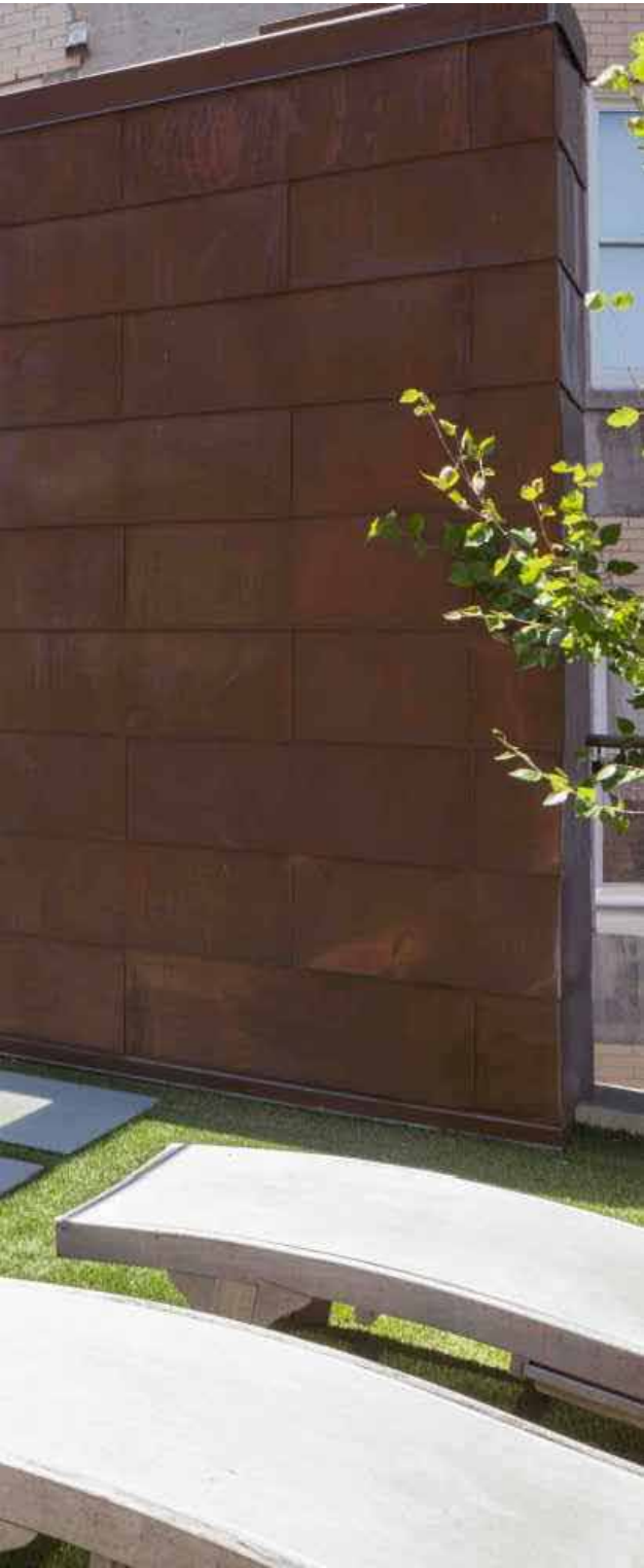
3 MATERIAL: COPPER PANEL CLADDING NTS
