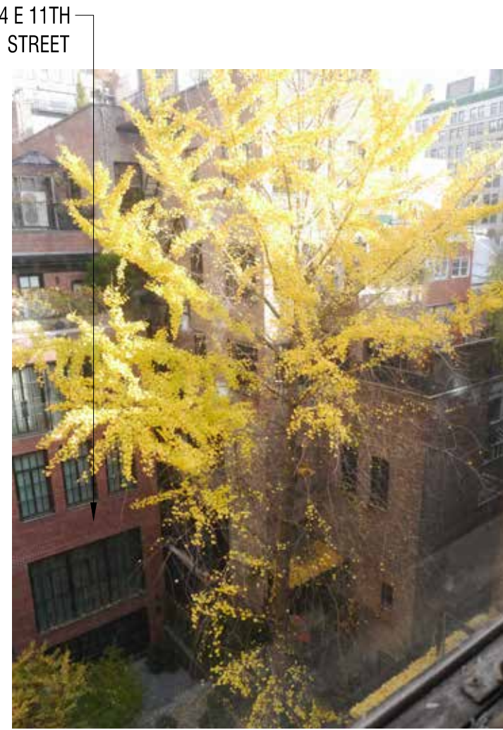
4 SITE PHOTOS: ACROSS, 14 E 11TH STREET REAR FACADE NTS
