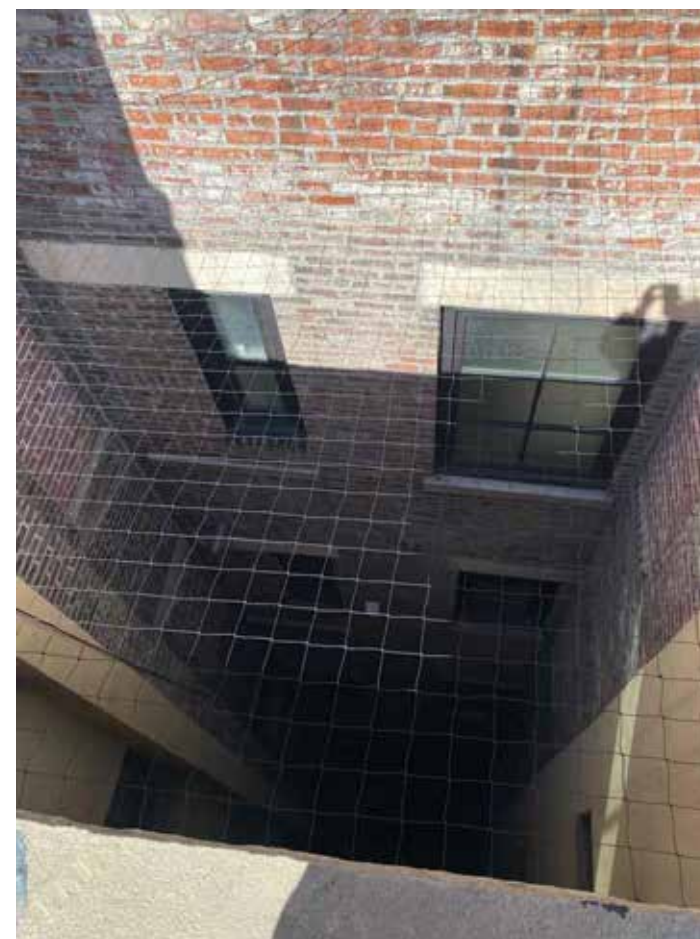
2 SITE PHOTOS: EXISTING LIGHTWELL SHARED WITH 3 E 10TH STREET NTS
