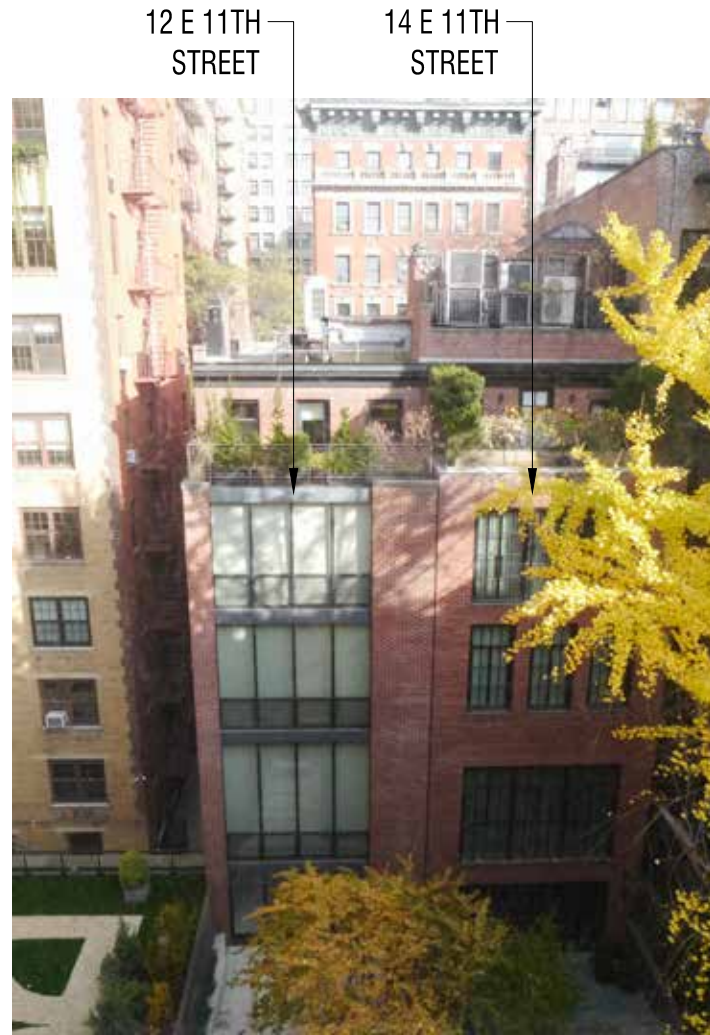
3 SITE PHOTOS: ACROSS, 12 E 11TH STREET REAR FACADE NTS
