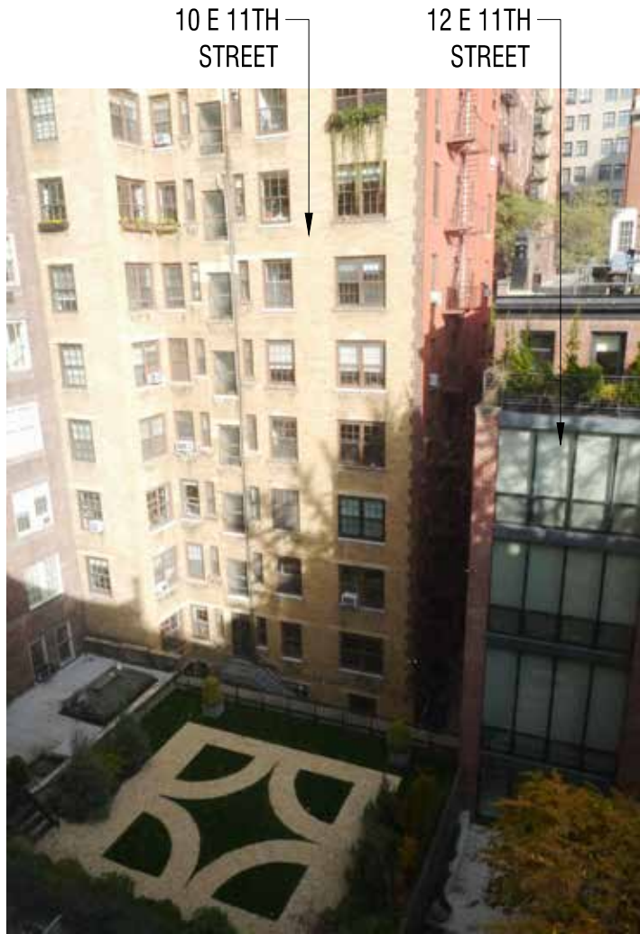
2 SITE PHOTOS: ACROSS, 10 E 11TH STREET REAR FACADE NTS
