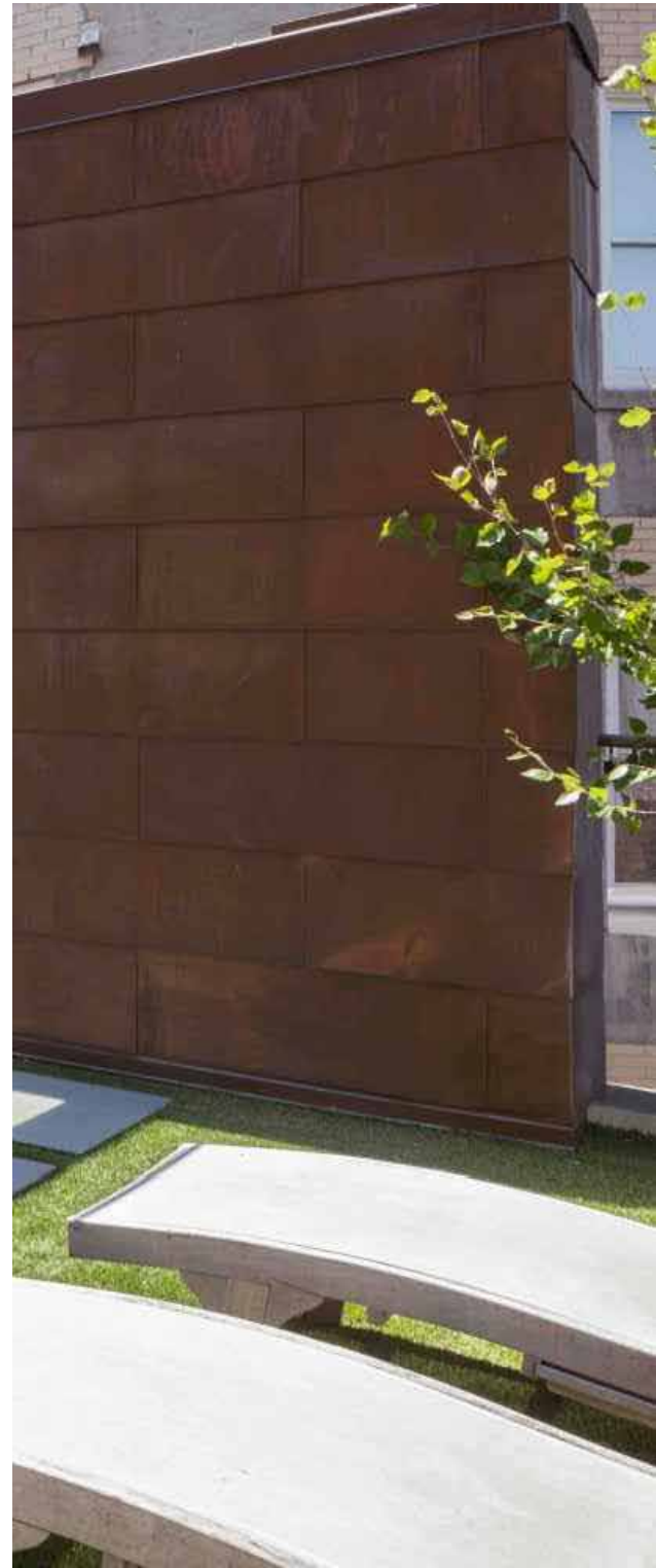
3 MATERIAL: COPPER PANEL CLADDING NTS
