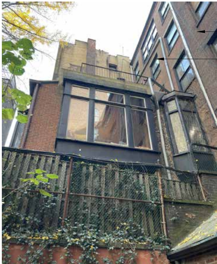
5 SITE PHOTOS: ADJACENT, 7 E 10TH STREET REAR FACADE NTS
