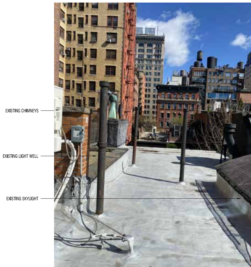
2 SITE PHOTOS: EXISTING ROOF VIEWING NORTH NTS
