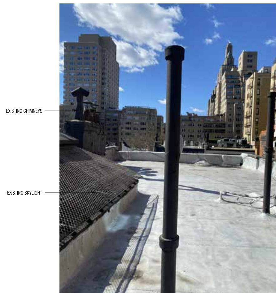
1 SITE PHOTOS: EXISTING ROOF VIEWING SOUTH NTS
