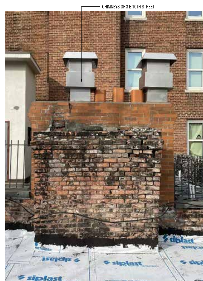
1 SITE PHOTOS: EXISTING ABANDONED CHIMNEY BY THE WEST SIDE NTS
