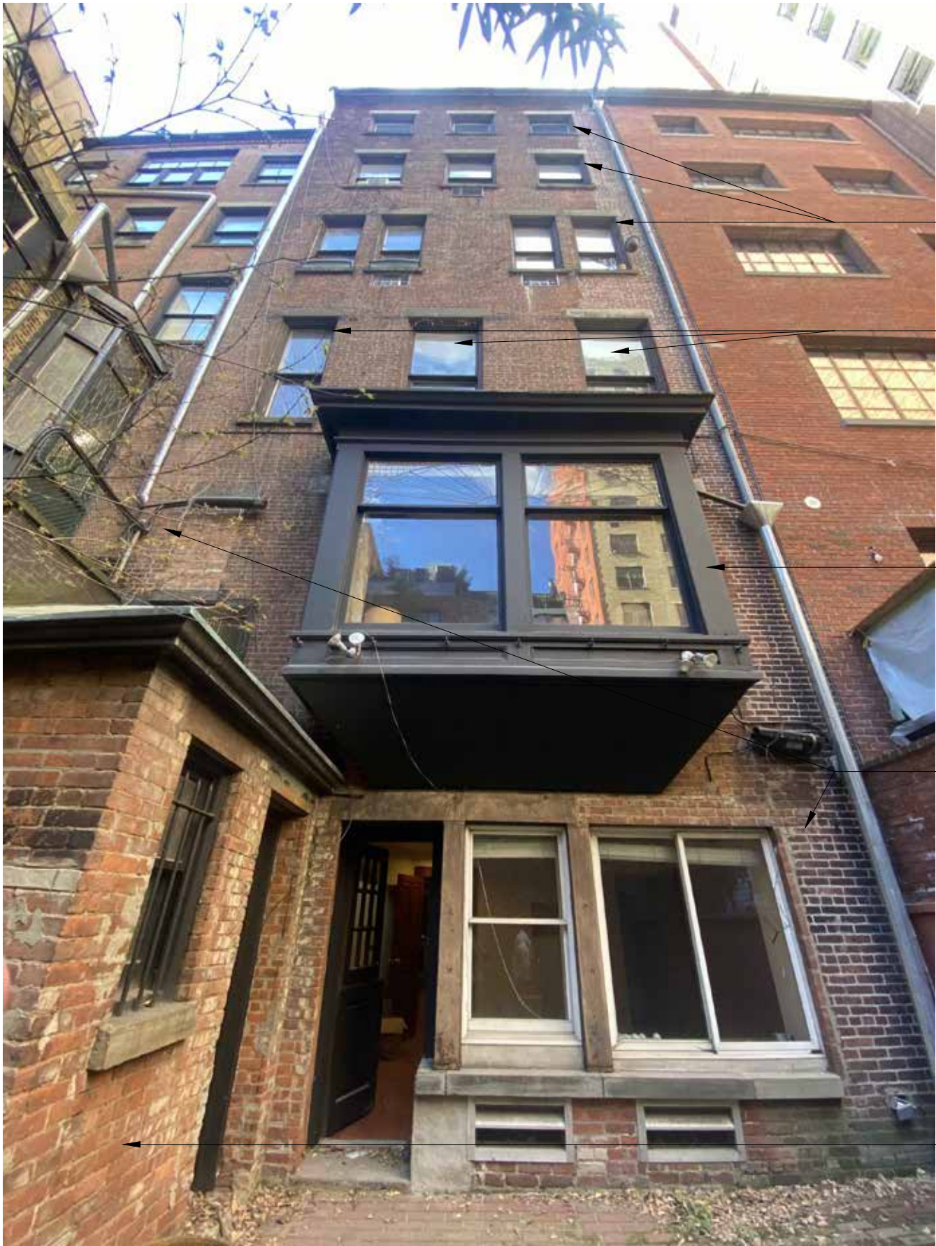
1 SITE PHOTO: EXISTING REAR FACADE (NORTH ELEVATION) NTS
