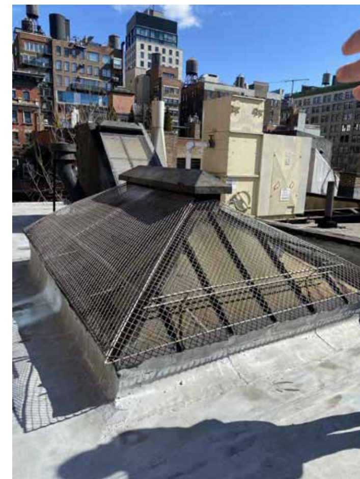
2 SITE PHOTOS: EXISTING SKYLIGHT
