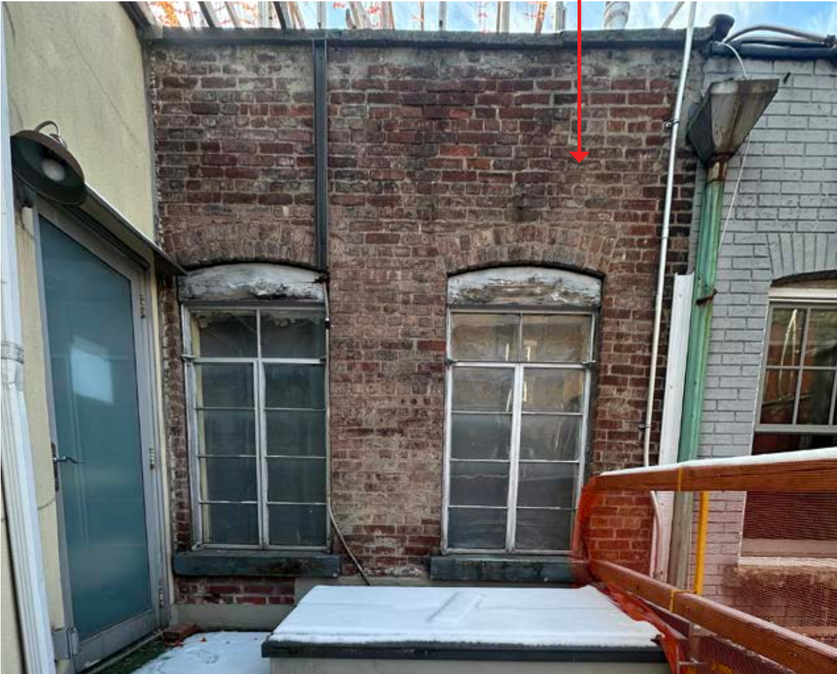
EAST ELEVATION MASONRY WALL
