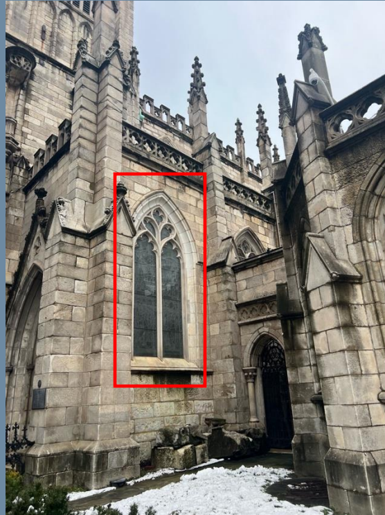
Limestone replacement units at stone tracery.
