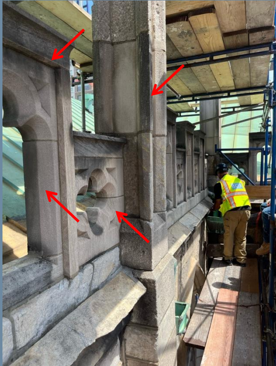
Limestone replacement units at pinnacle and balustrade.
