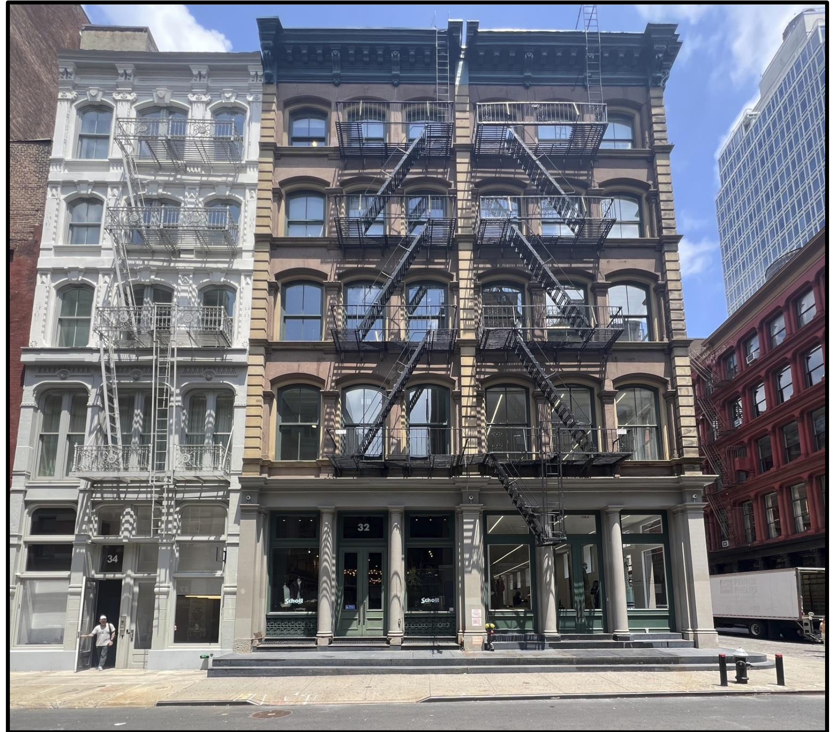
Current Primary Façade (2024)
