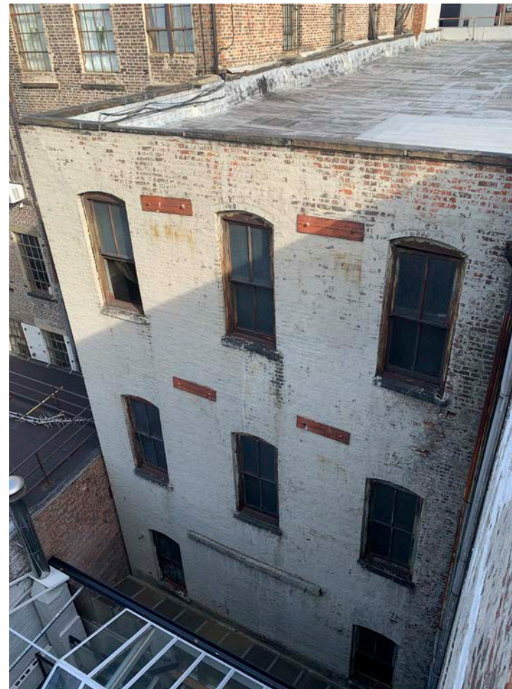
2. Rear Facade looking North-West
