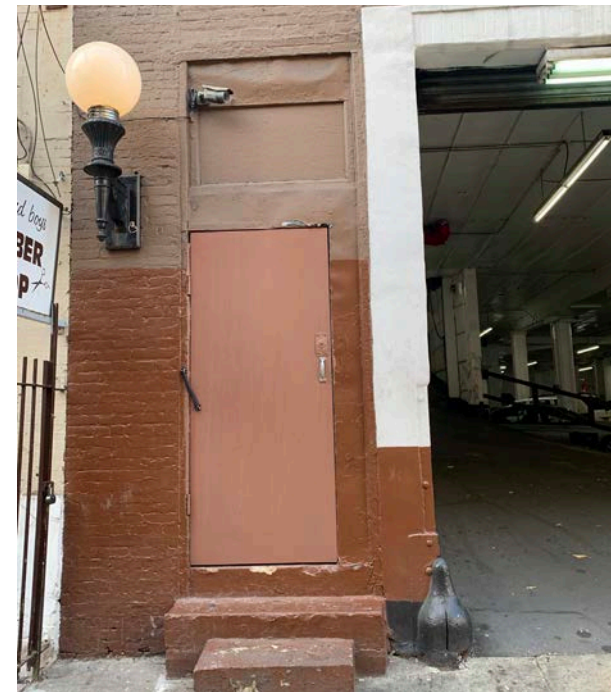
Entry Door, Stairs and Cast-Iron Globe Bracket Lamp
