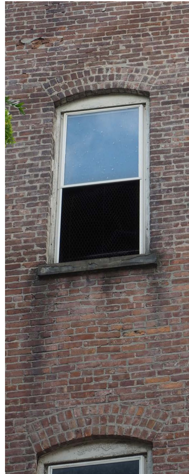
1/1 Double Hung Aluminum Window with Segmental Brick Arch Lintel, Masonry Sill
