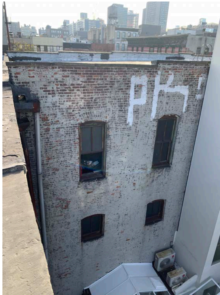
1. Rear Facade looking South-East
