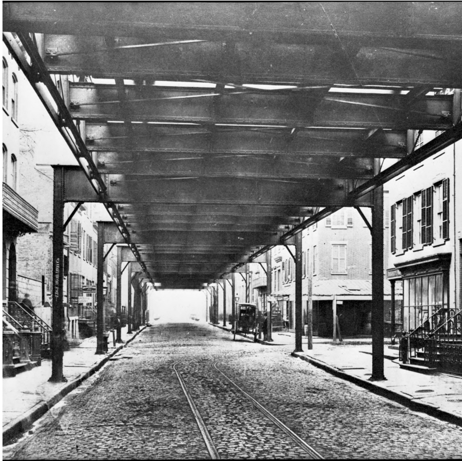
West 3rd Street under the Sixth Avenue El, c. 1878 (NYHS)
