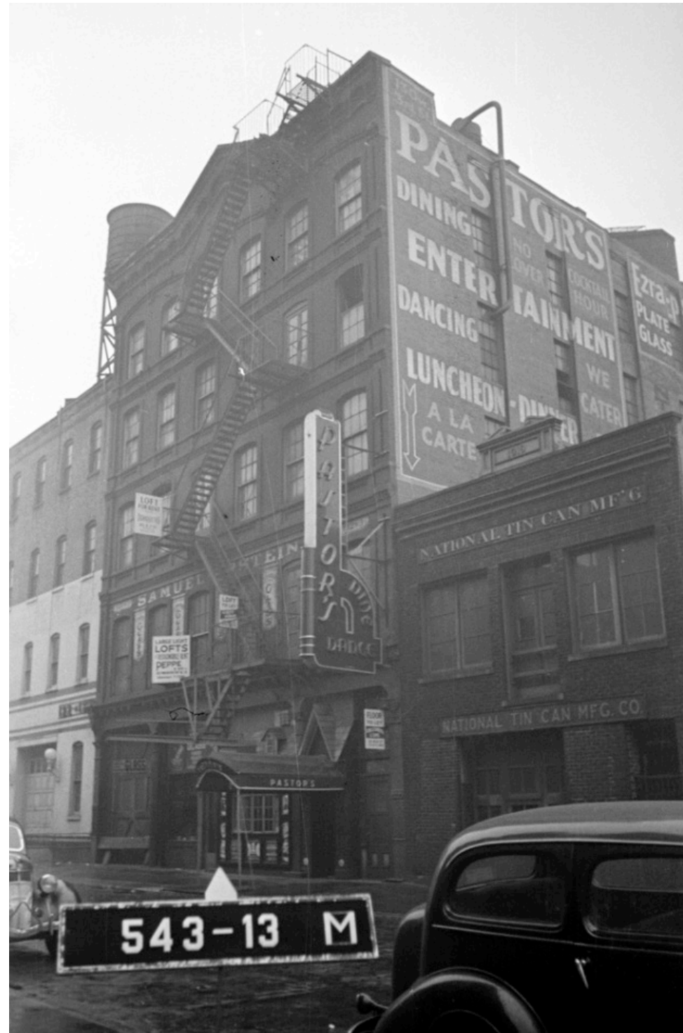
1940 (Muni) Repair Shop, 1874-75 Commercial conversion, 1940s
