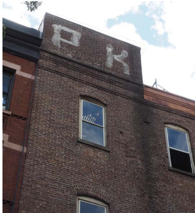
Northeastern Bulkhead, Windows, and Corbelled Cornice
