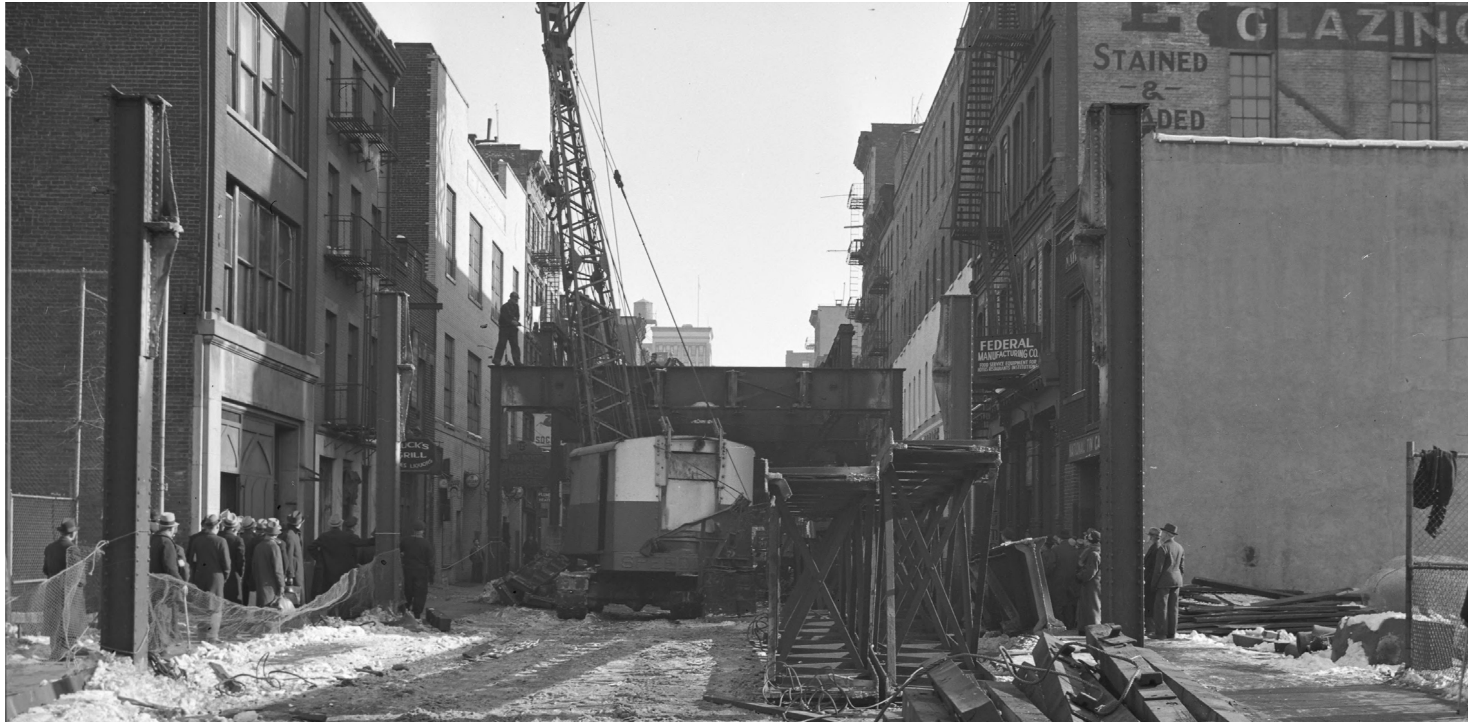
Dismantling of the Sixth Avenue El on West 3rd Street, 1939 (NYHS)
