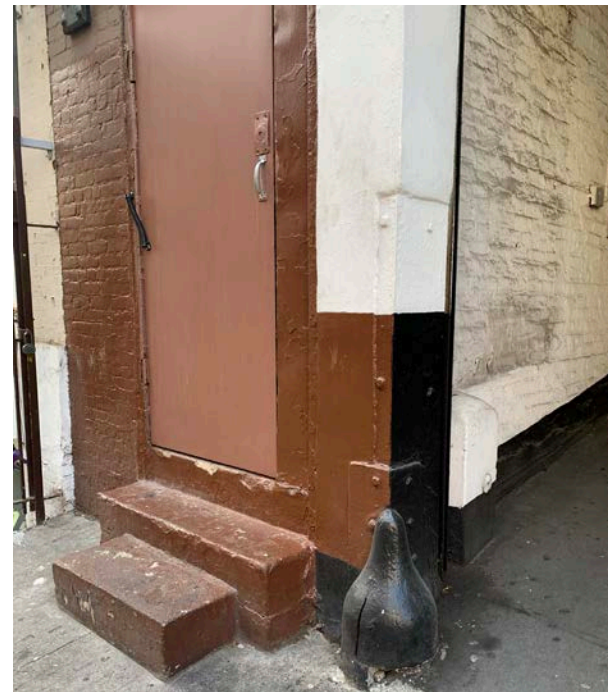
Garage Entry Bumpers, Stairs and Entry Door
