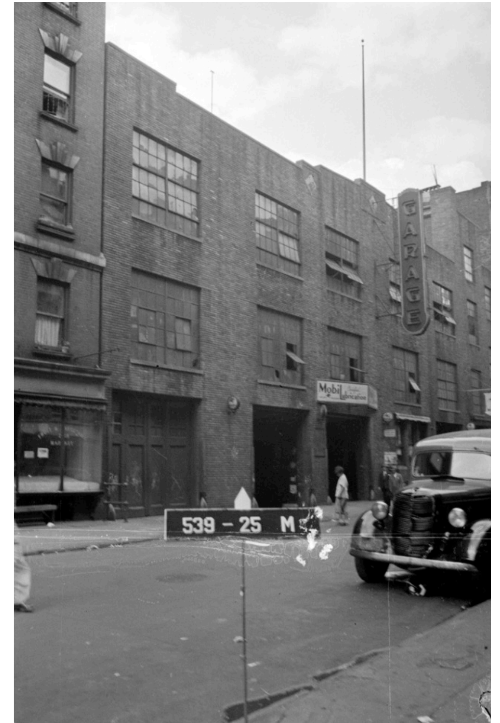
221 Thompson St Garage, 1919-20
