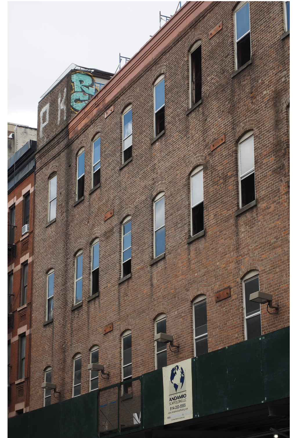
Second, Third, and Fourth Stories, Looking Southeast
