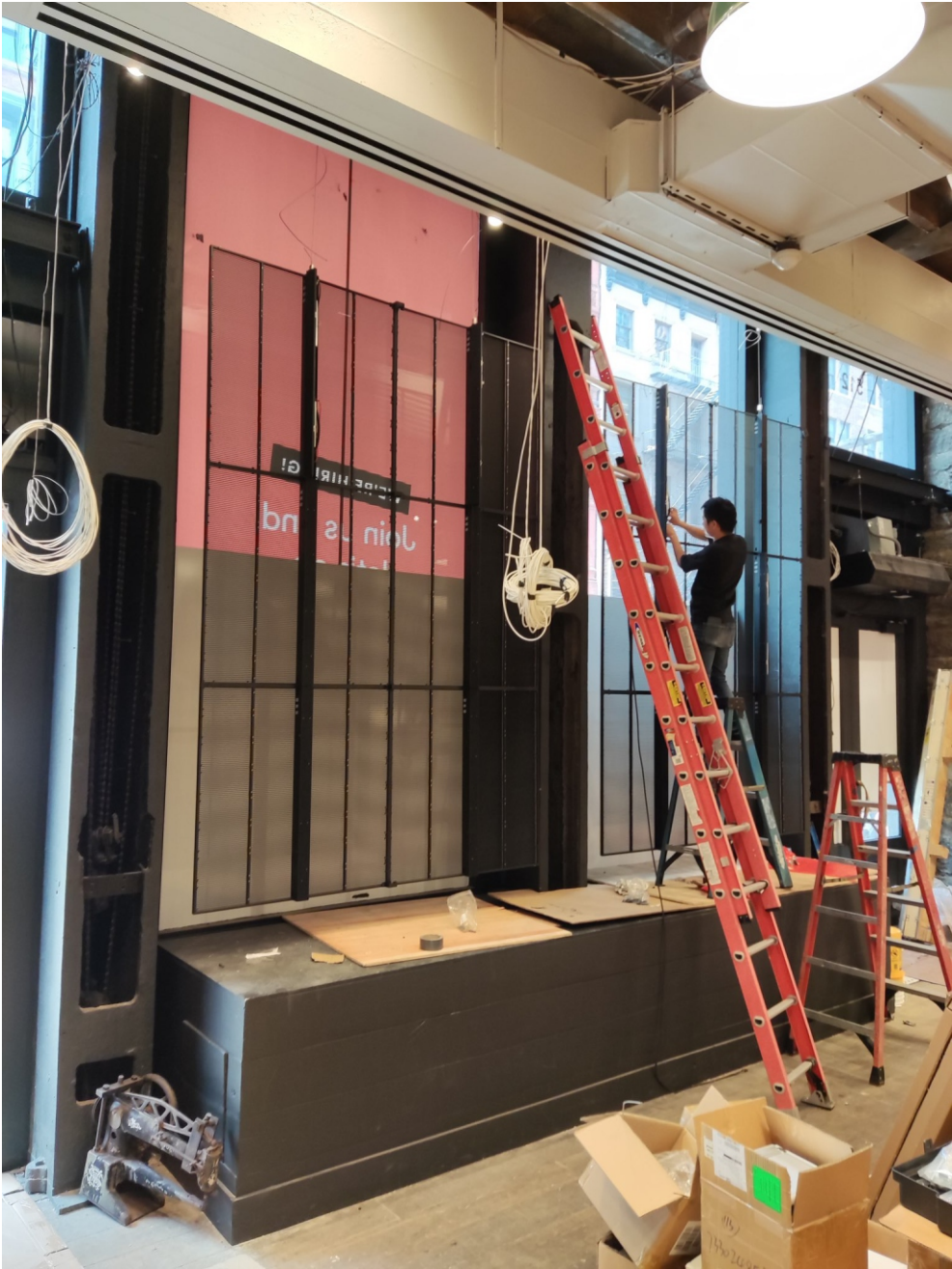
INSTALLATION PICTURE LED DISPLAY SIGN INSTALLED 8/15/2023
