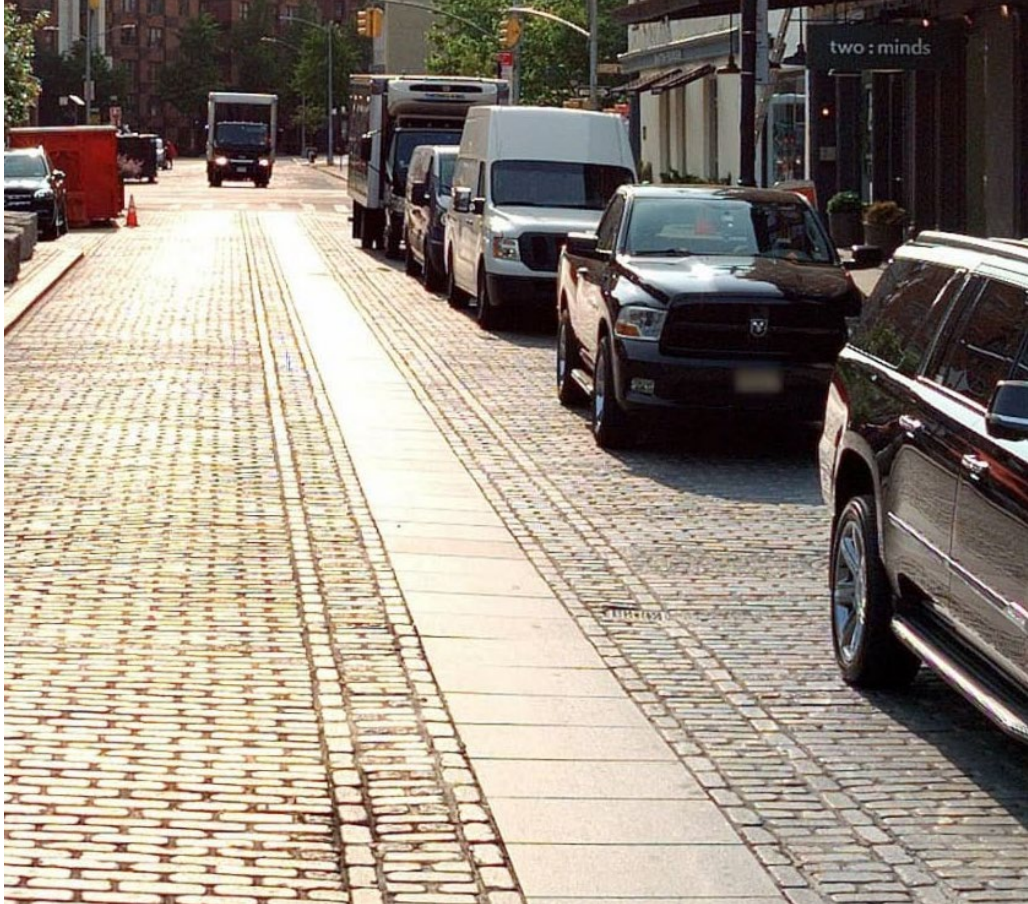
Completed granite bike lane on Gansevoort Street
