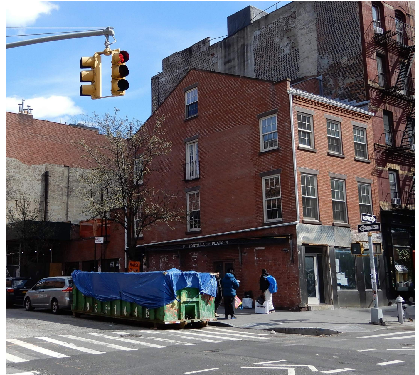
Mock-Up View from North West Corner of Washington Street and W 12th Street
