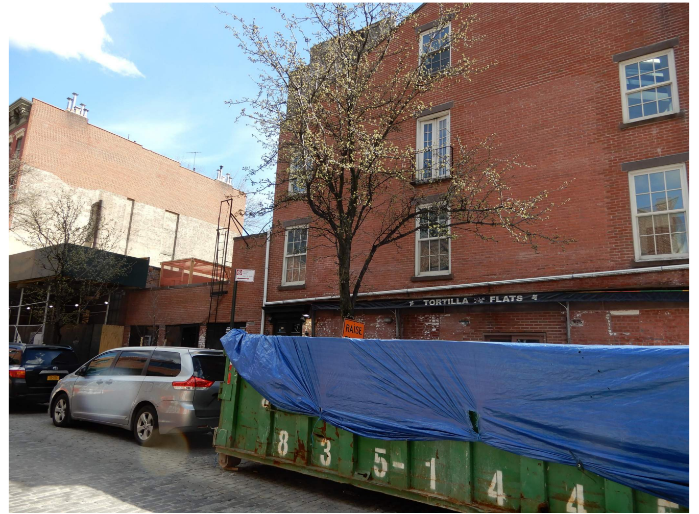
Mock-Up View from North East Corner of Washington Street and W 12th Street
