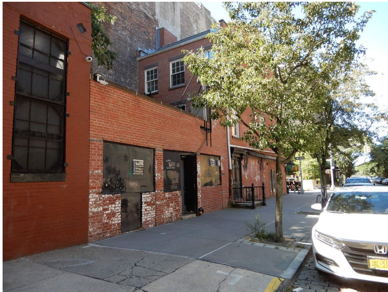
West 12th Street, Looking West
