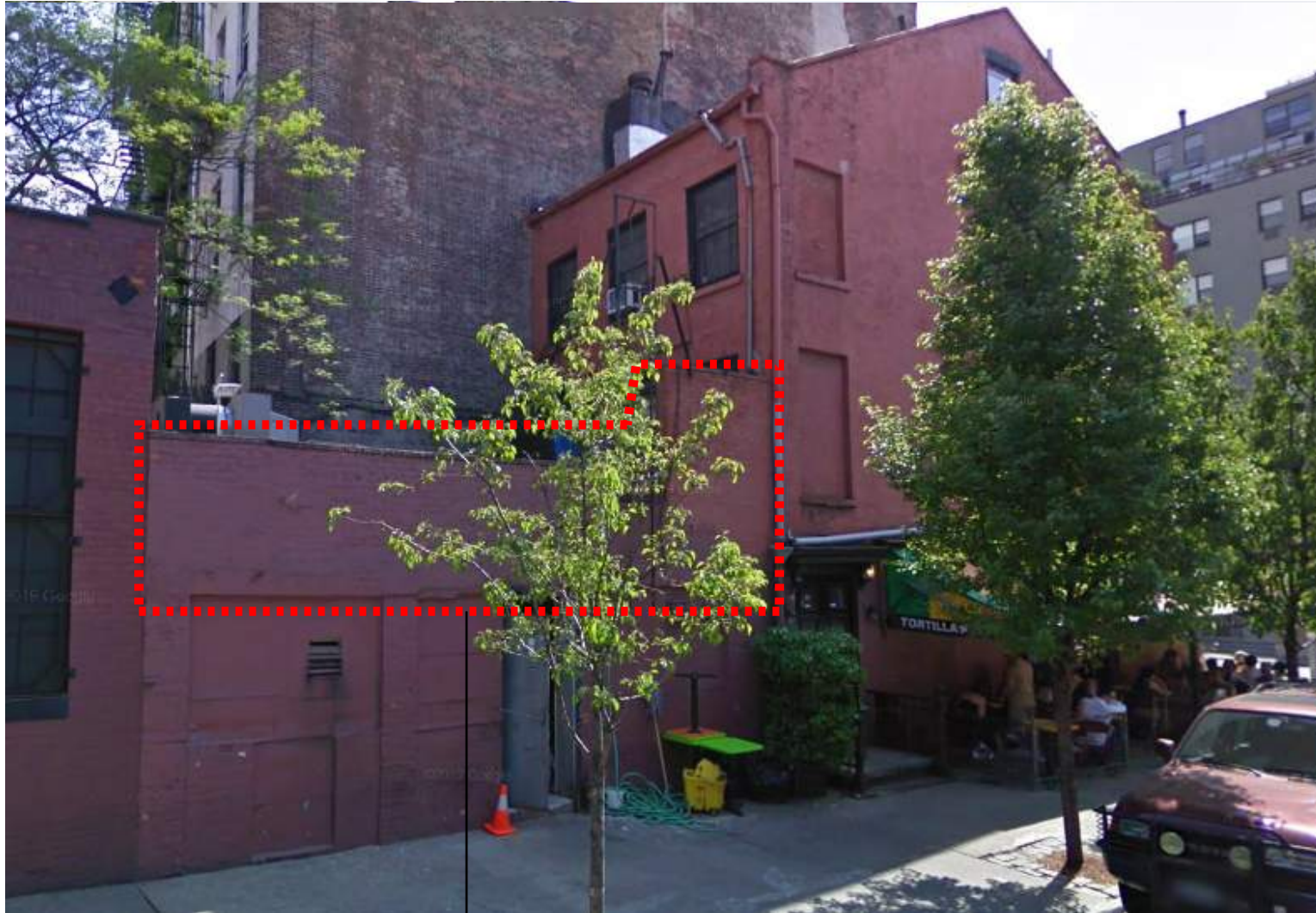
Rear Addition as of 2018, before Copping, parapet and stone lintel removed under #CNE-132234
