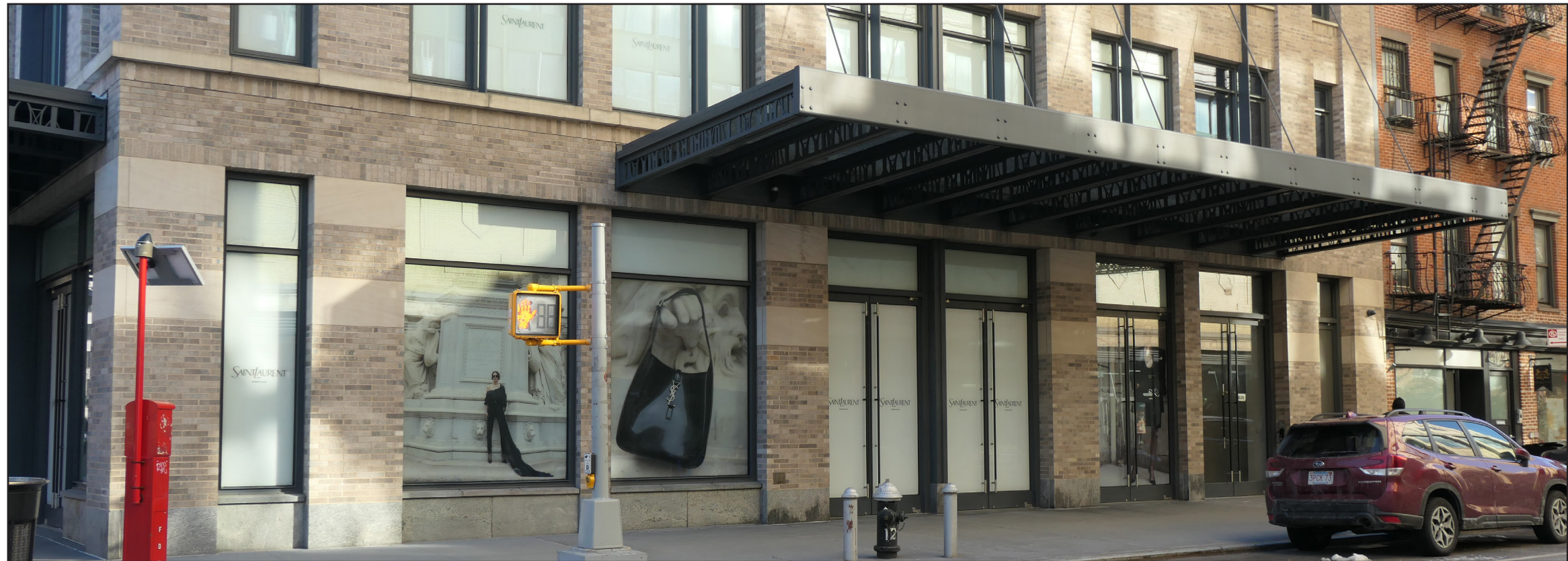
WASHINGTON STREET FACADE - EXISTING CONDITION
