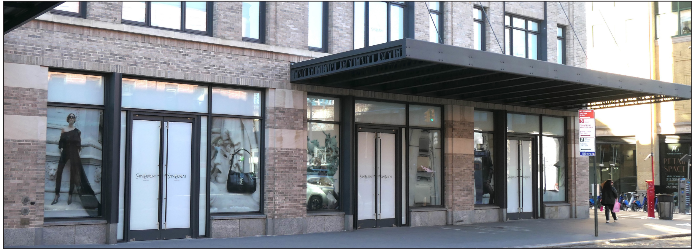
GANSEVOORT STREET FACADE - EXISTING CONDITION
