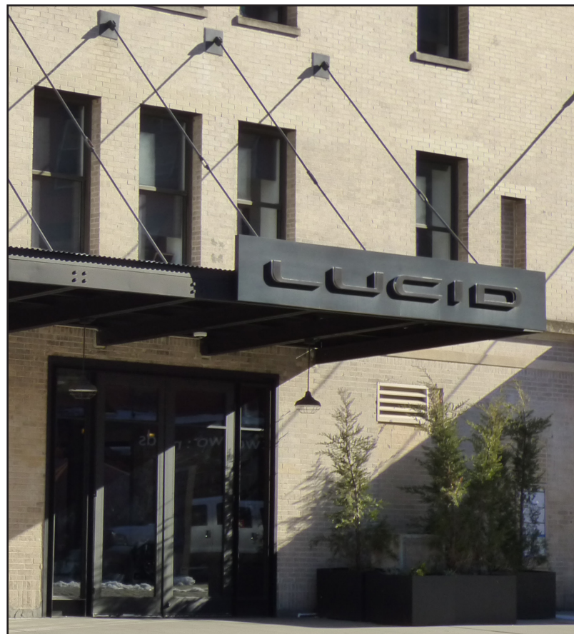
2 9TH AVENUE, PANEL SIGNAGE APPROVED 2020
