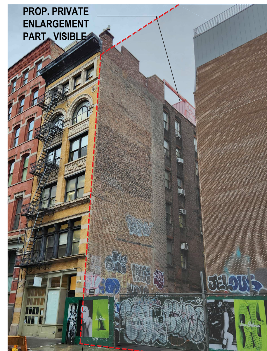
VIEW 7: ALONG WOOSTER STREET PROPOSED ADDITION IS PARTIALLY VISIBLE
