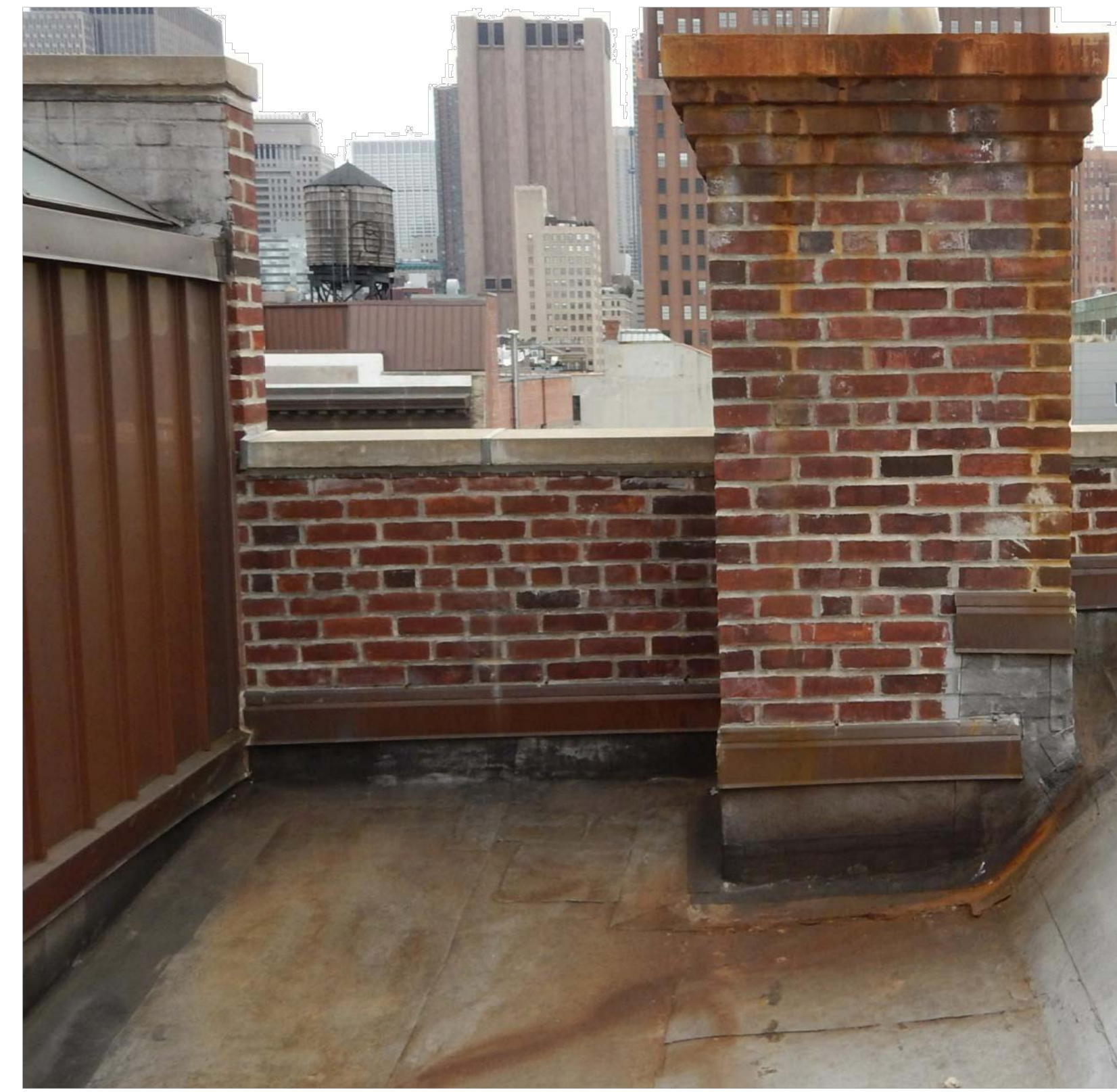
7 ROOF LEVEL PARAPET, LOOKING WEST
