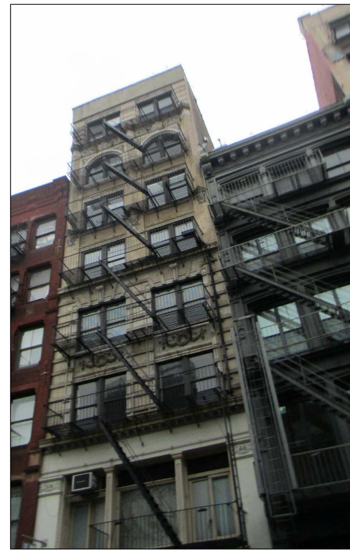
9 METAL FIRE ESCAPES
