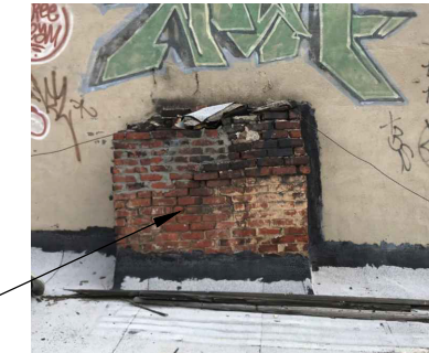
PHOTO OF EXISTING BRICK CHIMNEY
