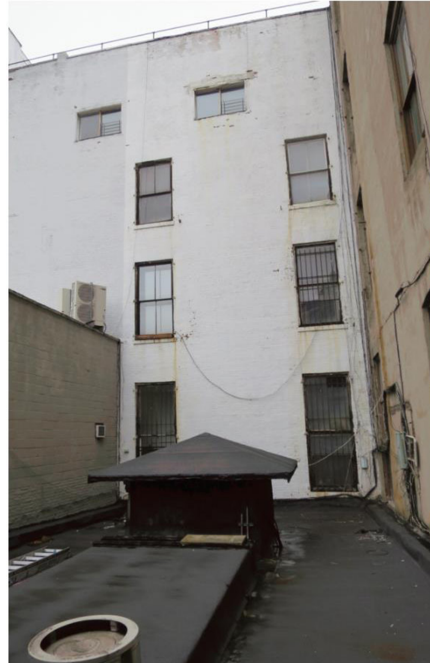
ROOF OF EXTENSION AT REAR, LOOKING WEST.
