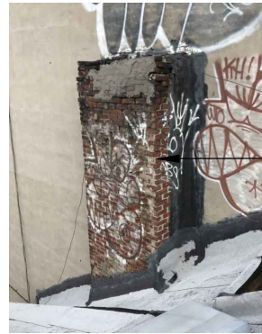
PHOTO OF EXISTING BRICK CHIMNEY
