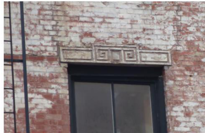
WINDOW LINTEL AT SECOND FLOOR. PAINTED BROWNSTONE WITH SOME MINOR DAMAGE.
