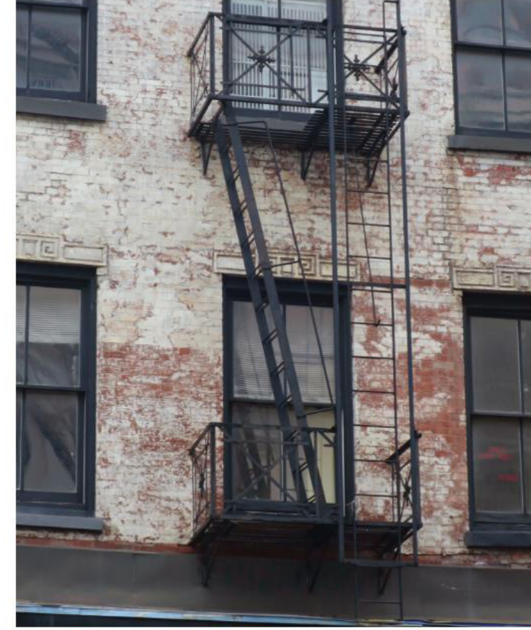
CENTRAL BAY FIRE ESCAPE.
