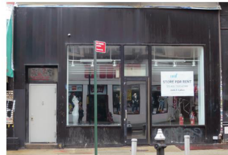
423 BROADWAY NON-HISTORIC ALUMINUM STOREFRONT. NO HISTORIC STRUCTURE OR FABRIC REMAINS.
