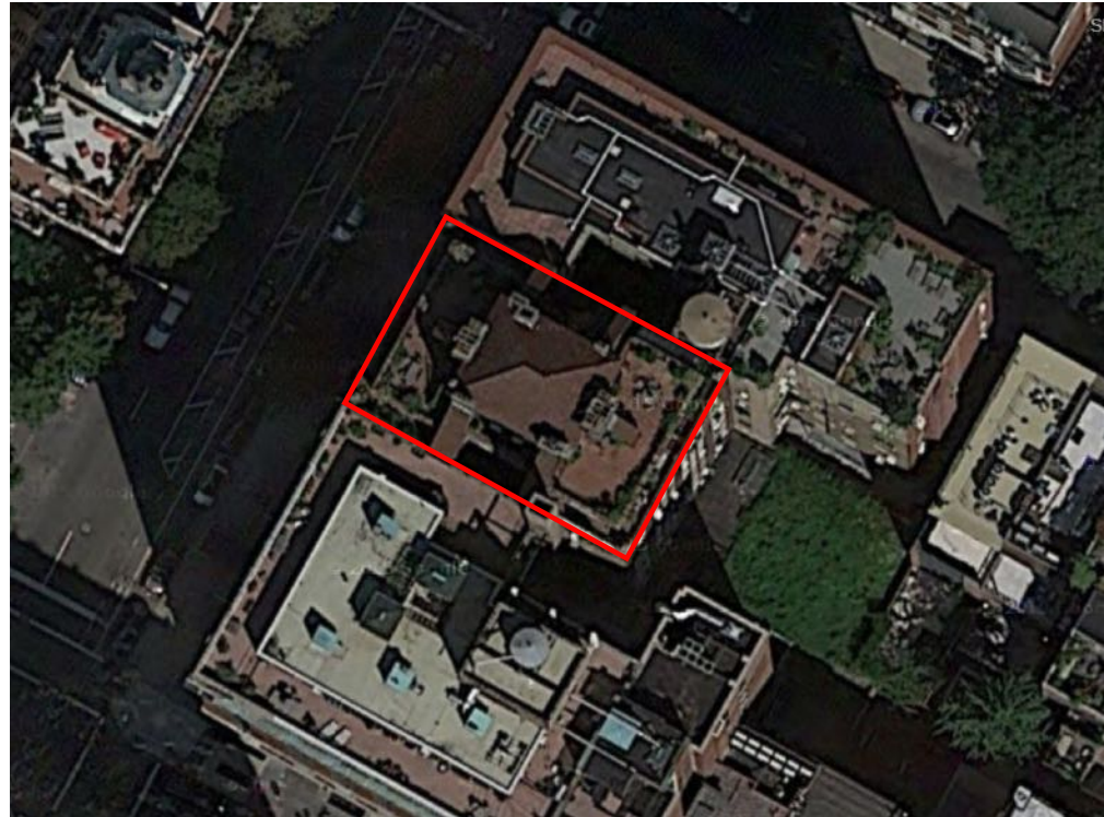
IMAGE 1 - AERIAL VIEW GOOGLE MAPS
