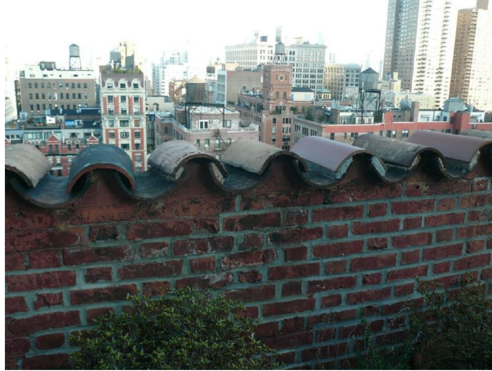
DETAIL VIEW OF EXISTING PARAPET WALL
