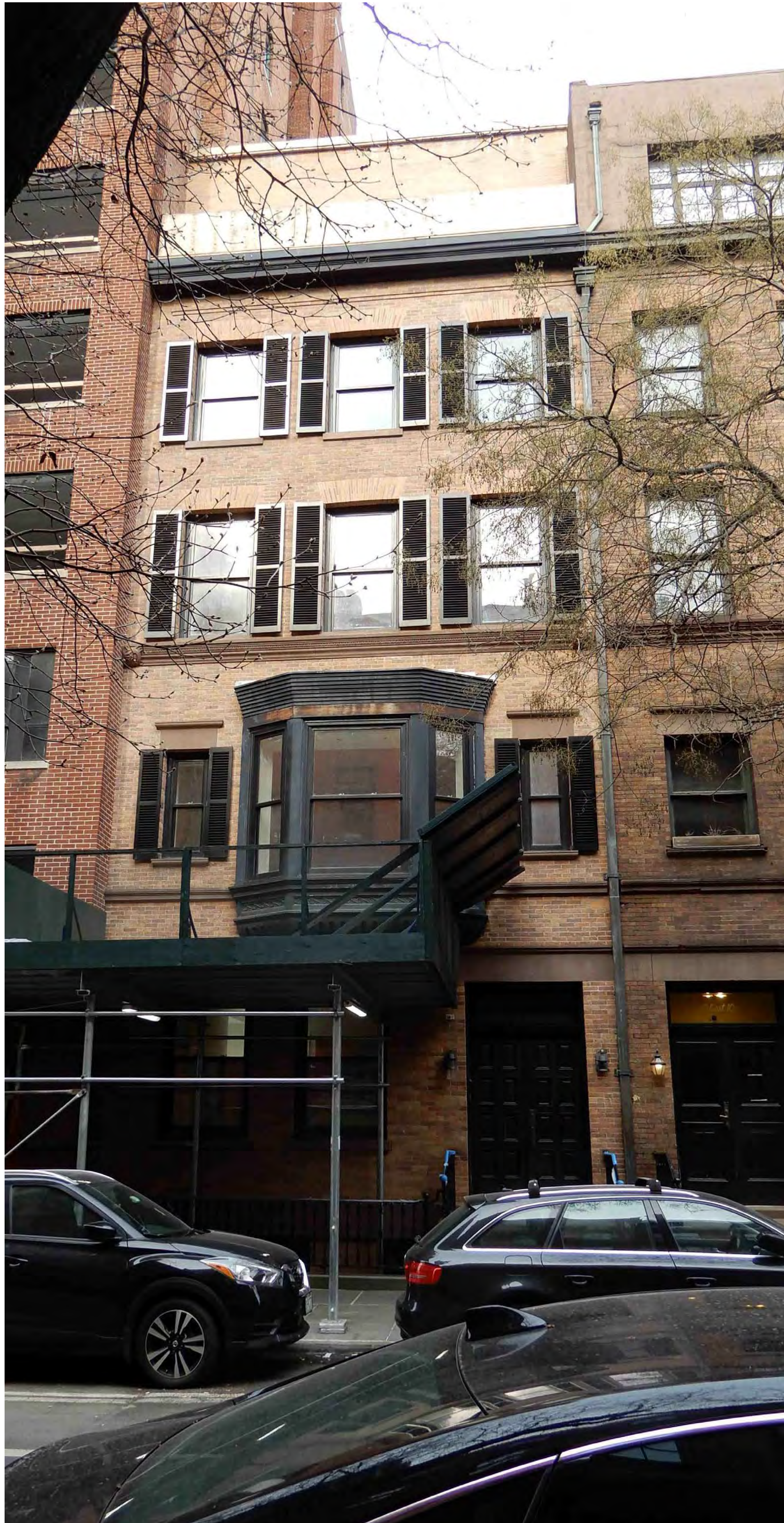
1 FRONT FACADE EXISTING 1" = 50'-0"
