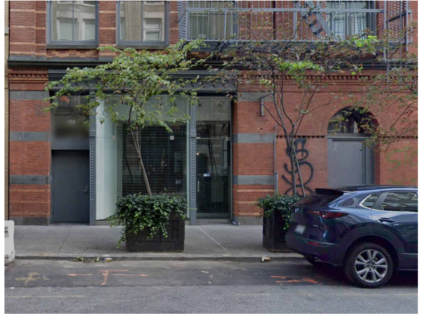
EXISTING CONDITIONS- PRINCE STREET STOREFRONT
