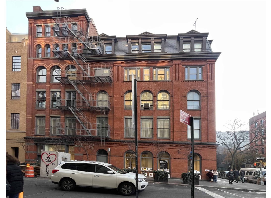
EXISTING CONDITIONS- PRINCE STREET
