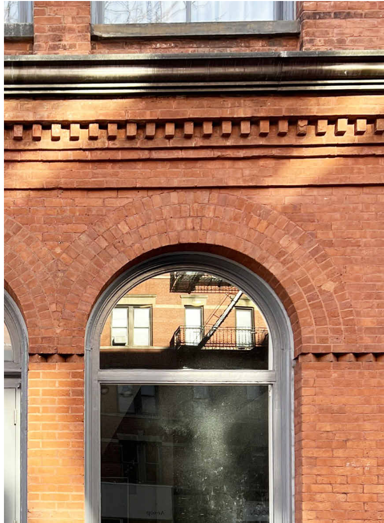
EXISTING CONDITIONS- TYPICAL BRICKWORK
