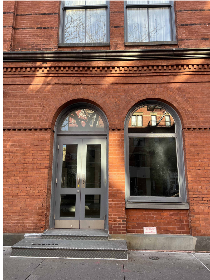
EXISTING CONDITIONS- WEST BROADWAY ENTRANCE
