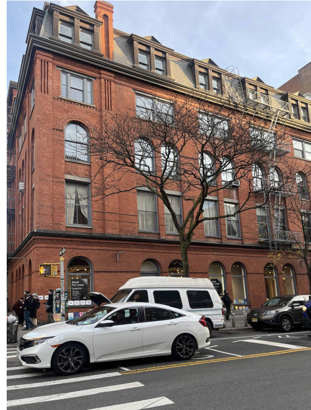
EXISTING CONDITIONS- WEST BROADWAY
