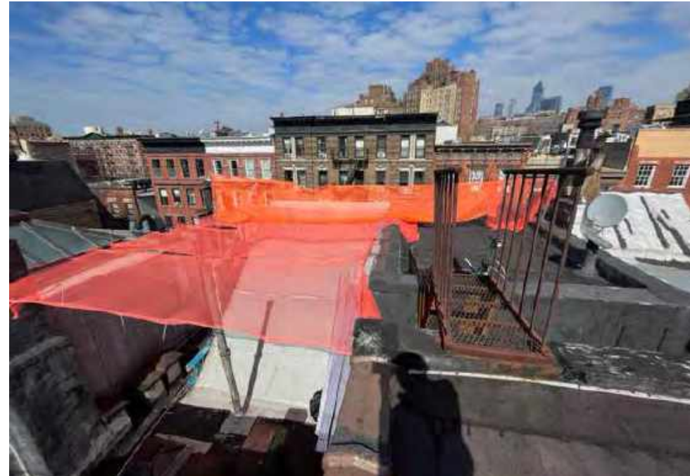
VIEW LOOKING NORTH
