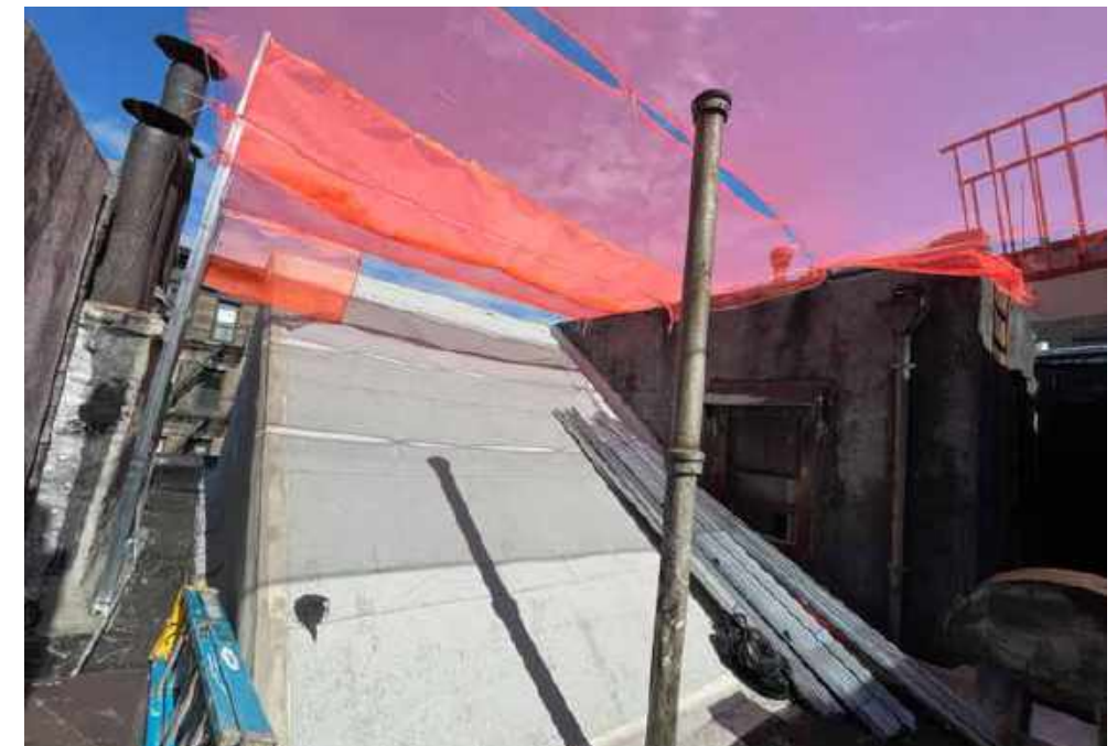
VIEW LOOKING NORTH BETWEEN EXISTING SKYLIGHTS
