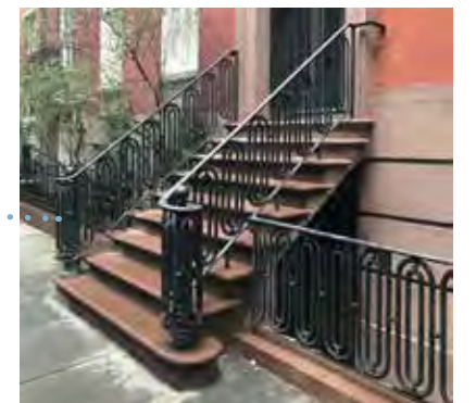
BROWNSTONE STOOP, NATURAL BRICK, BLACK METAL RAILINGS AND FENCE TO MATCH 278 WEST 11TH STREET.
