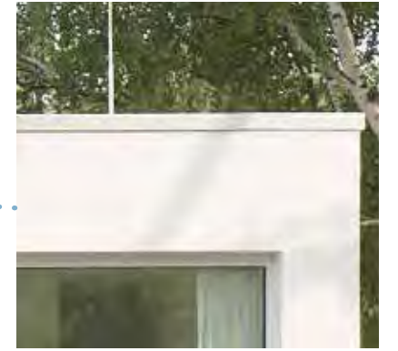
LIGHT STUCCO SIDING WITH PAINTED METAL FASCIA.
