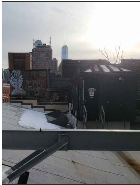
5 VIEW OF FREIGHT ELEVATOR FROM NORTH SIDE
