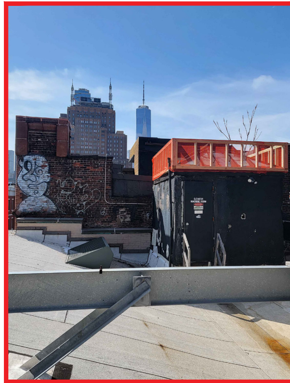
5* VIEW OF FREIGHT ELEVATOR FROM NORTH SIDE
