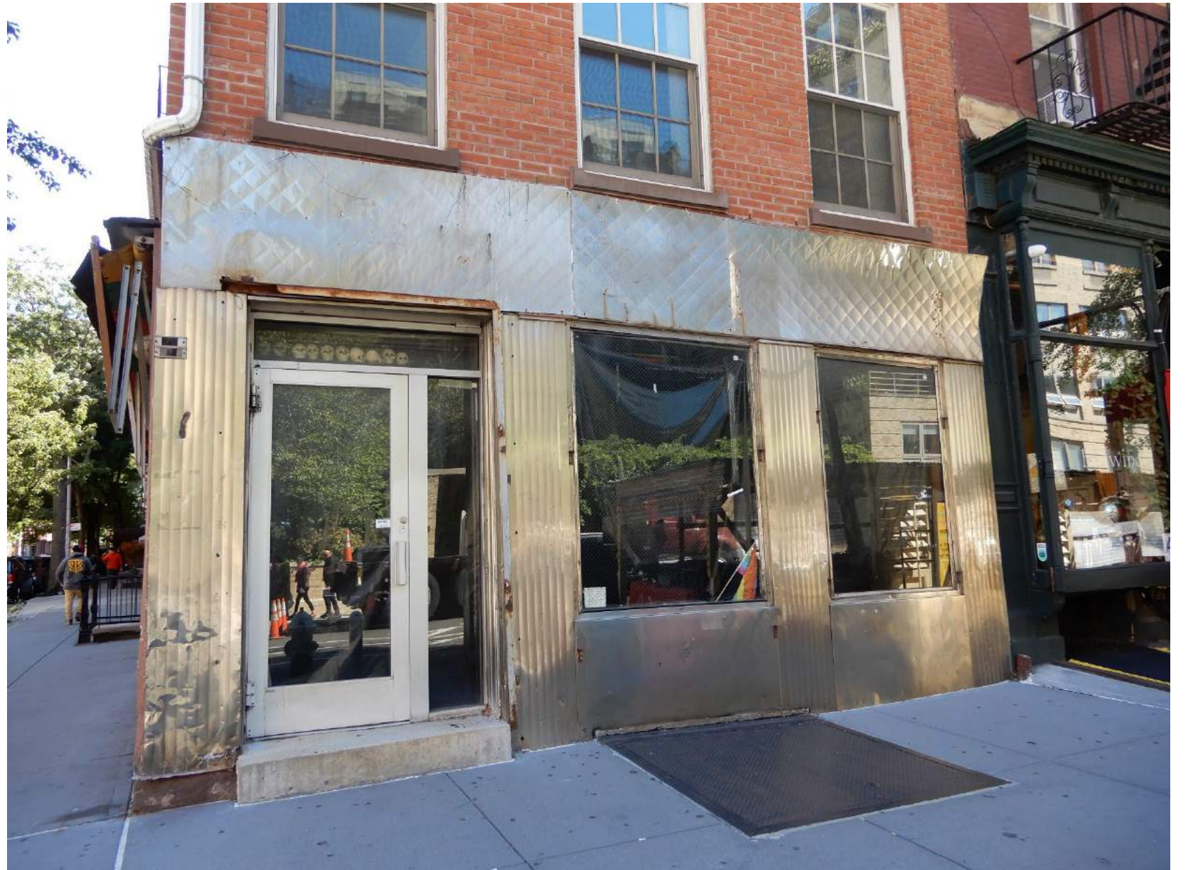
Storefront, Washington Street
