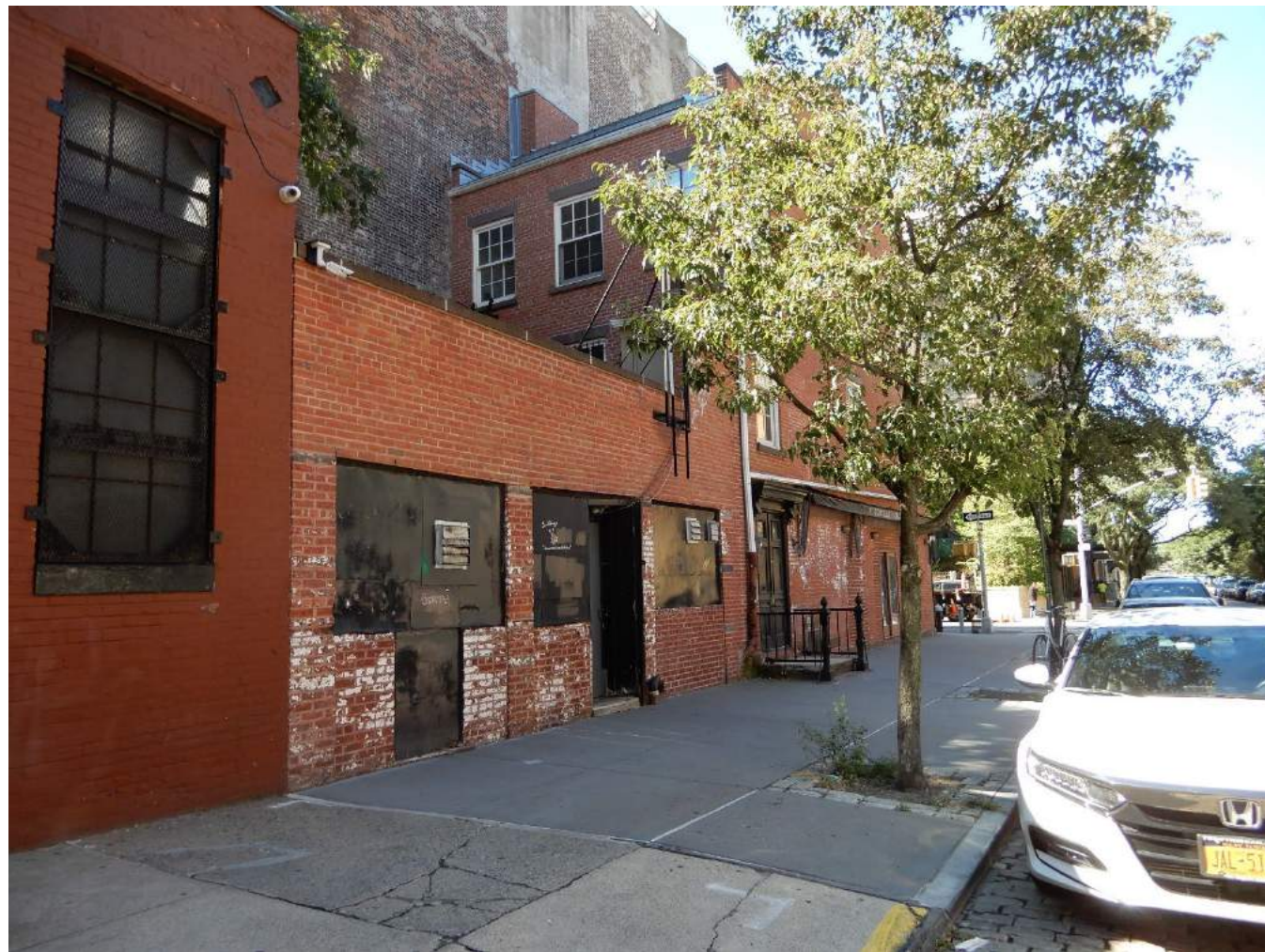
West 12th Street, Looking West
