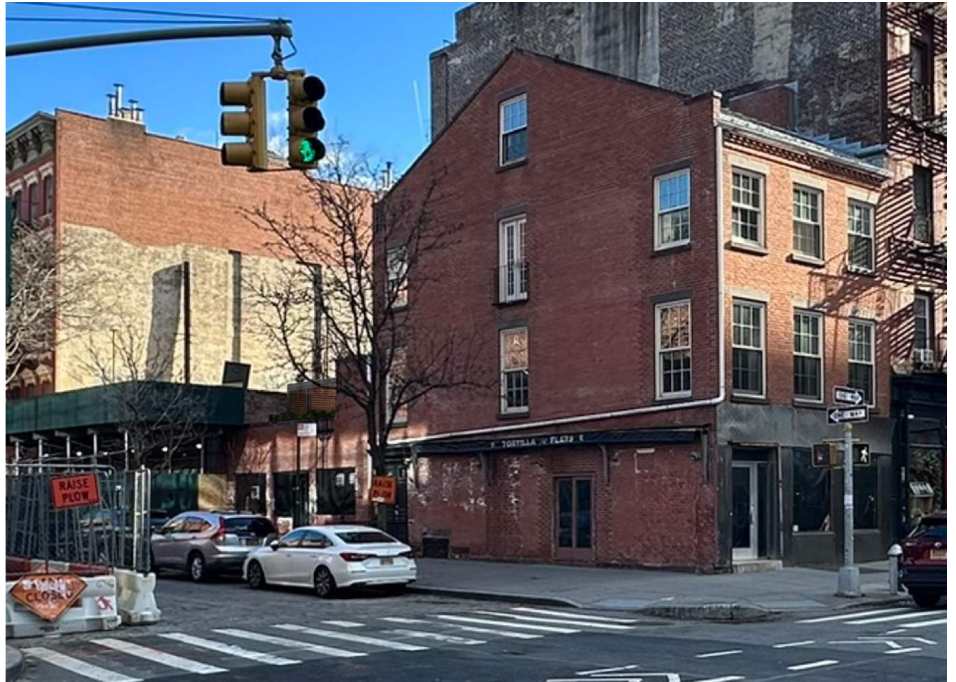
View from Washington Street North West Side
