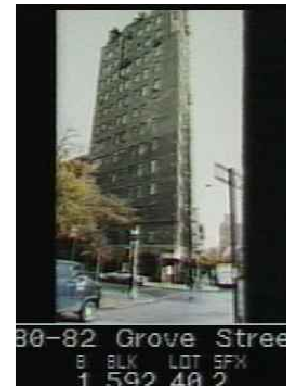
⑥ EXIST FACADE PICT. 10 SHERIDAN SQUARE (BUILT 1929)
