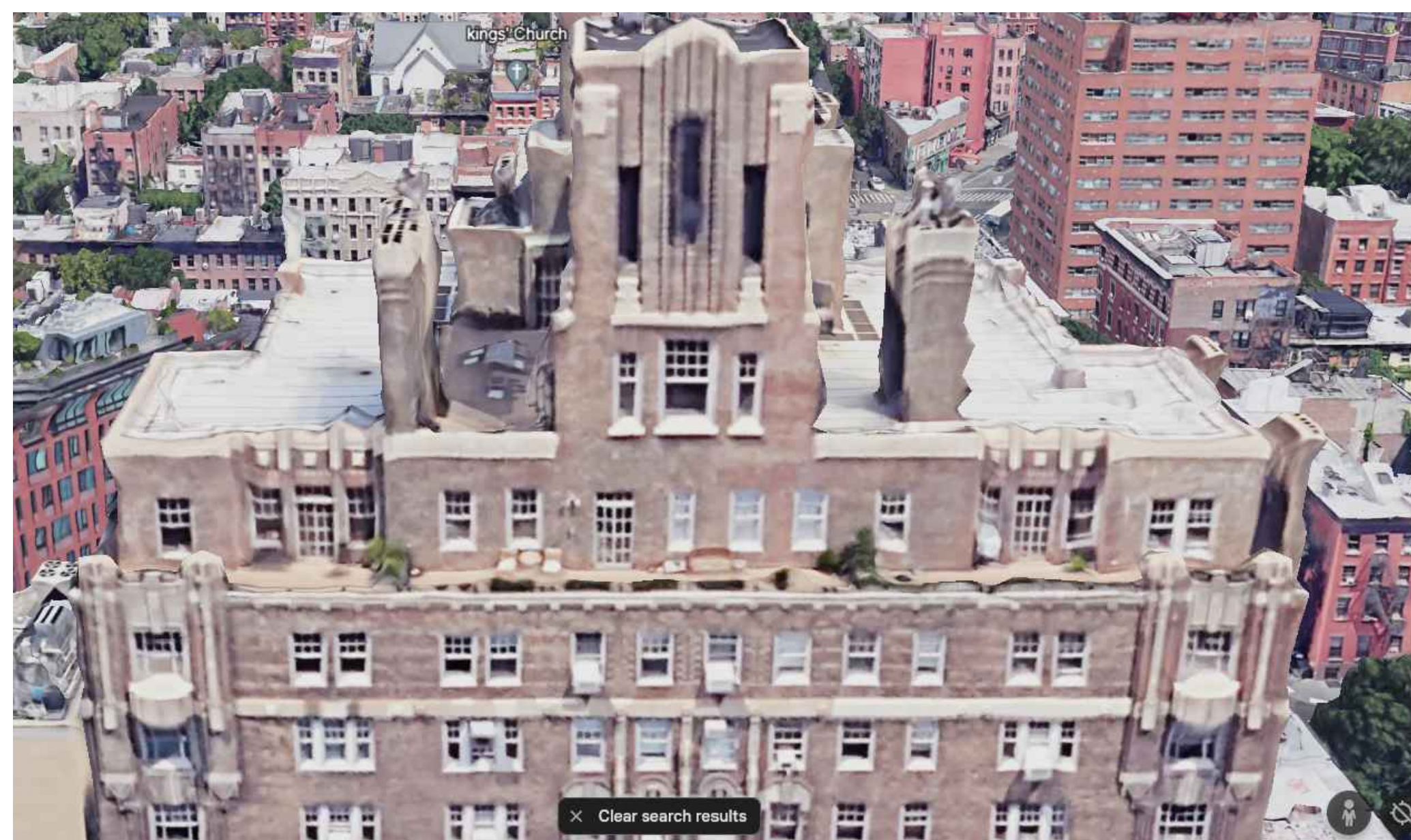
EXIST FACADE PICT. 45 CHRISTOPHER STREET (BUILT 1931) ⑤
