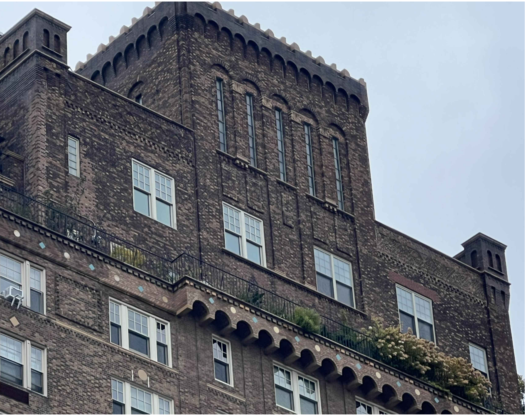
EXIST SOUTH FACADE PICT.
