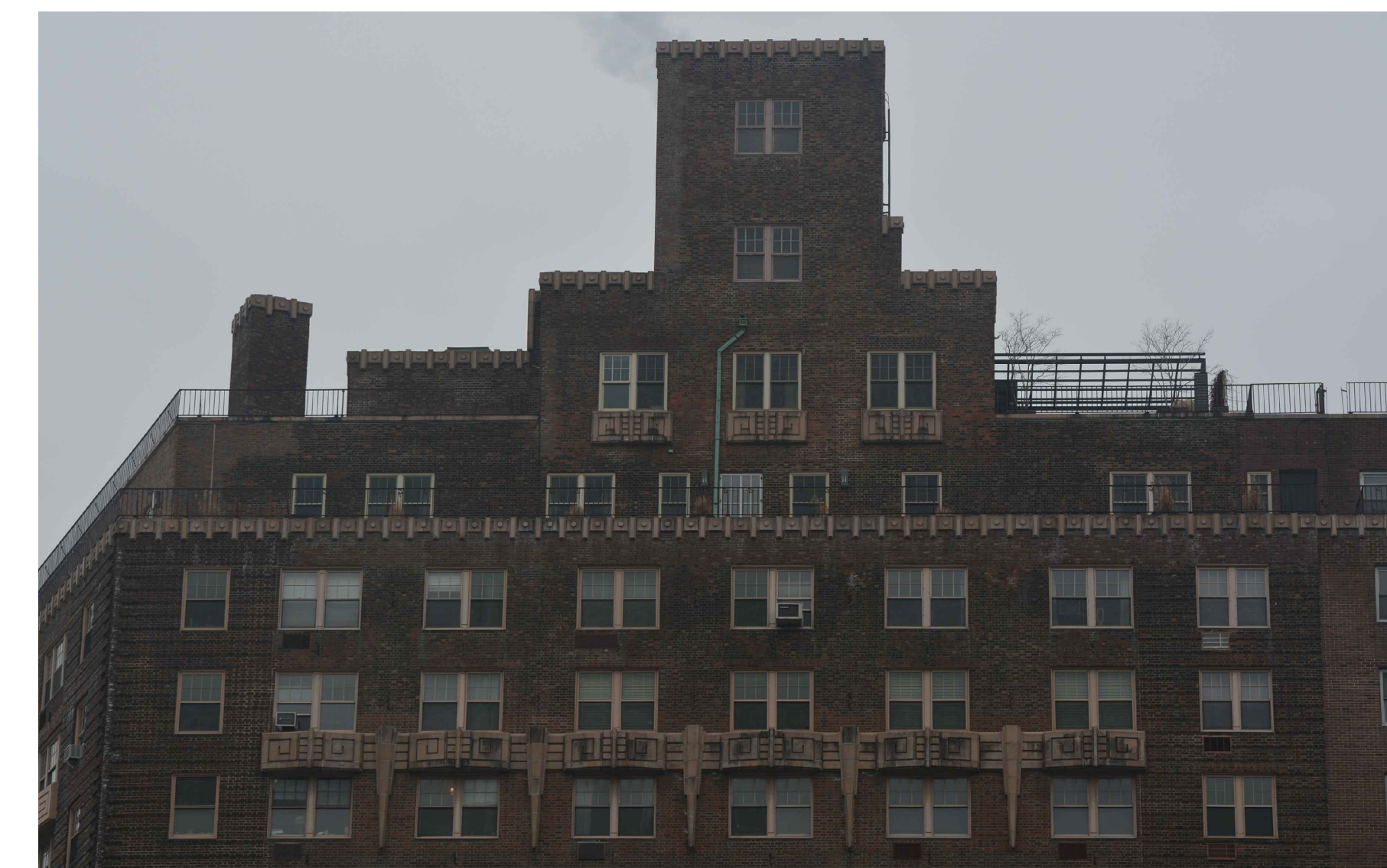
④ EXIST FACADE PICT. 2 HORATIO STREET (BUILT 1931)
