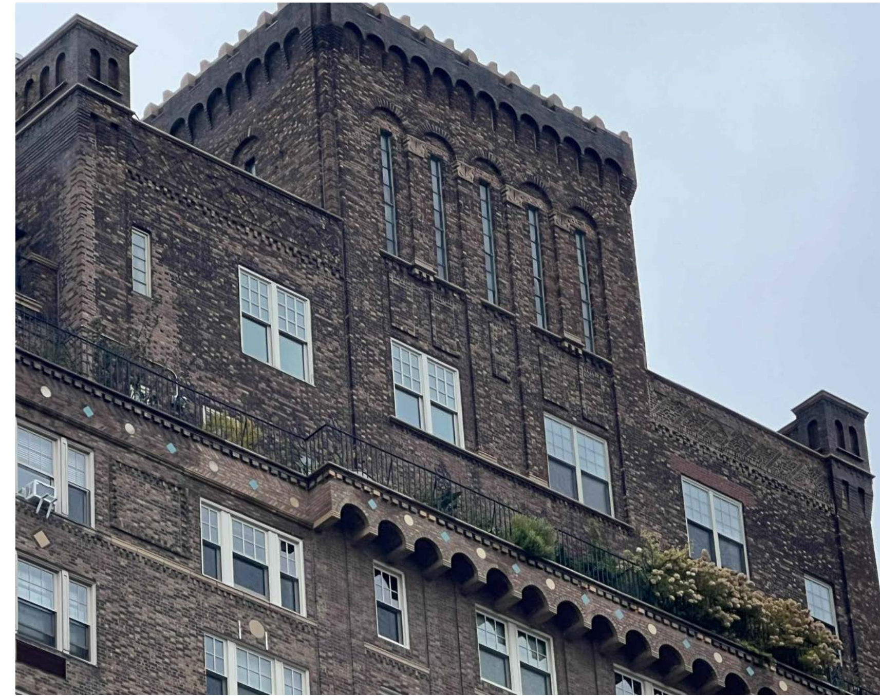
EXIST SOUTH FACADE PICT.
