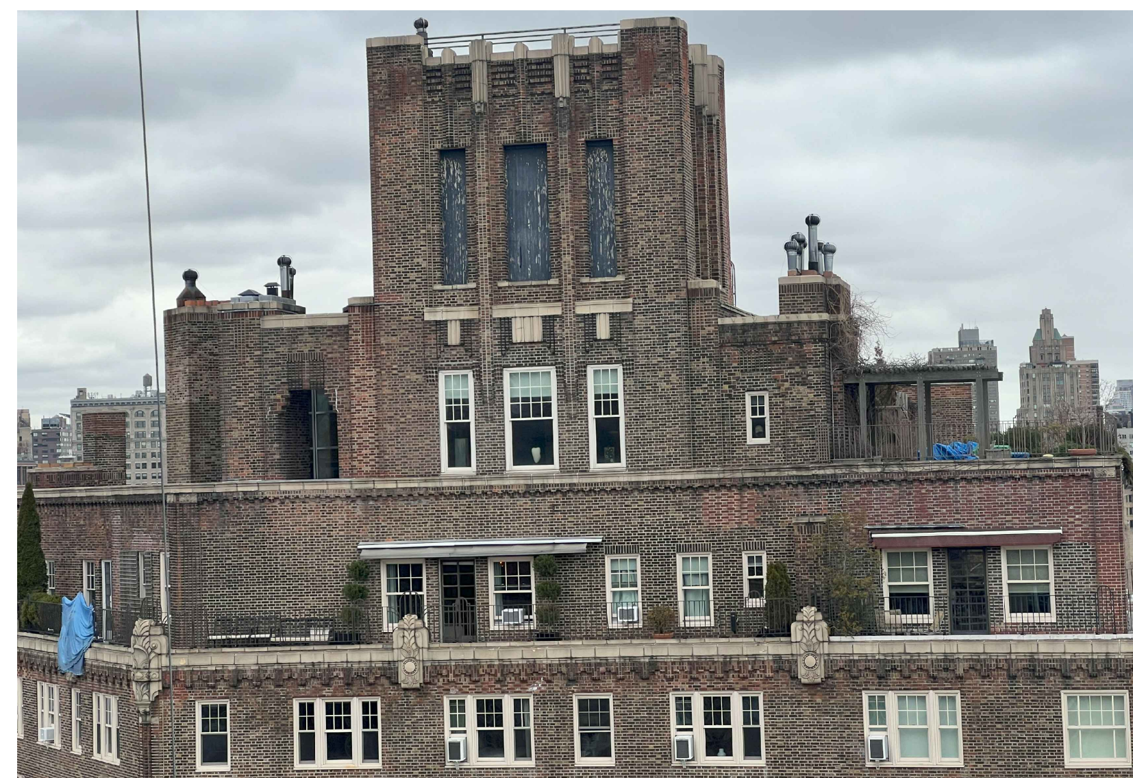
EXIST FACADE PICT. 302 WEST 12TH STREET (BUILT 1931) ③
