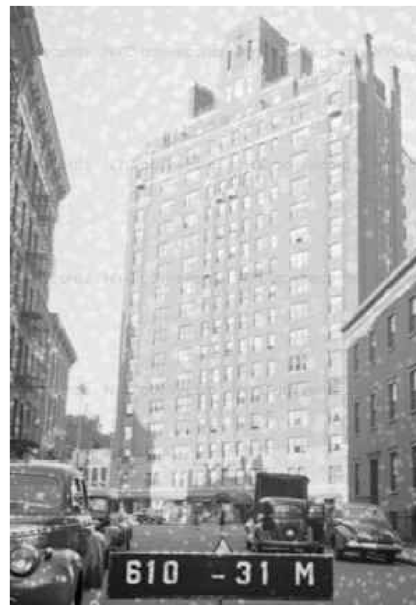
EXIST FACADE PICT. 45 CHRISTOPHER STREET (BUILT 1931) ⑤
