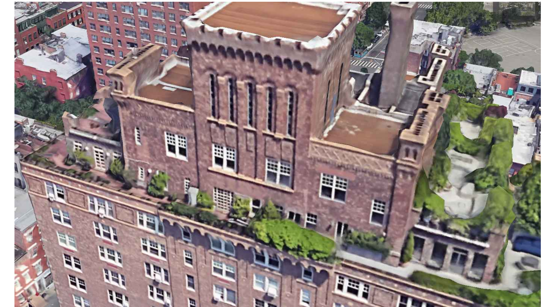
② EXIST SOUTH FACADE PICT. 299 WEST 12TH STREET (BUILT 1931)
