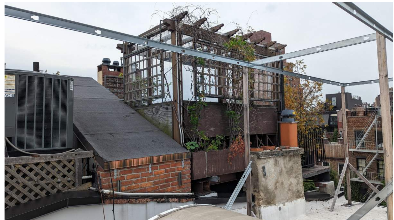
Existing Roof View (Southeast)
