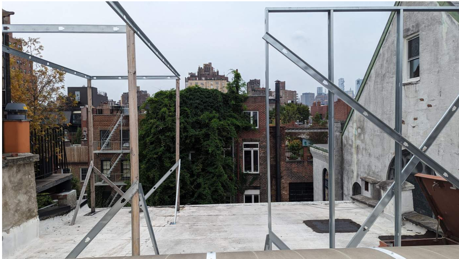
Roof View facing South (rear yard)
