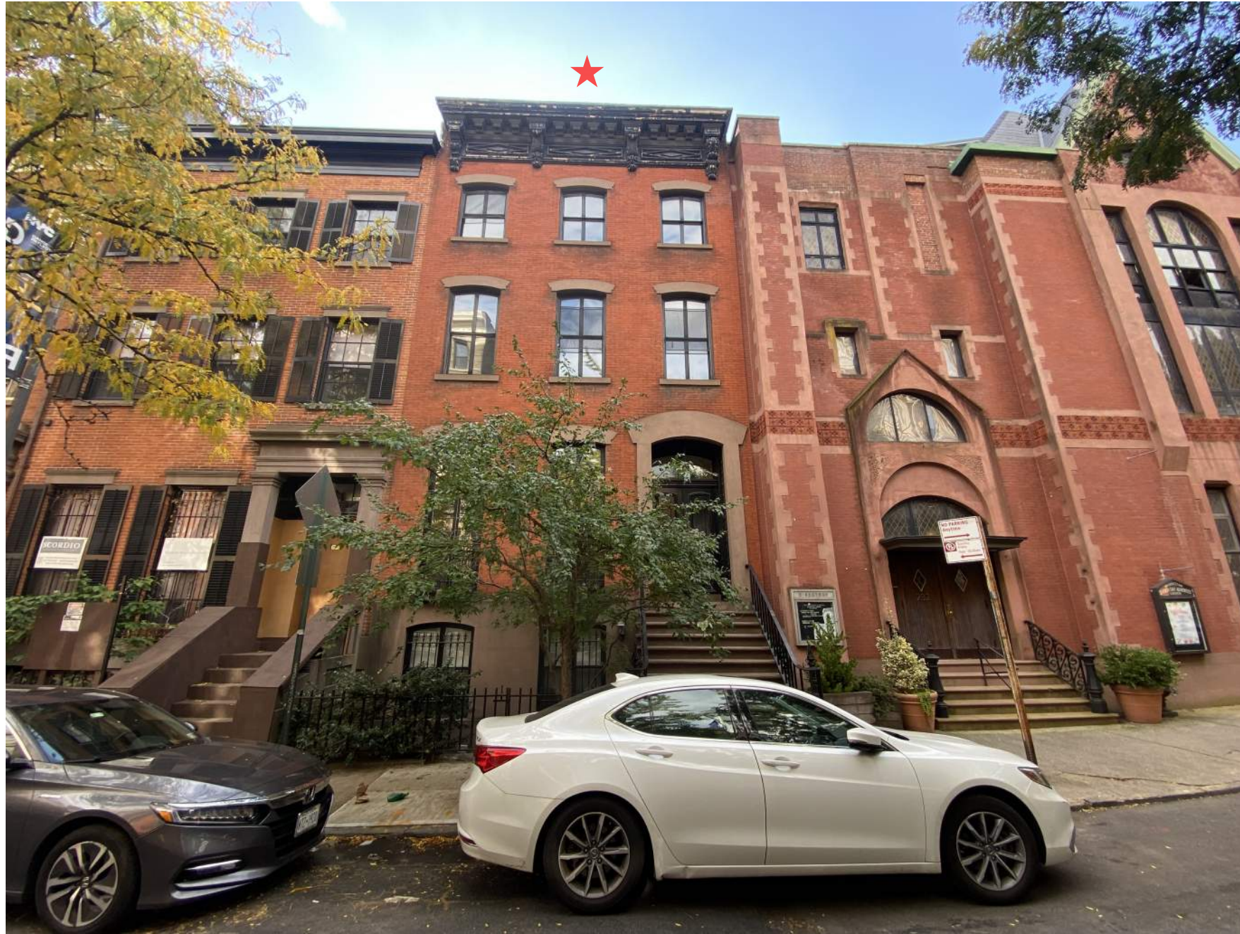
Existing 230 W. 11th Street Facade
