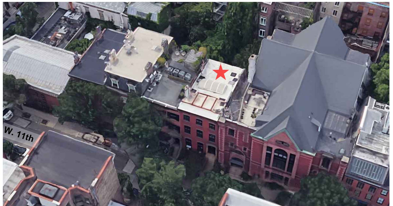
AERIAL VIEW FRONT FACADE
