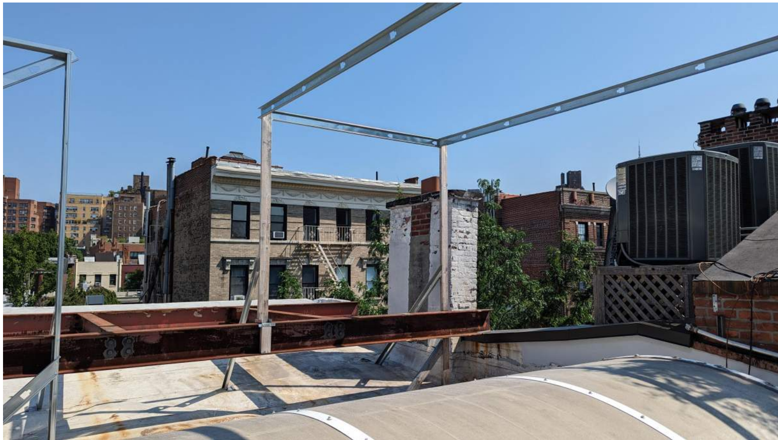
Existing Roof View (Northeast)
