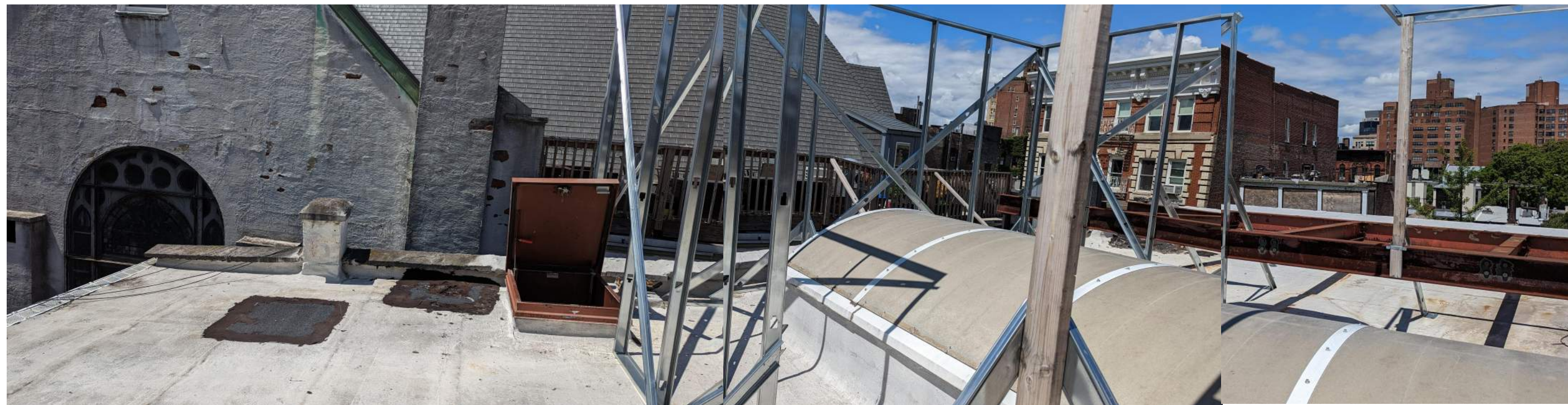
Roof View facing West (towards the Church)
