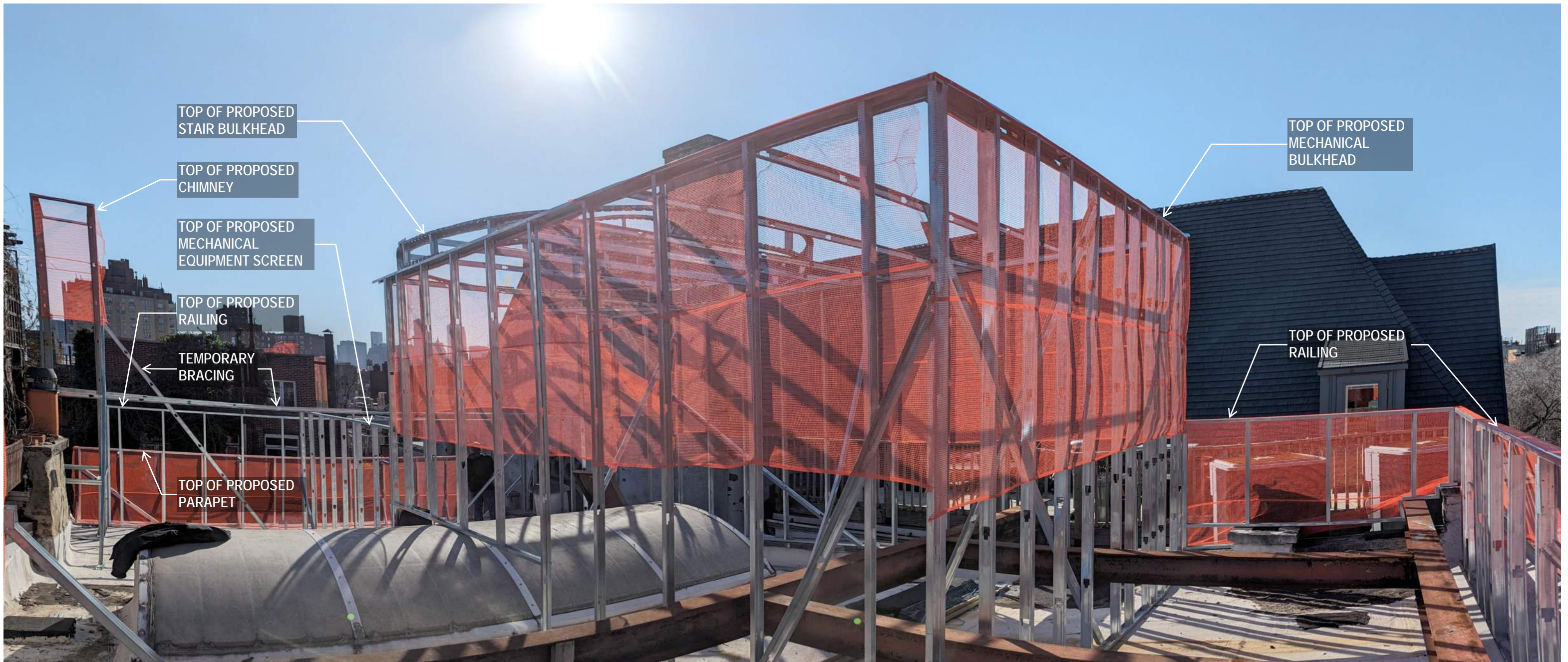
MOCKUP - ROOFTOP VIEW LOOKING SOUTH
