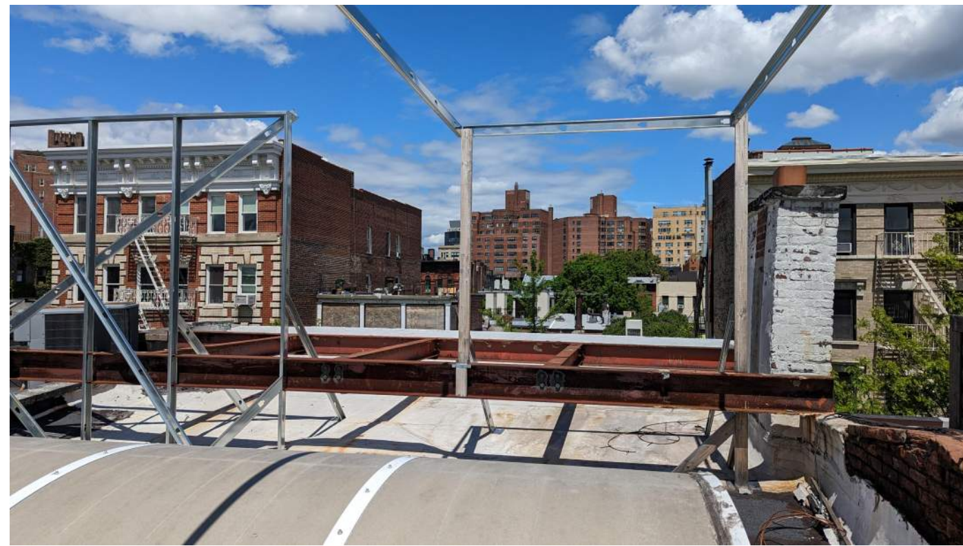
Existing Roof View (North)
