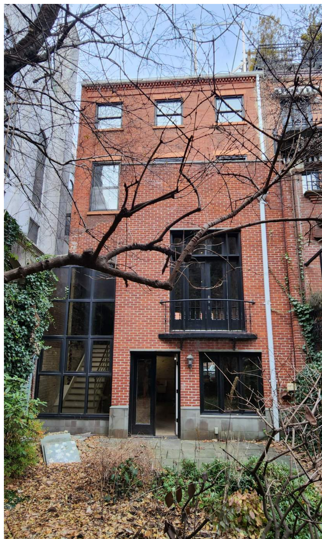
Existing Rear Facade
