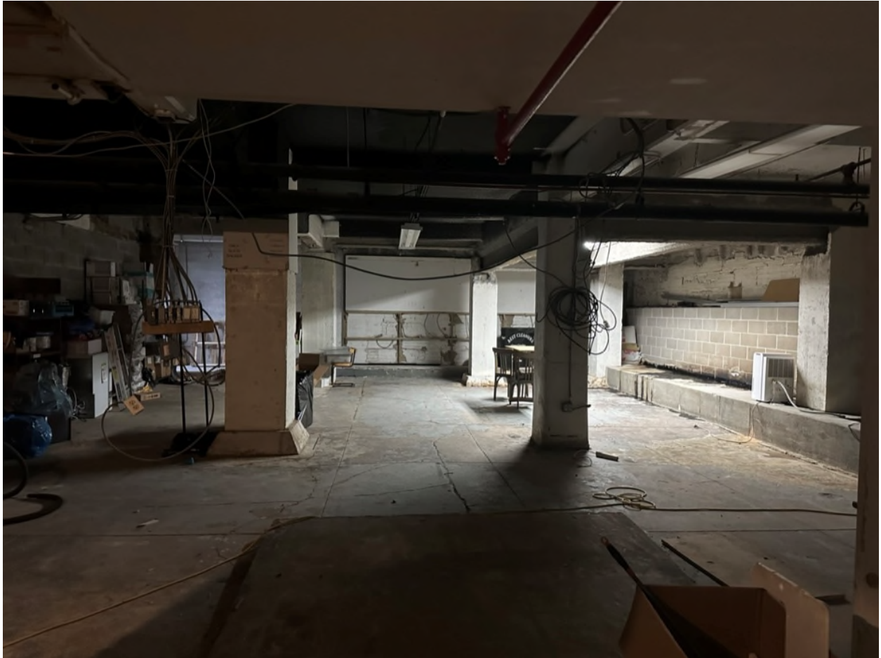
New cellar space
