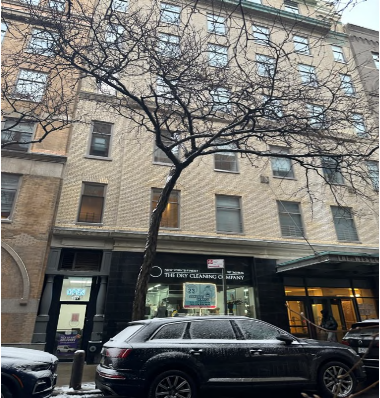
Entrance for new ground floor space
