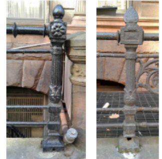
EXISTING NEWEL POSTS: SQUARE BASE
