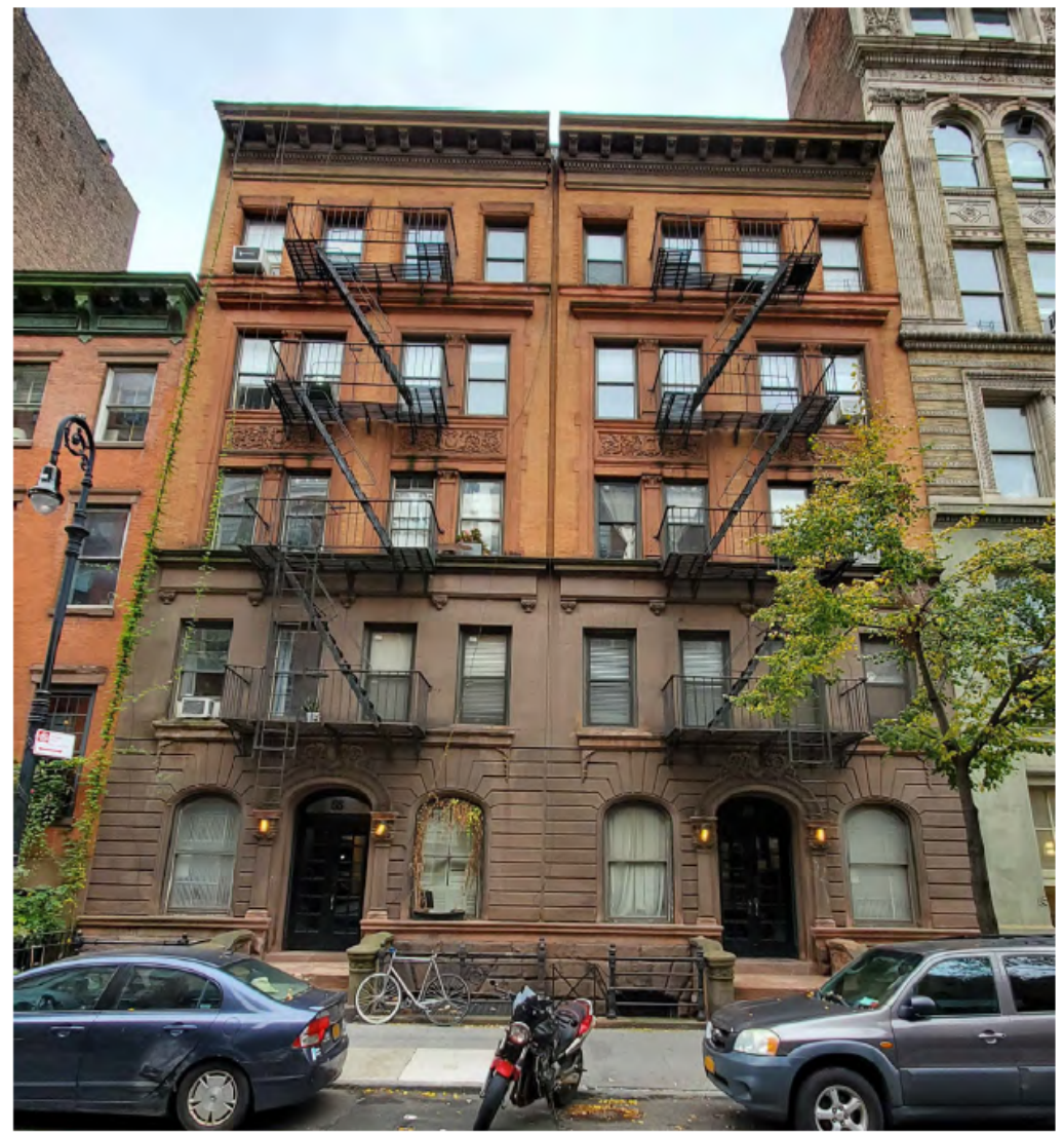
1 EXISTING STREET FACADE @66 & 68 WEST 10TH STREET: 2019
