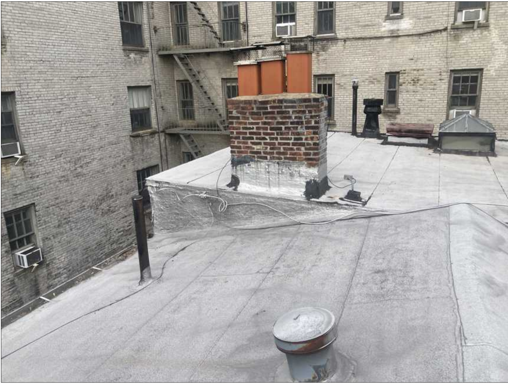
4 grove street - existing roof west
