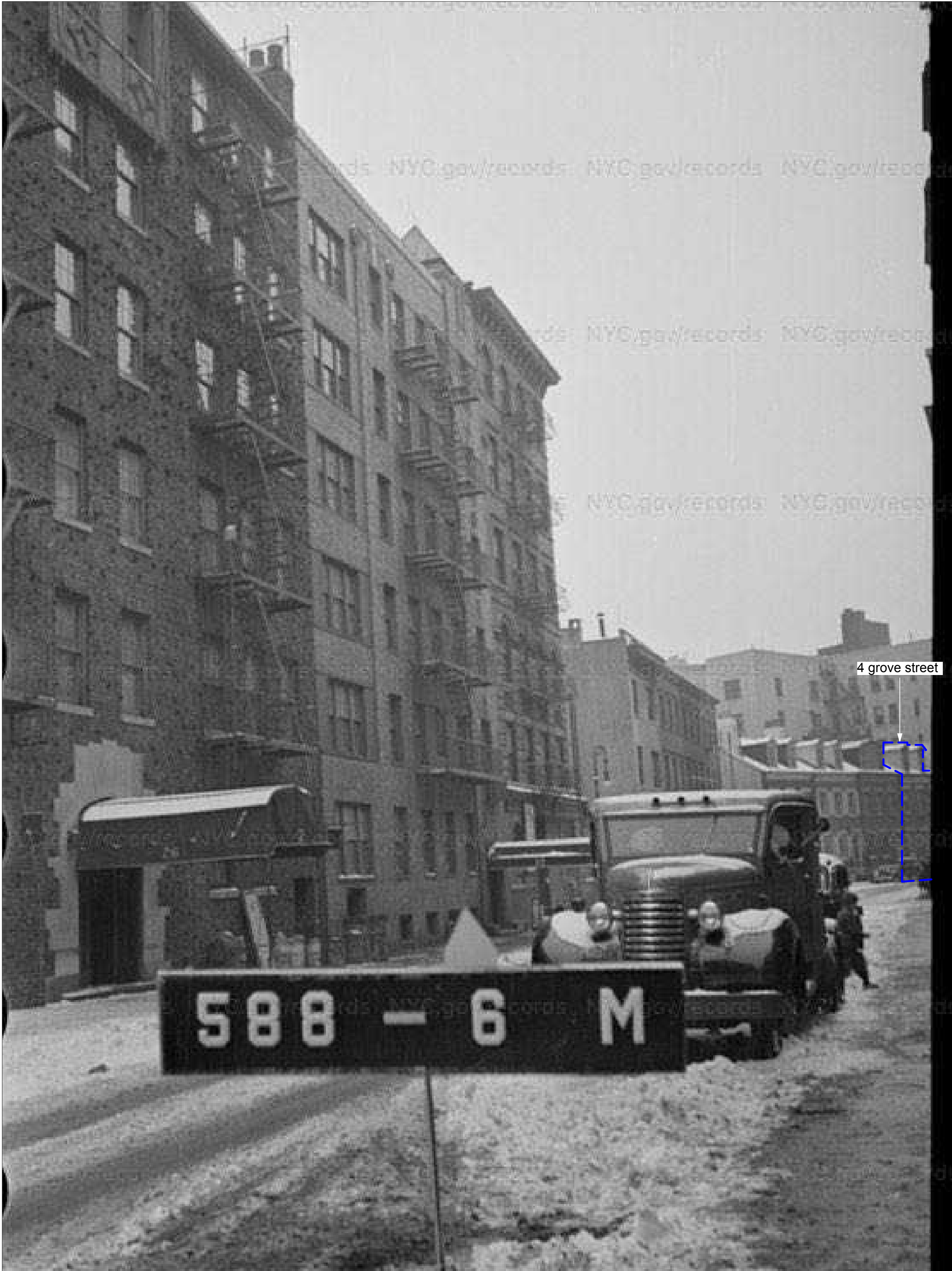
grove street from 26 grove street, facing south west 1940's tax map photograph courtesy: new york city department of finance
