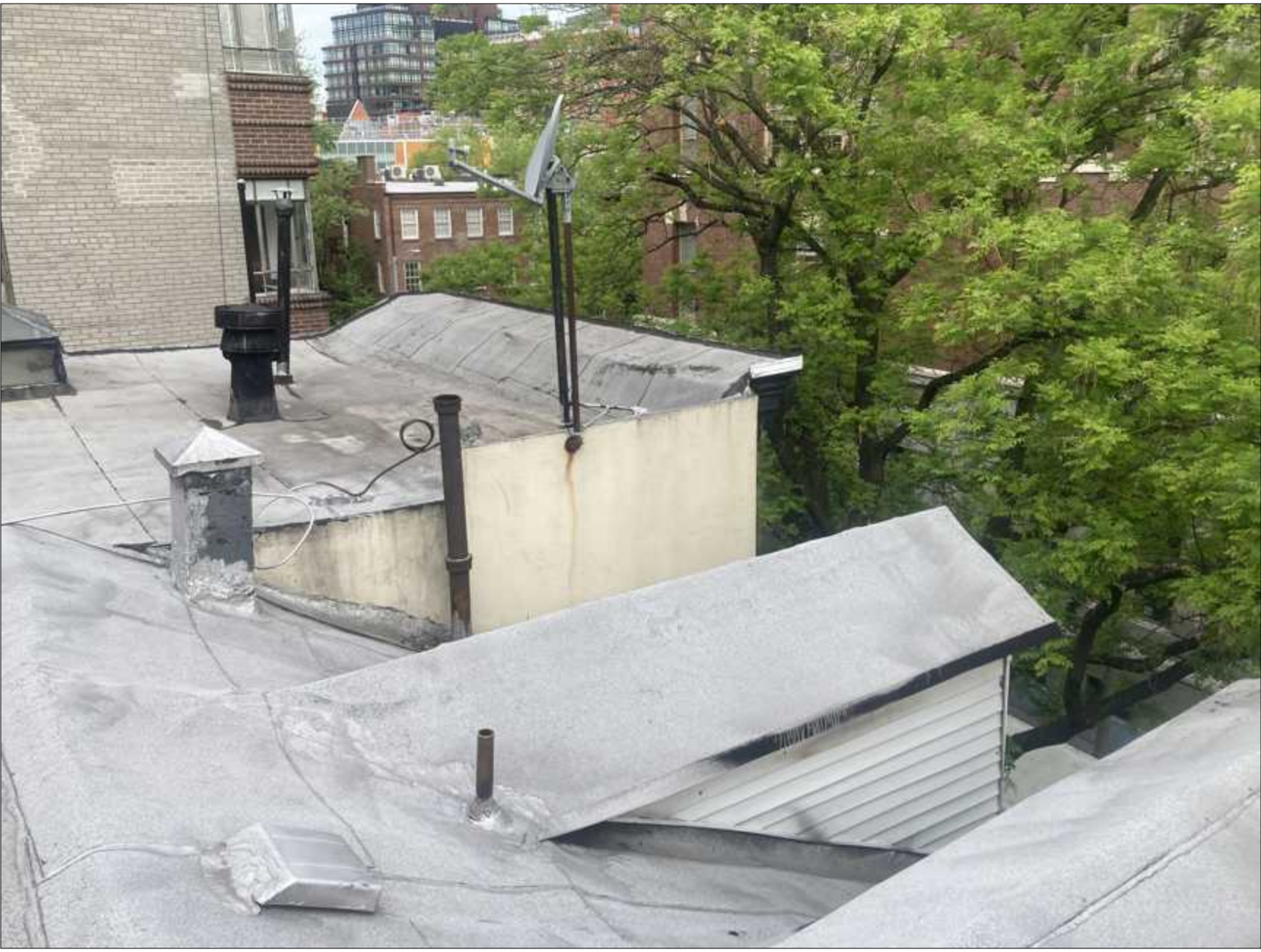
4 grove street - existing roof west
