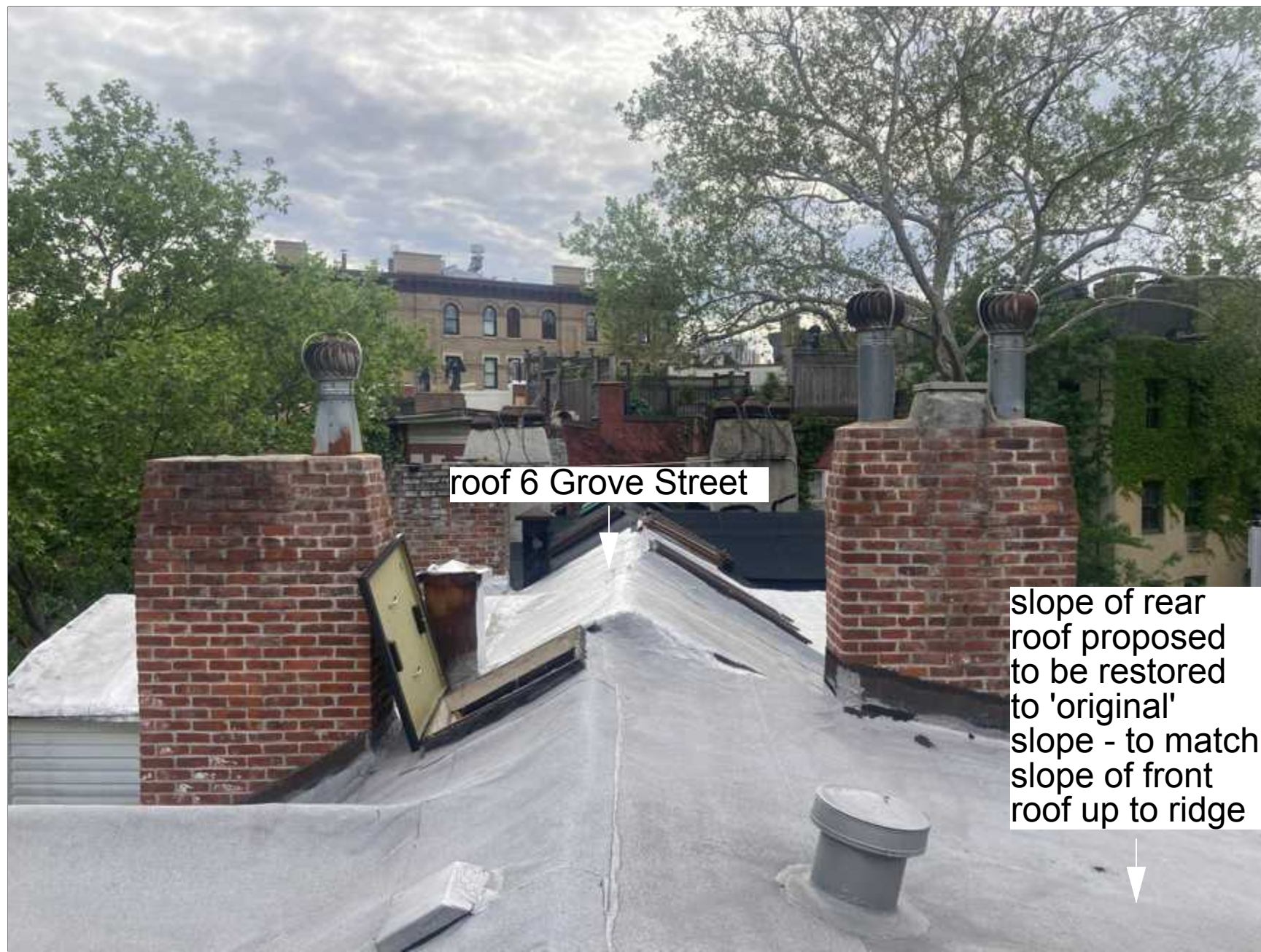
4 grove street - existing roof east
