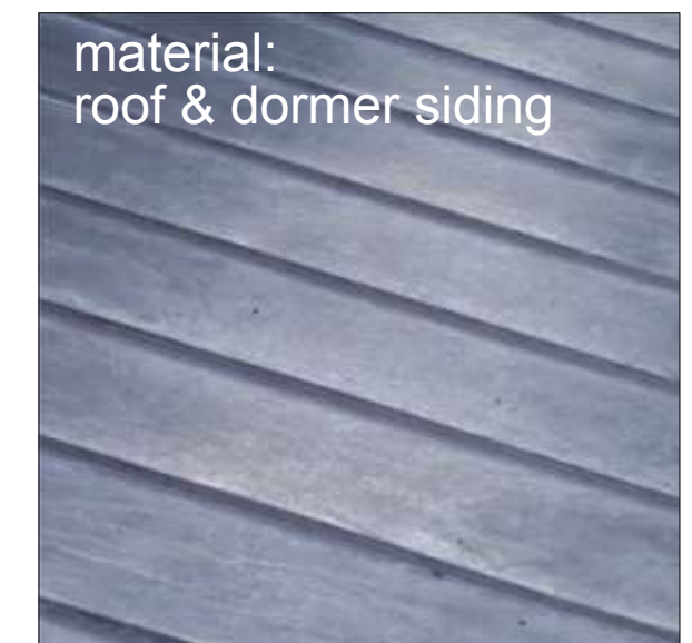
material: roof & dormer siding roofing & dormer siding finish material: lead-coated copper
