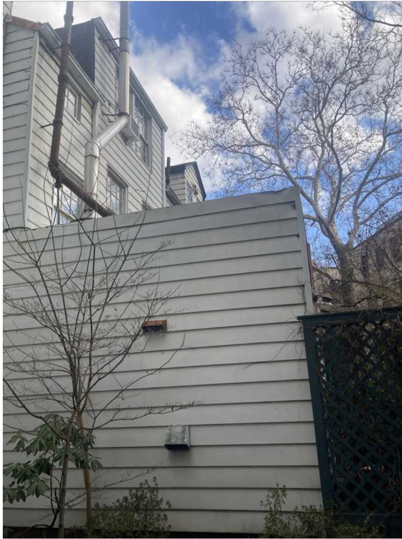
4 grove street - rear facing northeast towards 6 grove street
