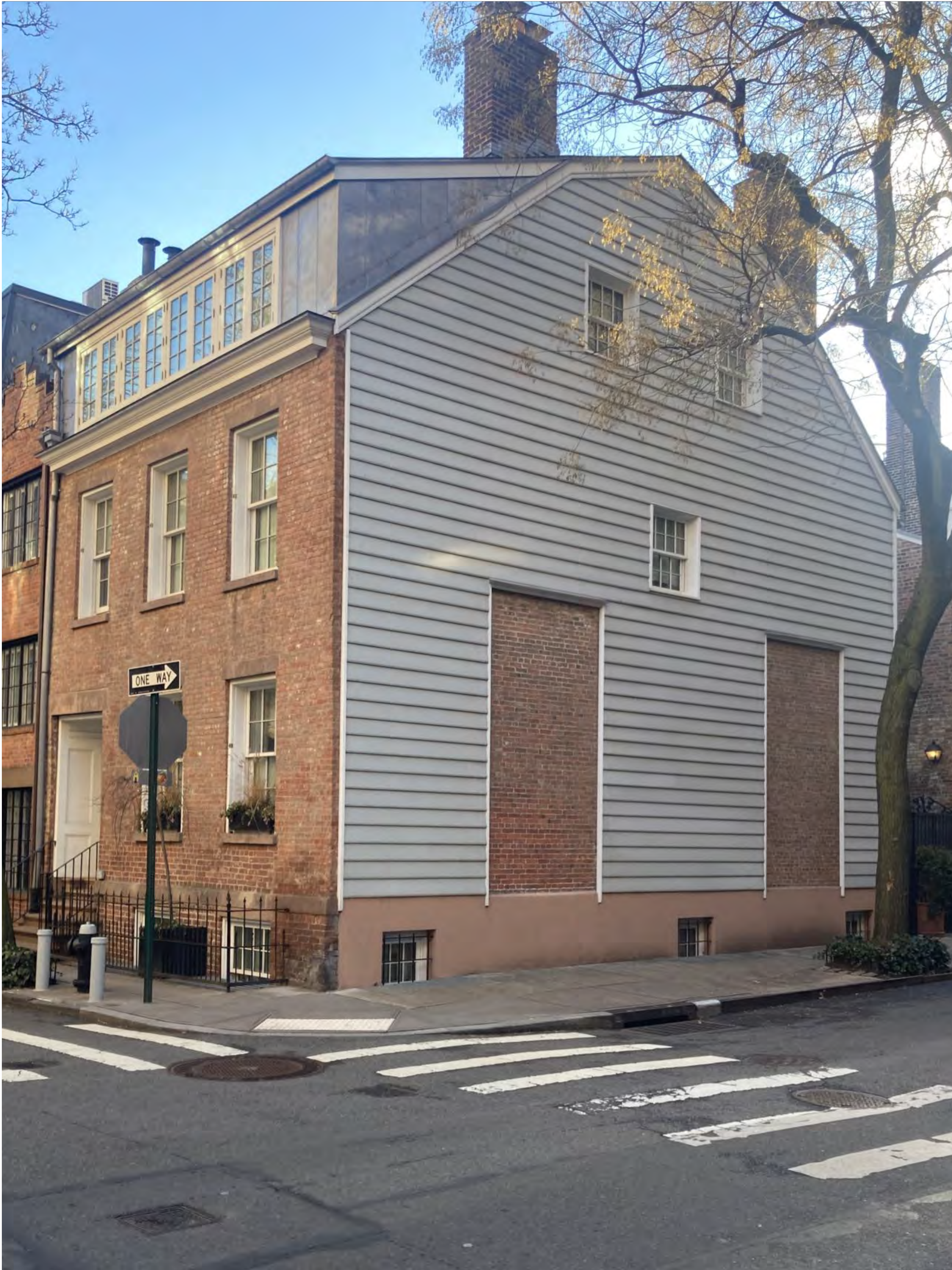
77 bedford street 77 bedford was originally constructed c. 1799-1800; full width front side 'dormer' added c. 1923, with lead-coated copper standing seam was installed c. 2014-16
