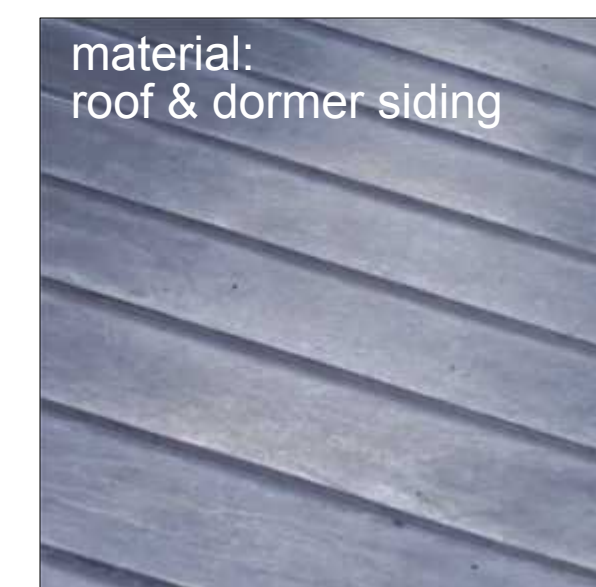
material: roof & dormer siding roofing & dormer siding finish material: lead-coated copper
