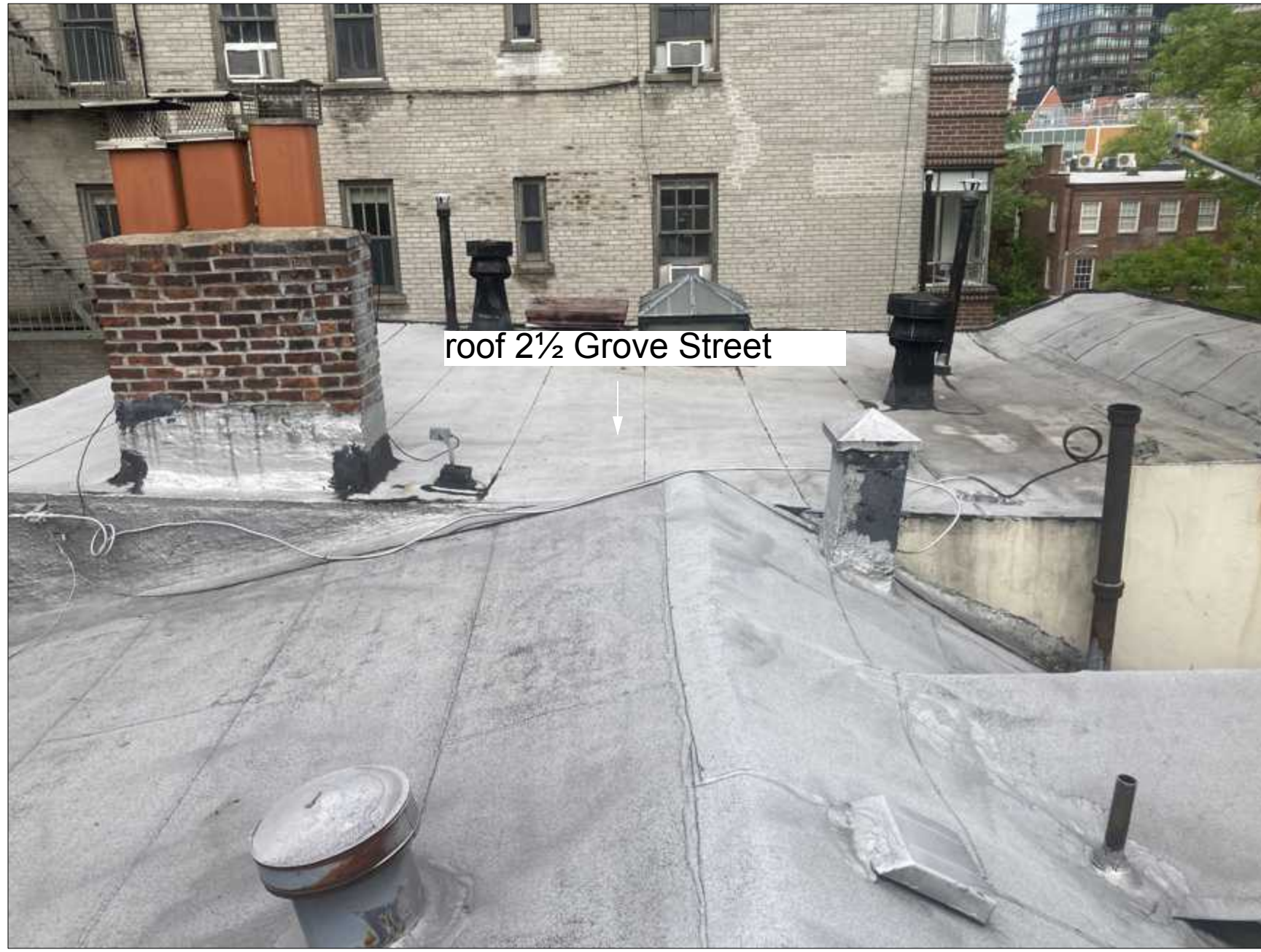
4 grove street - existing roof west
