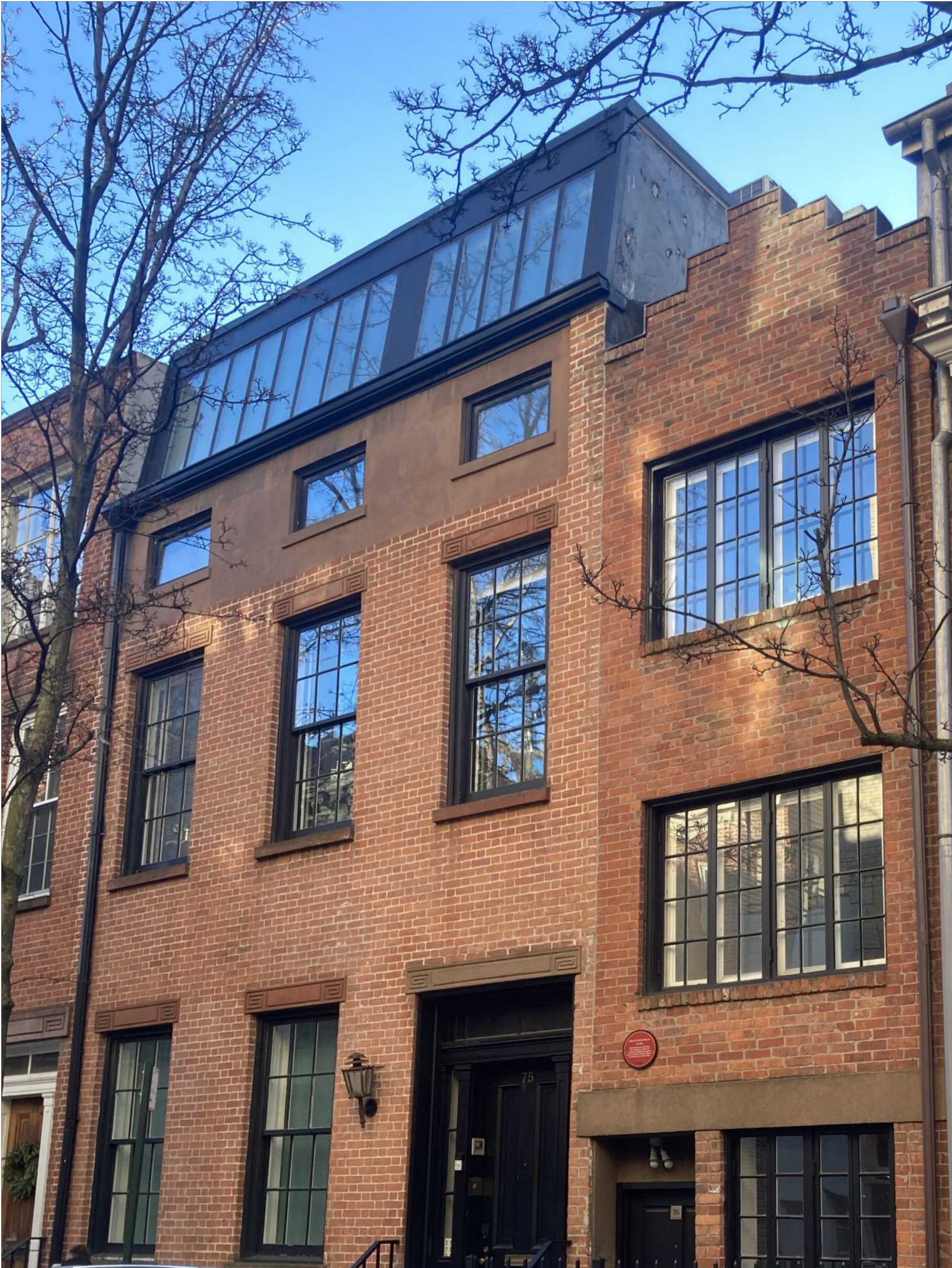
75 bedford street 75 bedford was originally constructed c. 1836; the artist/studio dormer/window was originally installed circa or prior to 1940s and rebuilt c. 2014-2016
