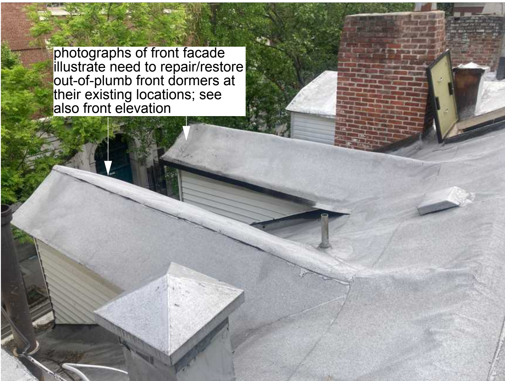
4 grove street - existing roof east
