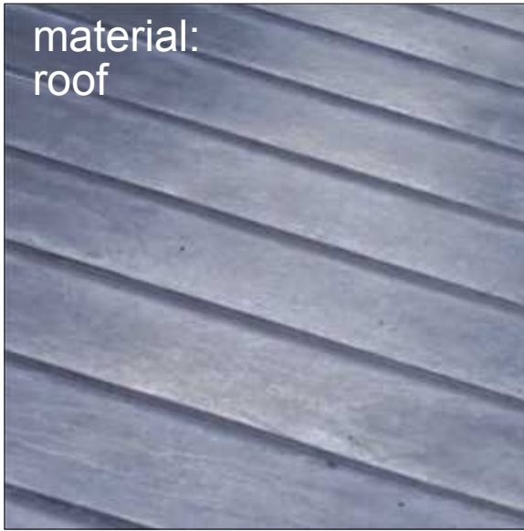
material: roof roofing finish material: lead-coated copper
