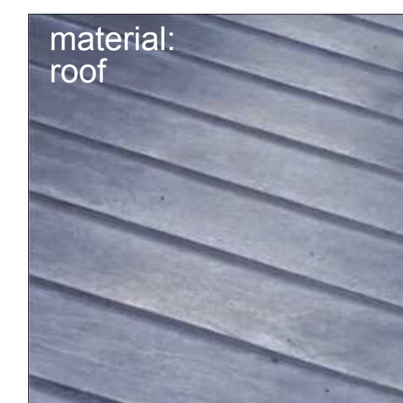
material: roof roofing finish material: lead-coated copper
