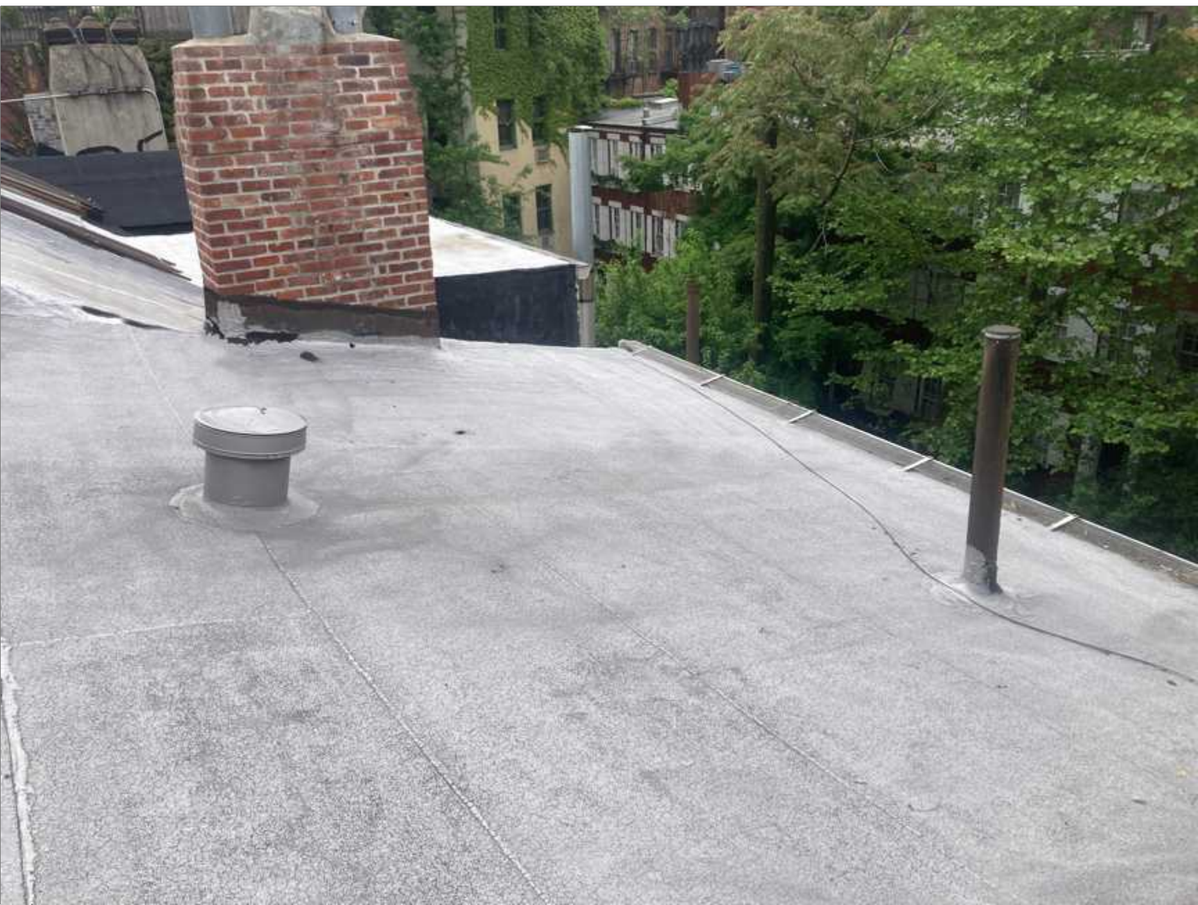
4 grove street - existing roof east
