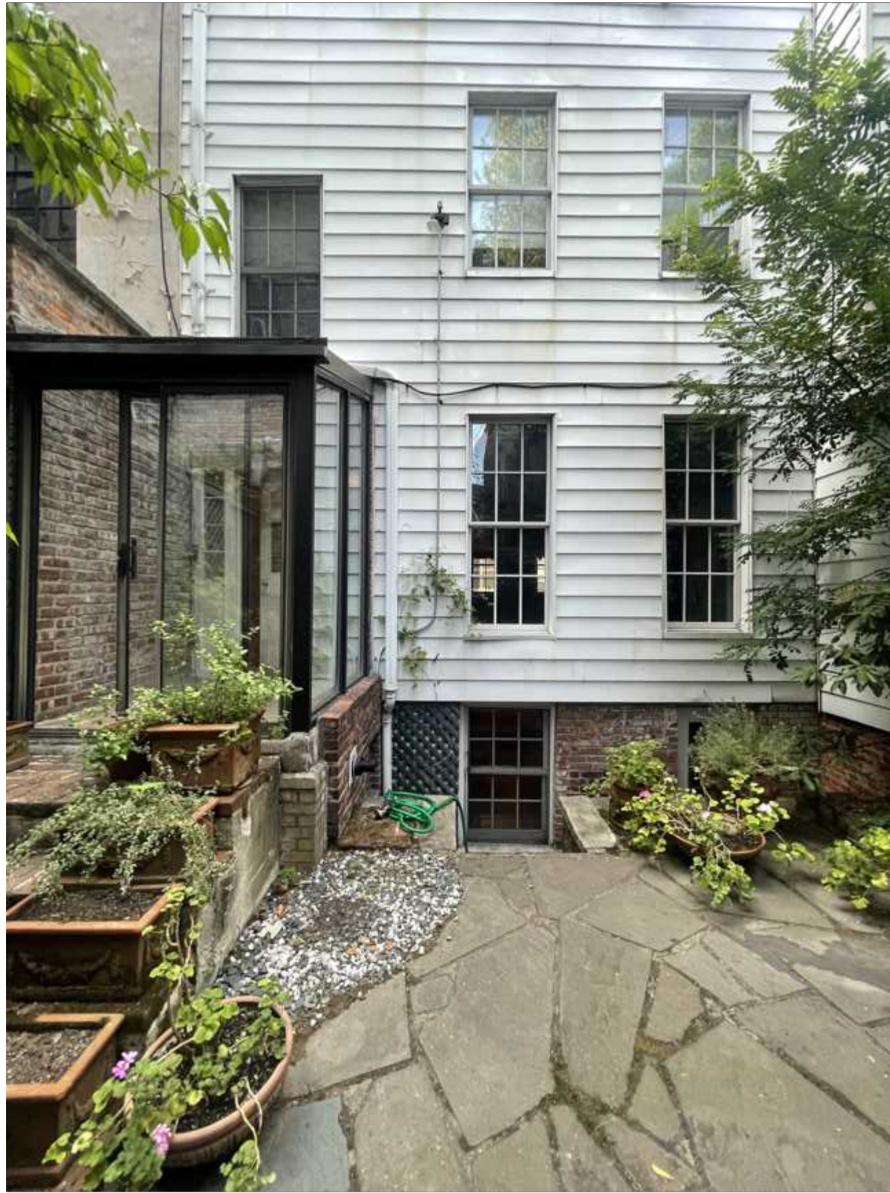
4 grove street - rear facing north
