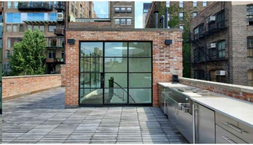
EXISTING ROOF TERRACE LOOKING NORTH AT BULKHEAD SCALE: 1/8" = 1'-0"
