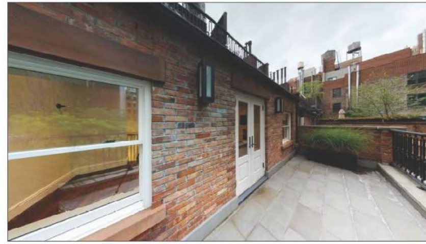
2 EXISTING 4TH FLOOR TERRACE LOOKING WEST LPC-103.00 SCALE: NTS
