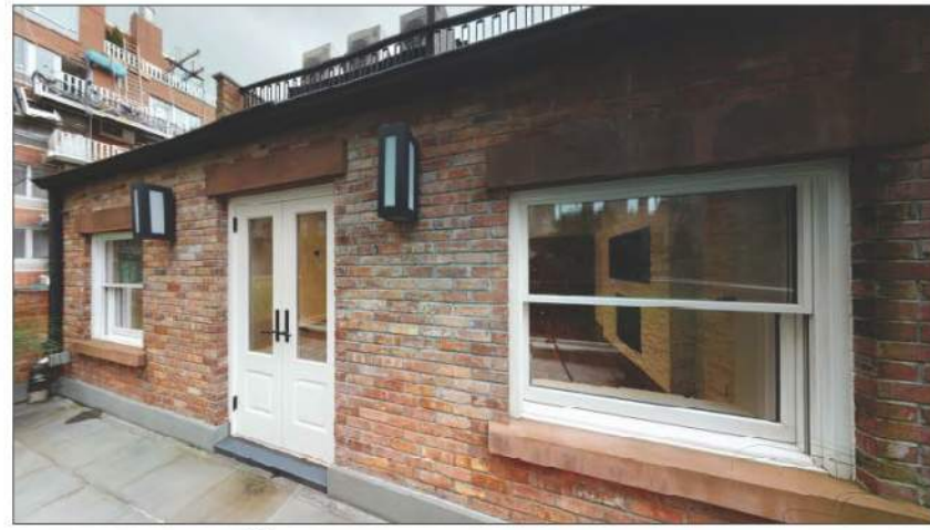
1 EXISTING 4TH FLOOR TERRACE LOOKING EAST LPC-103.00 SCALE: NTS
