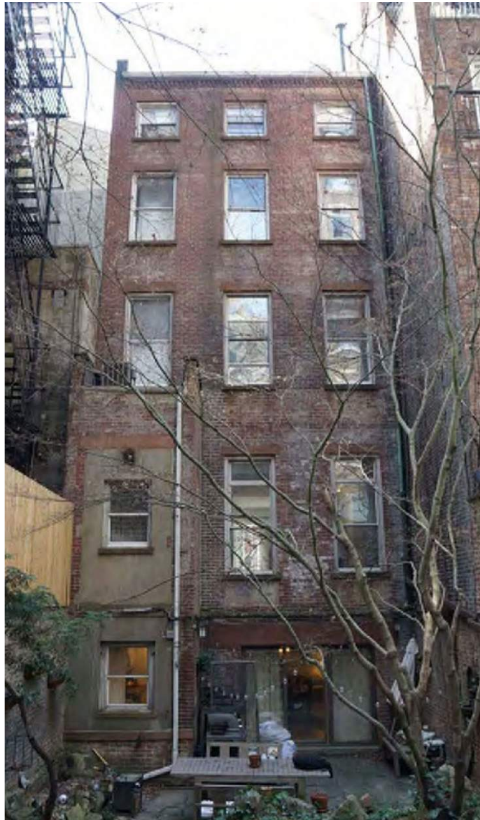
NEIGHBOR - 29 E 11 TH ST EXISTING REAR FAÇADE 2020
