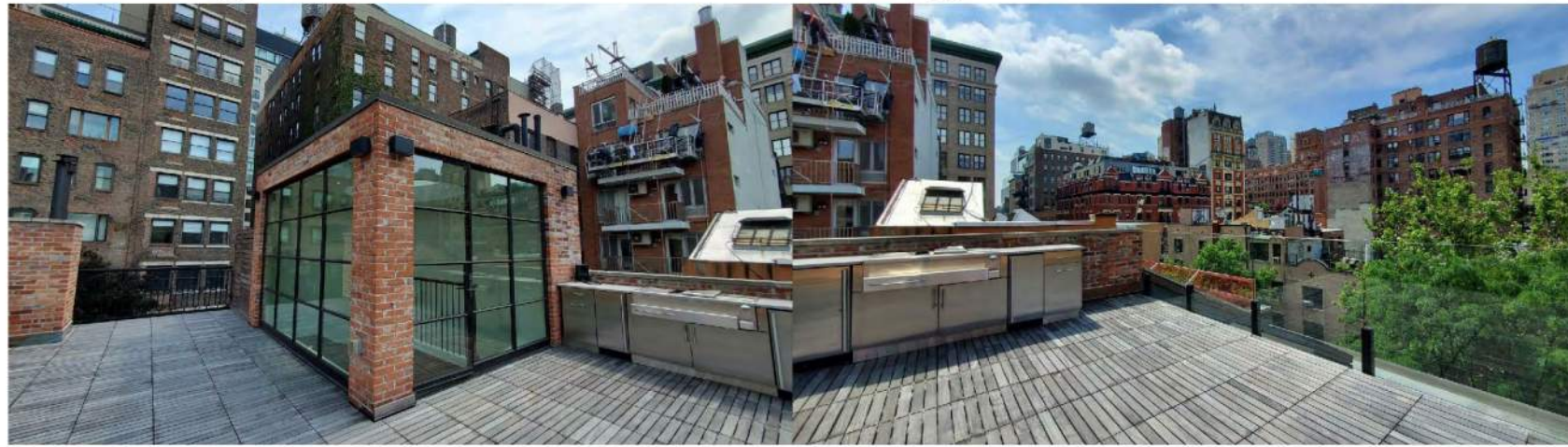
EXISTING ROOF TERRACE LOOKING NORTH EAST AT BULKHEAD SCALE: 1/8" = 1'-0"
