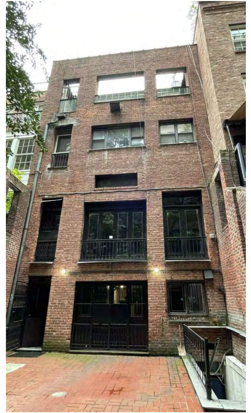
NEIGHBOR - 25 E 11 TH ST EXISTING REAR FAÇADE 2022
