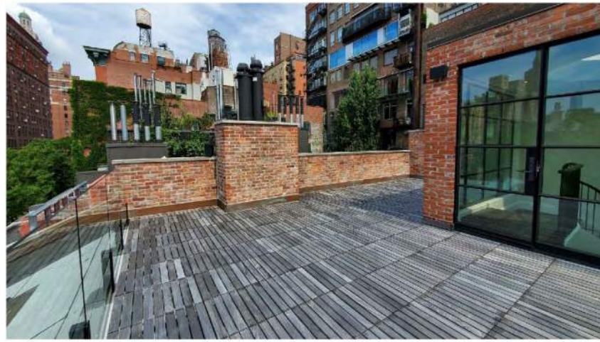
EXISTING ROOF TERRACE LOOKING WEST SCALE: 1/8" = 1'-0"
