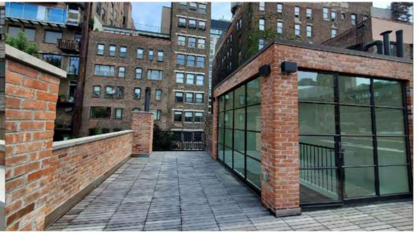
EXISTING ROOF TERRACE LOOKING NORTH SCALE: 1/8" = 1'-0"
