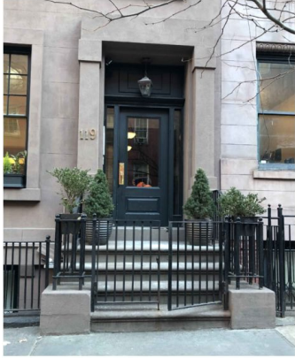
01 119 WAVERLY PLACE FRONT GATE AND FENCE
