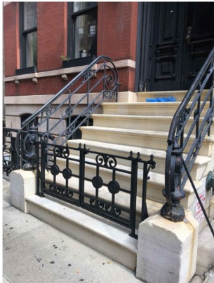
04 133 W Forth Street FRONT GATE
