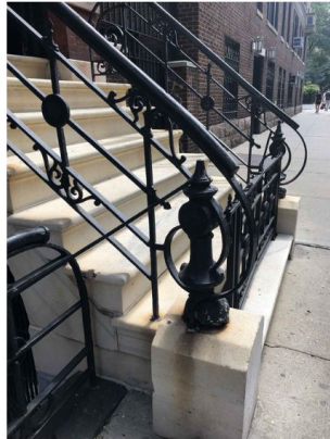
05 133 W Forth Street FRONT GATE
