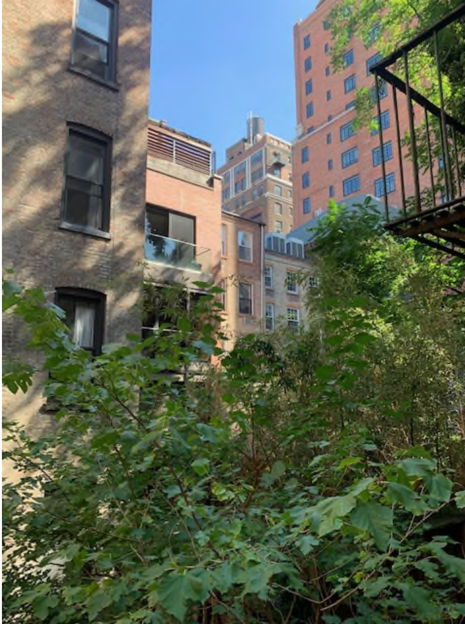
Sixth Avenue Building
