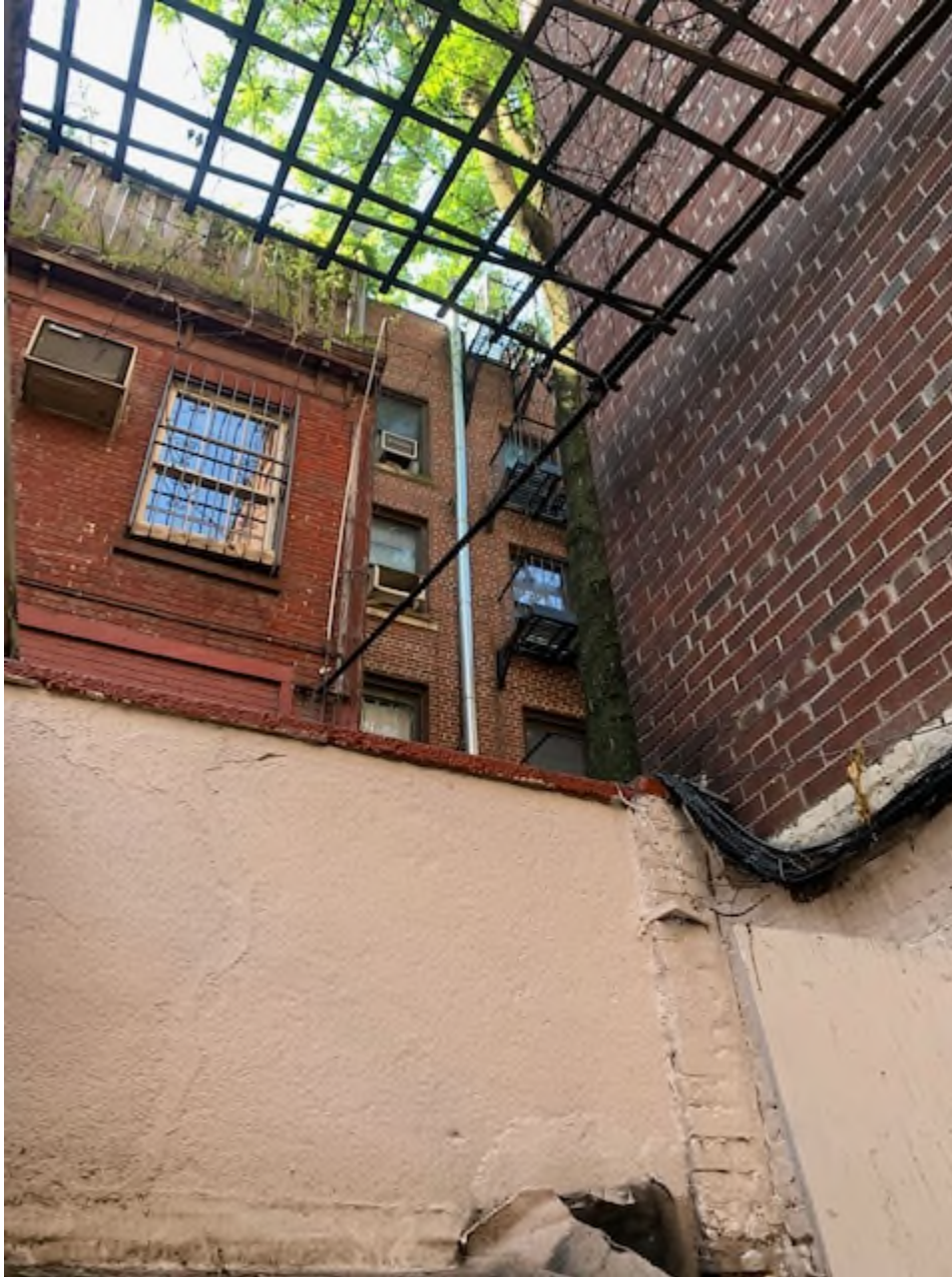
Back of 147 West 4 th Street
