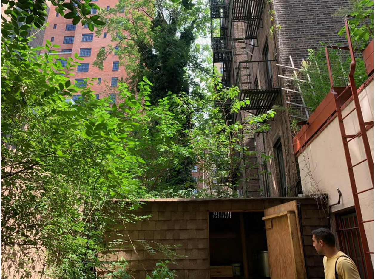
Back of 145 West 4 th Street
