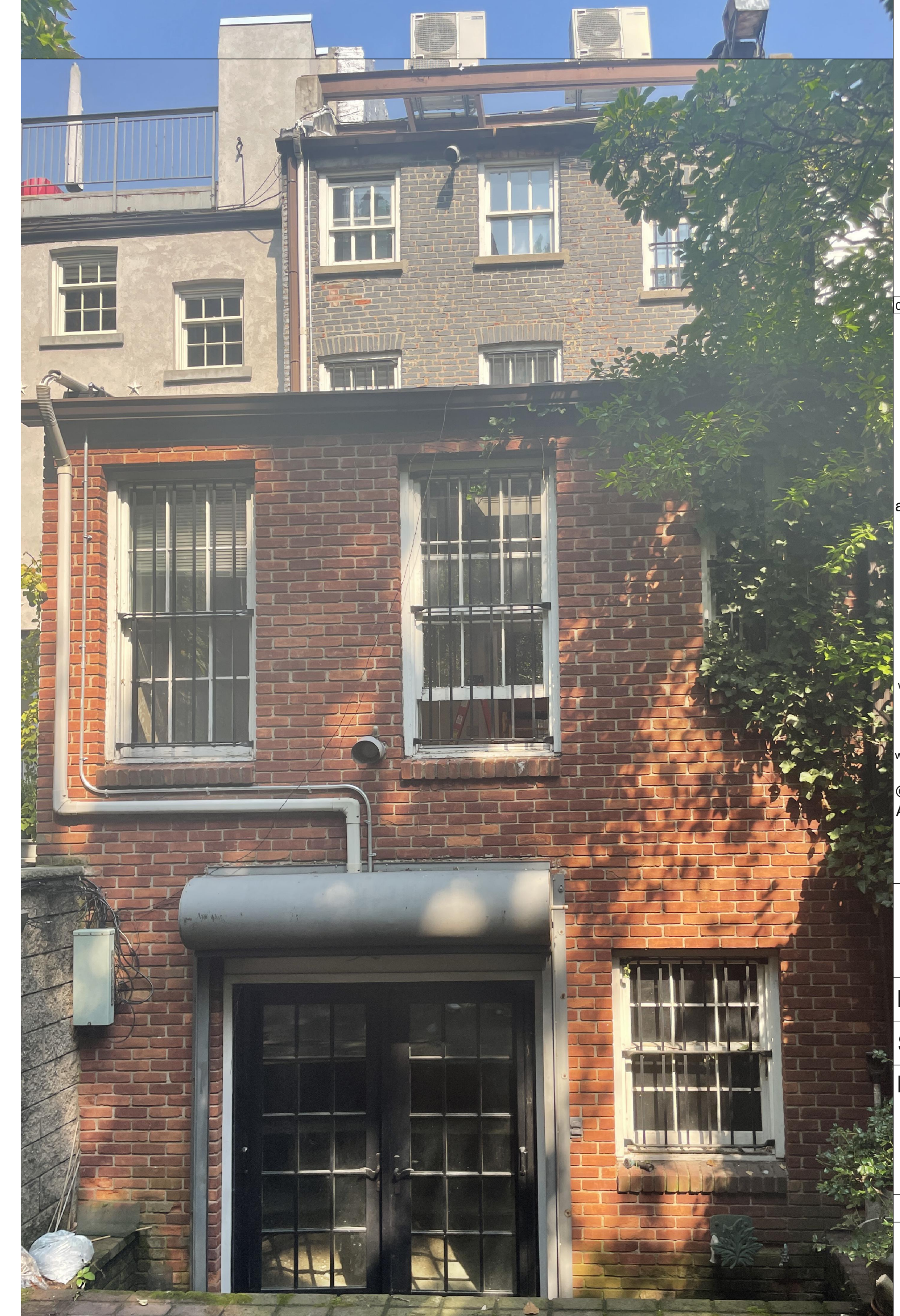
7 ENLARGED EXISTING REAR ELEVATION PHOTO
