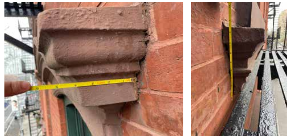
Existing Stone Header and Sill Profiles
