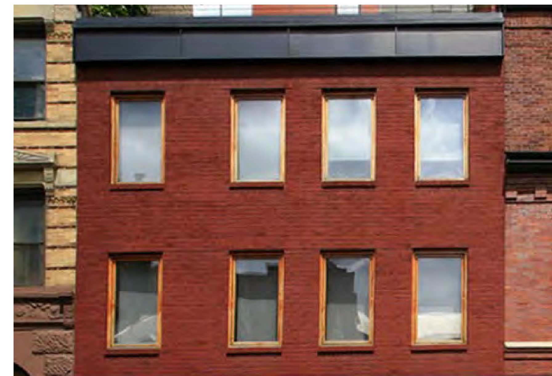
13 LEROY STREET - FULL-PANE WINDOW
