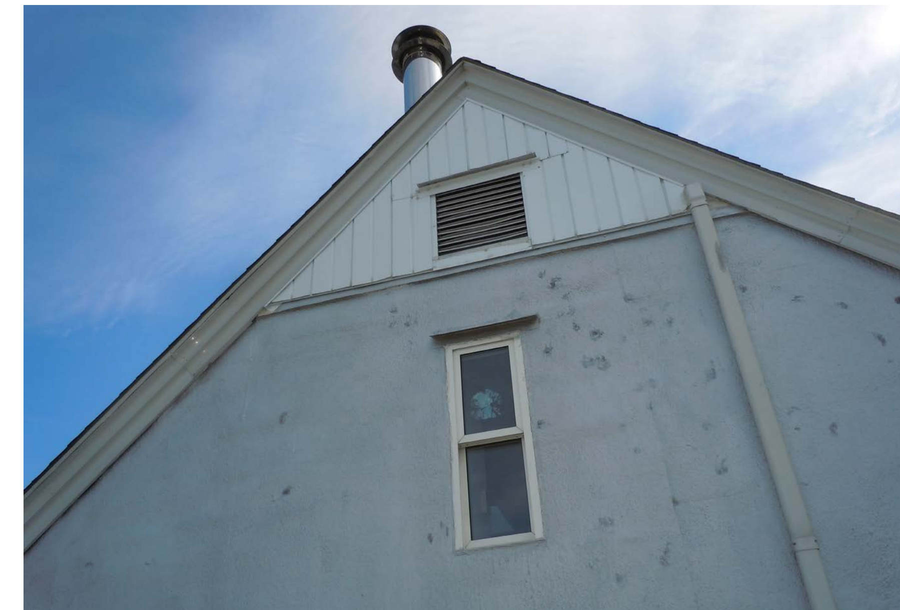
EXISTING ROOFTOP PENTHOUSE - REAR
