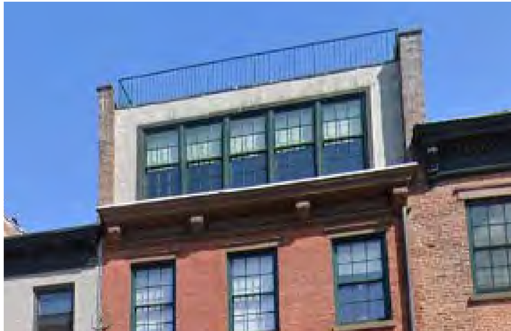
444 6TH AVENUE, 1844 BUILT, ROOFTOP ADDITION LEGALIZED POST-LANDMARK DESIGNATION (1969) IN 2015
