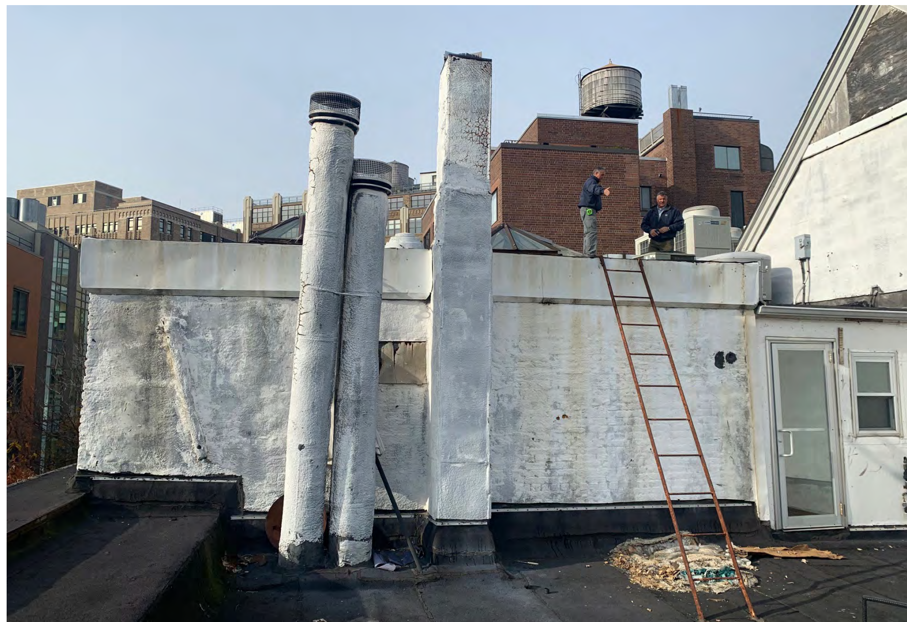
EXISTING ROOFTOP BULKHEAD
