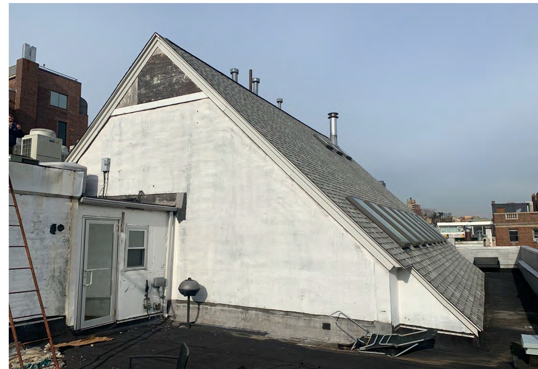
EXISTING ROOFTOP BULKHEAD AND PENTHOUSE - FRONT
