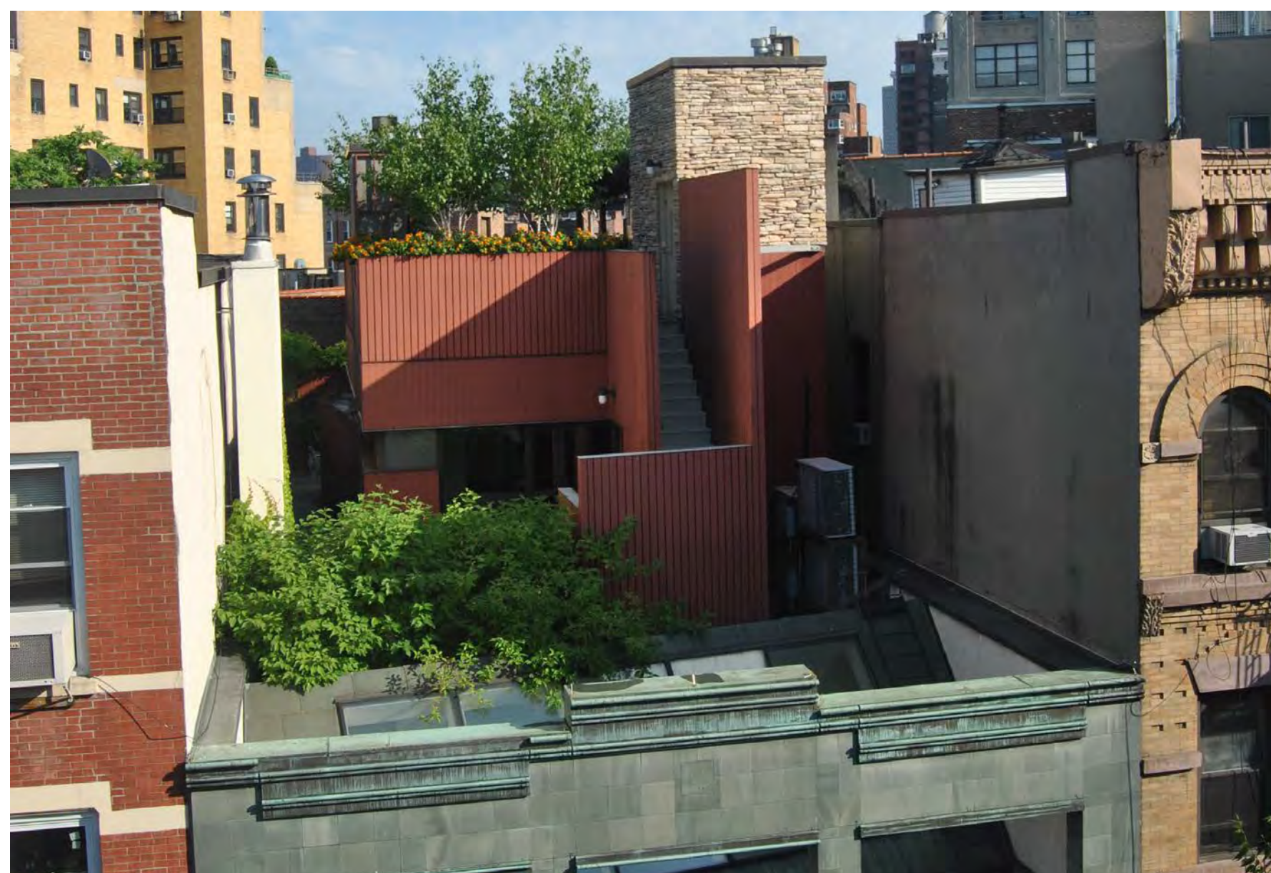
42 DOWNING STREET - ONE-STORY ROOFTOP ADDITION WITH BULKHEAD
