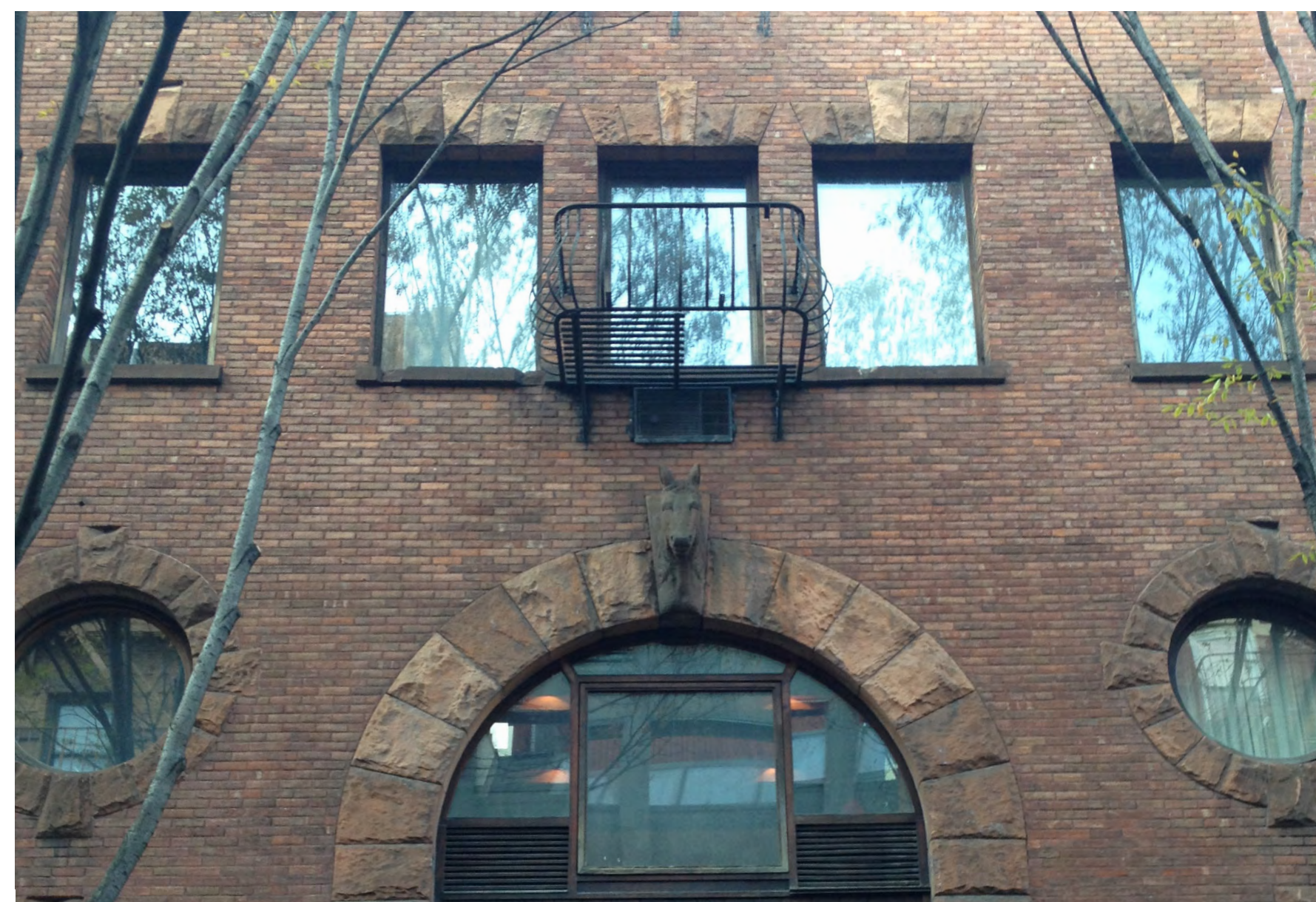
51 DOWNING STREET - 3RD FLOOR WINDOWS
