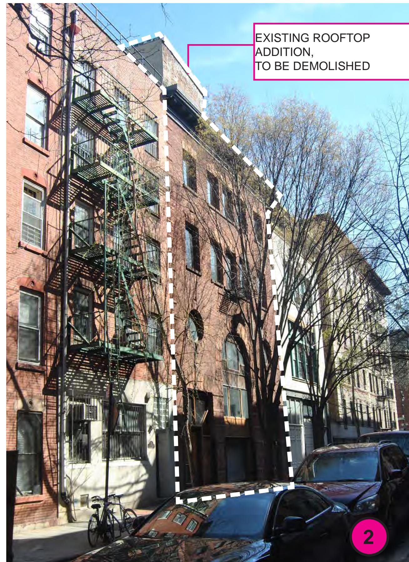
VIEW 2: DOWNING STREET LOOKING EAST - EXISTING VIEW
