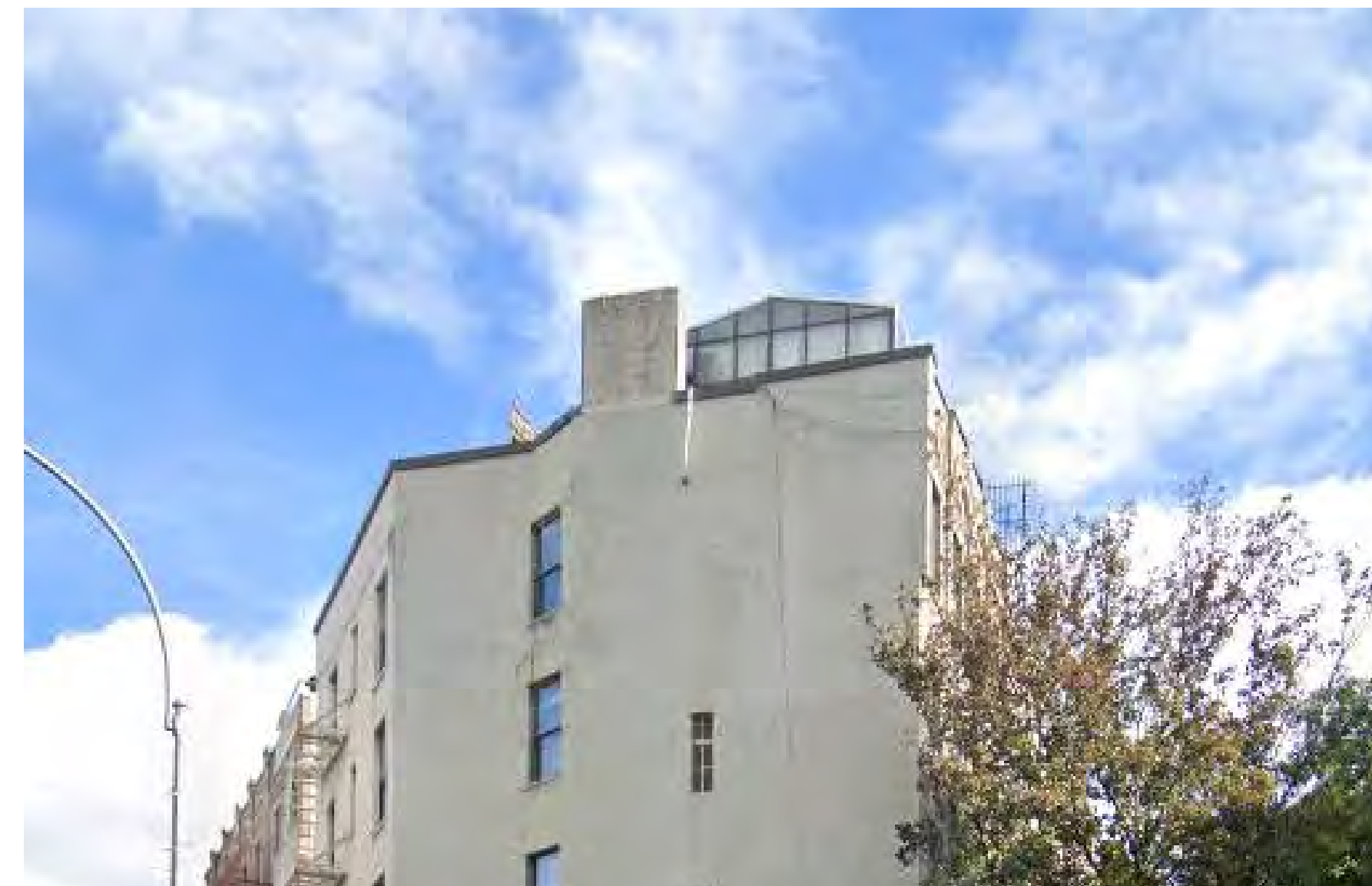
47 7TH AVENUE SOUTH, BUILT 1896, ROOFTOP ADDITION ADDED PRE-LANDMARK DESIGNATION (2010)
