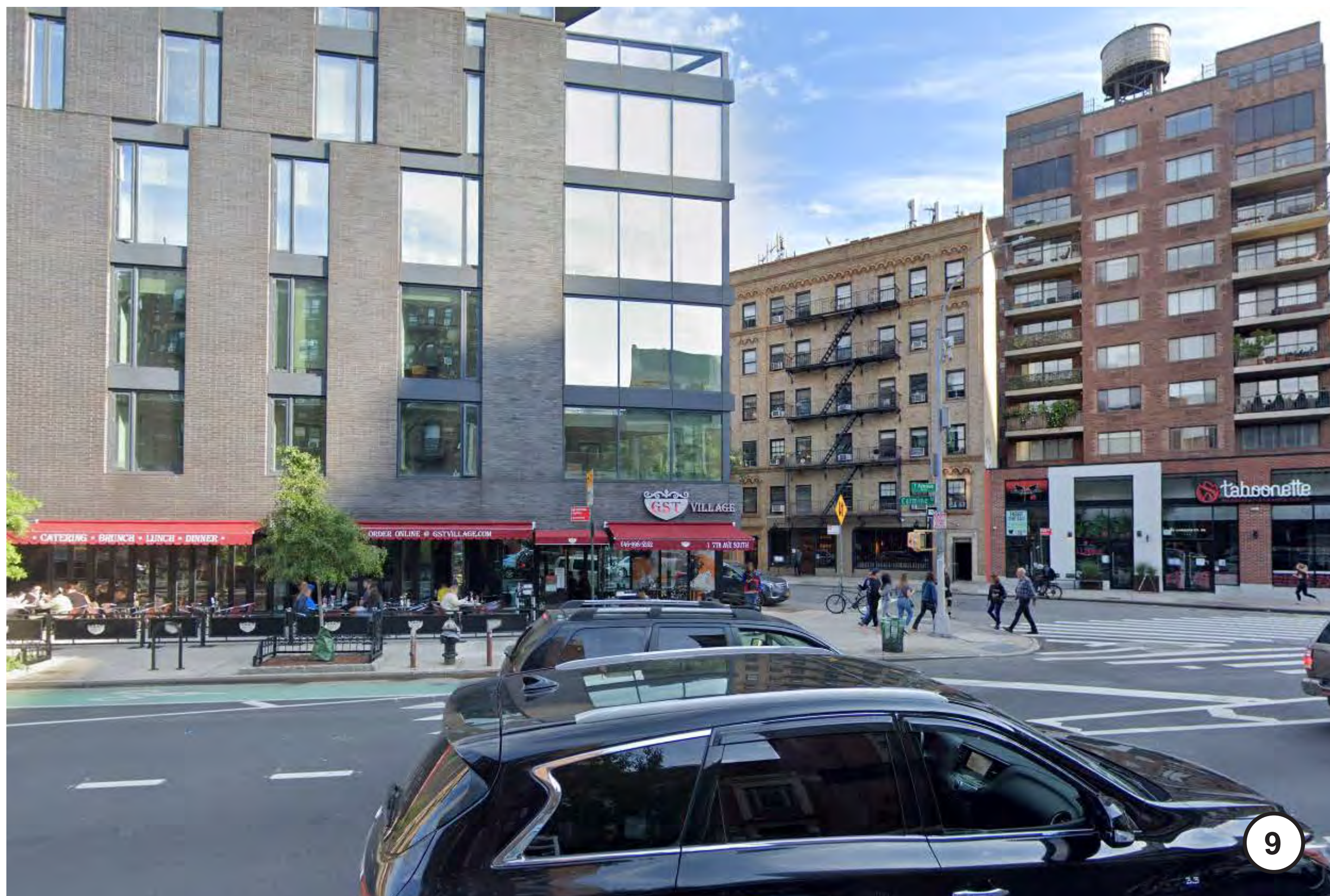
VIEW 9: 7TH AVE X CARMINE STREET LOOKING SE, ROOFTOP ADDITION NOT VISIBLE
