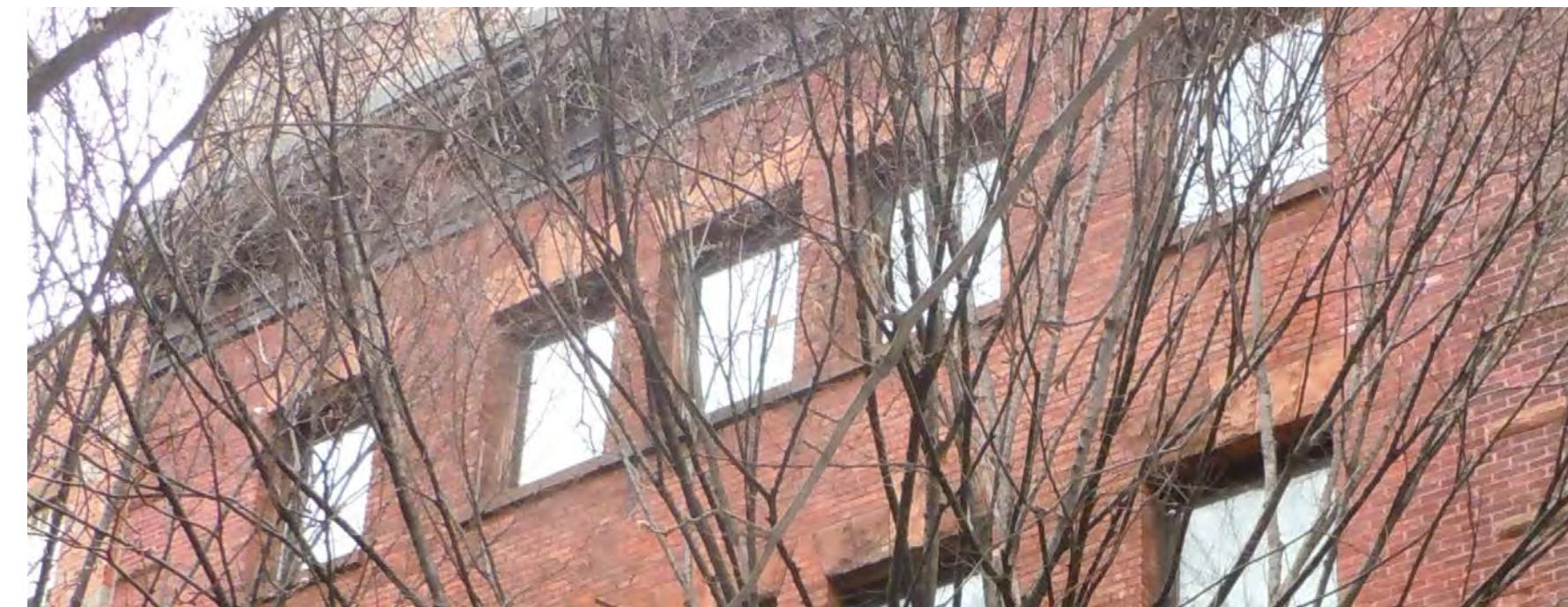
EXISTING 4TH FLOOR WINDOWS
