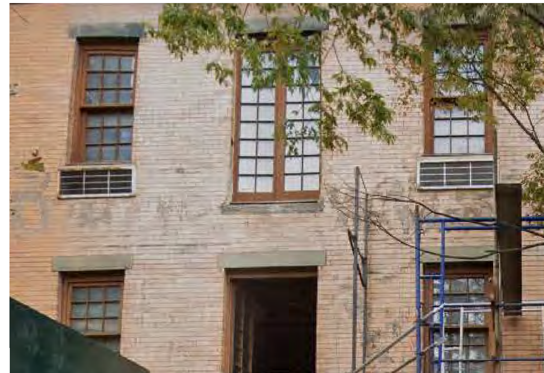
44 PERRY STREET - WOOD FRAME
