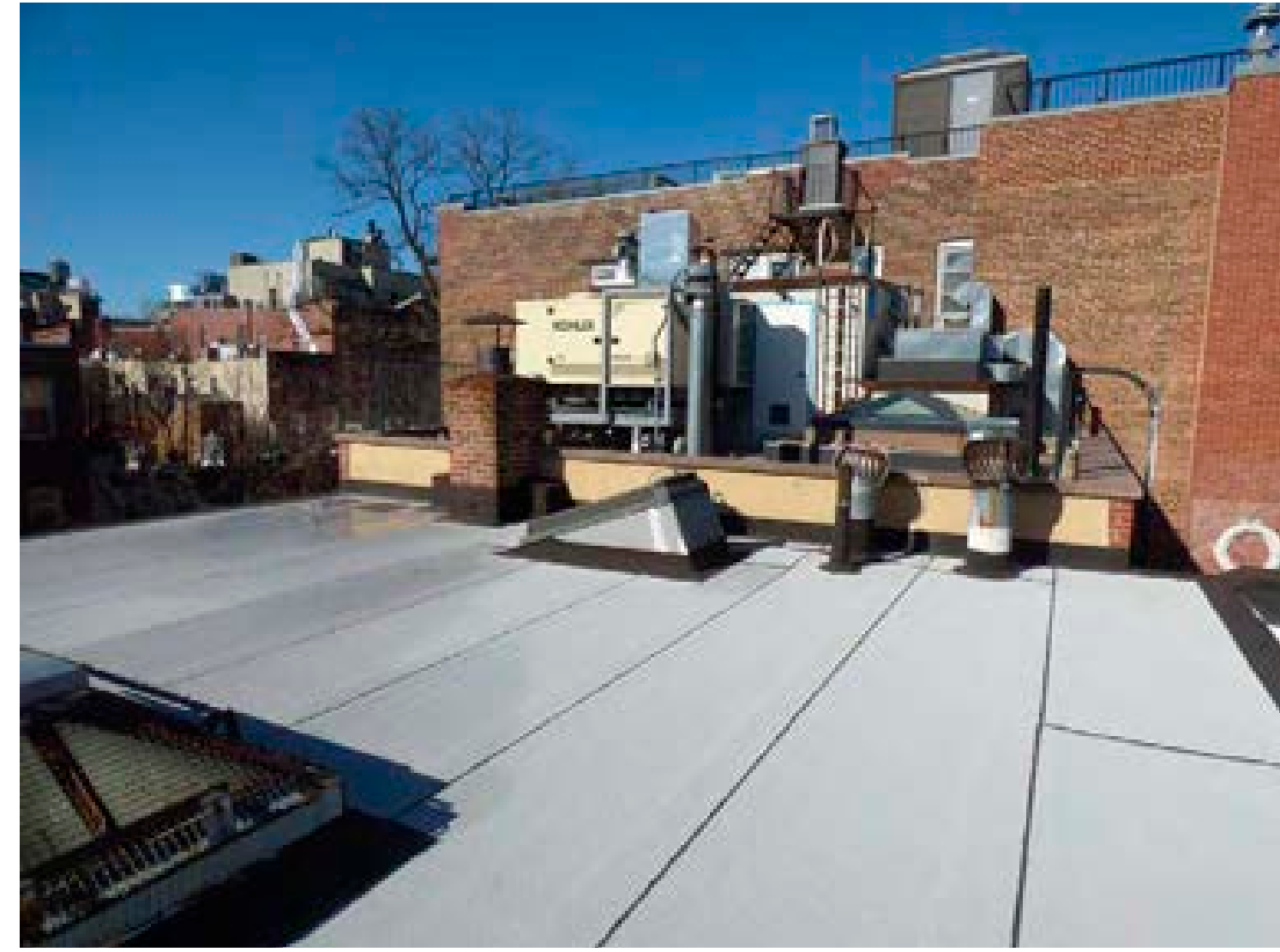
Roof (HQP, 2023), Looking West
