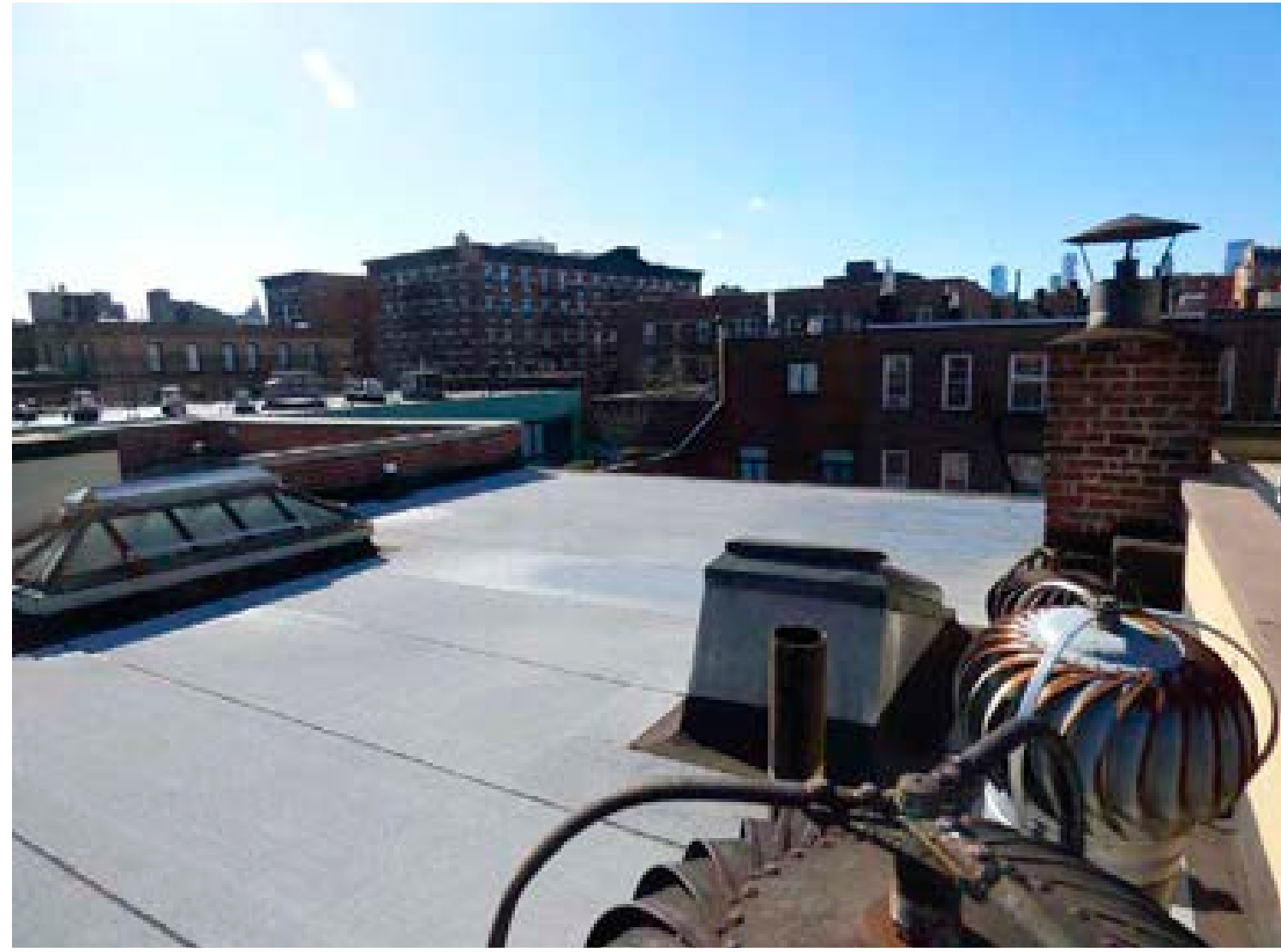
Roof (HQP, 2023), Looking Southeast
