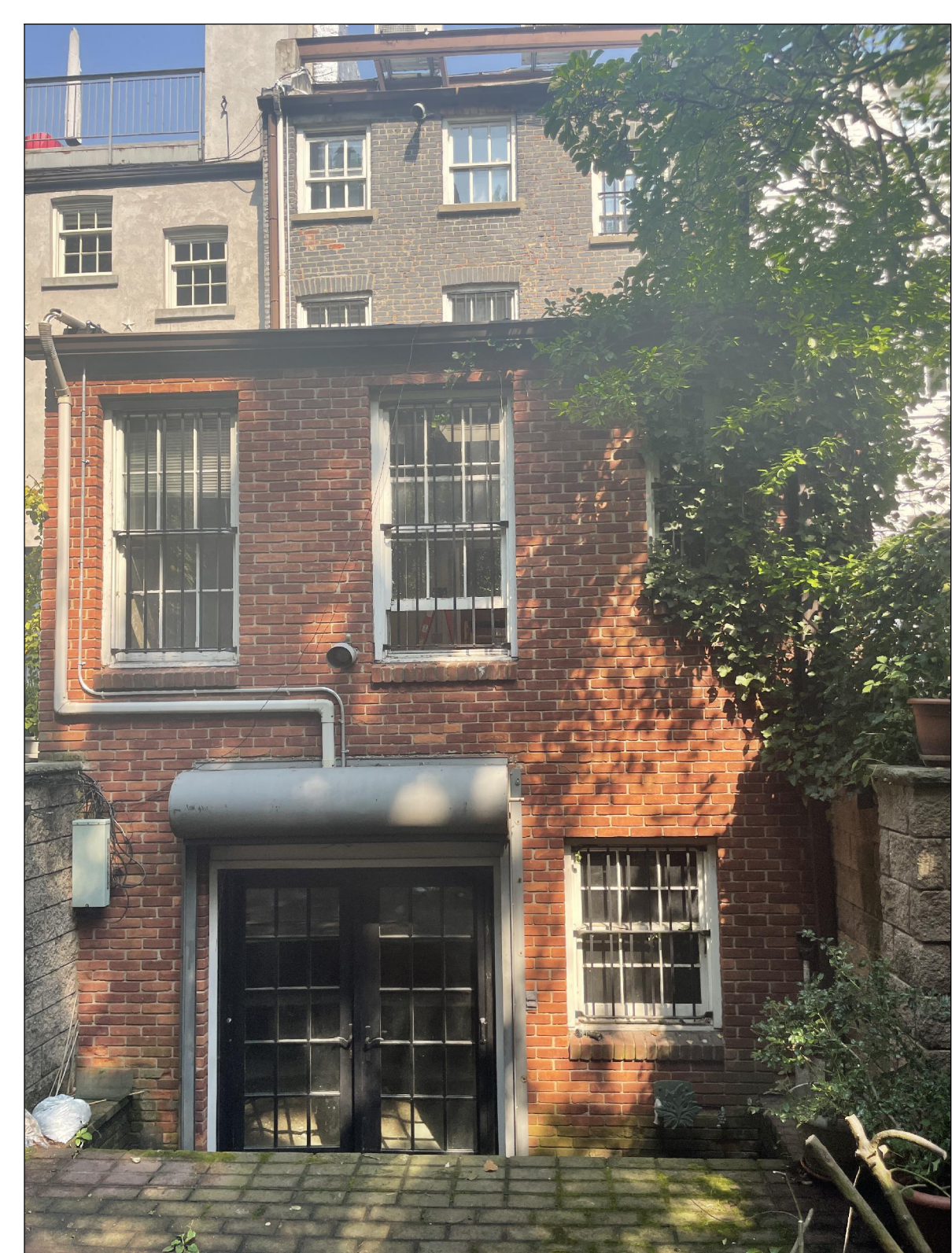
4 130 BANK ST. CURRENT REAR FACADE
