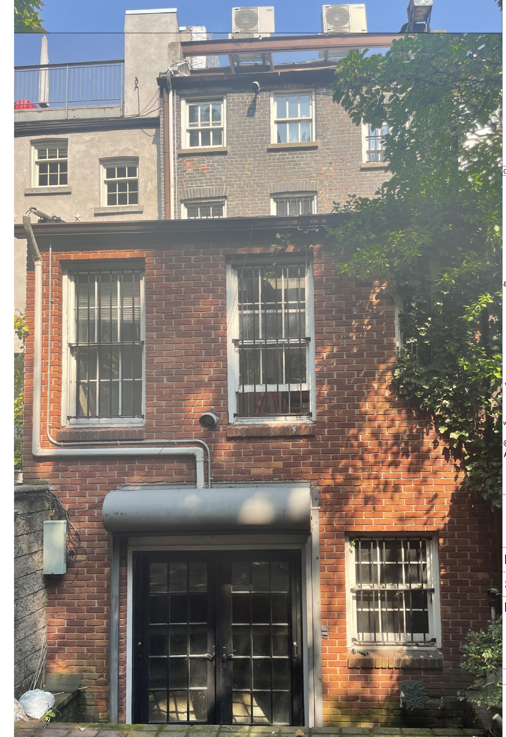
7 ENLARGED EXISTING REAR ELEVATION PHOTO
