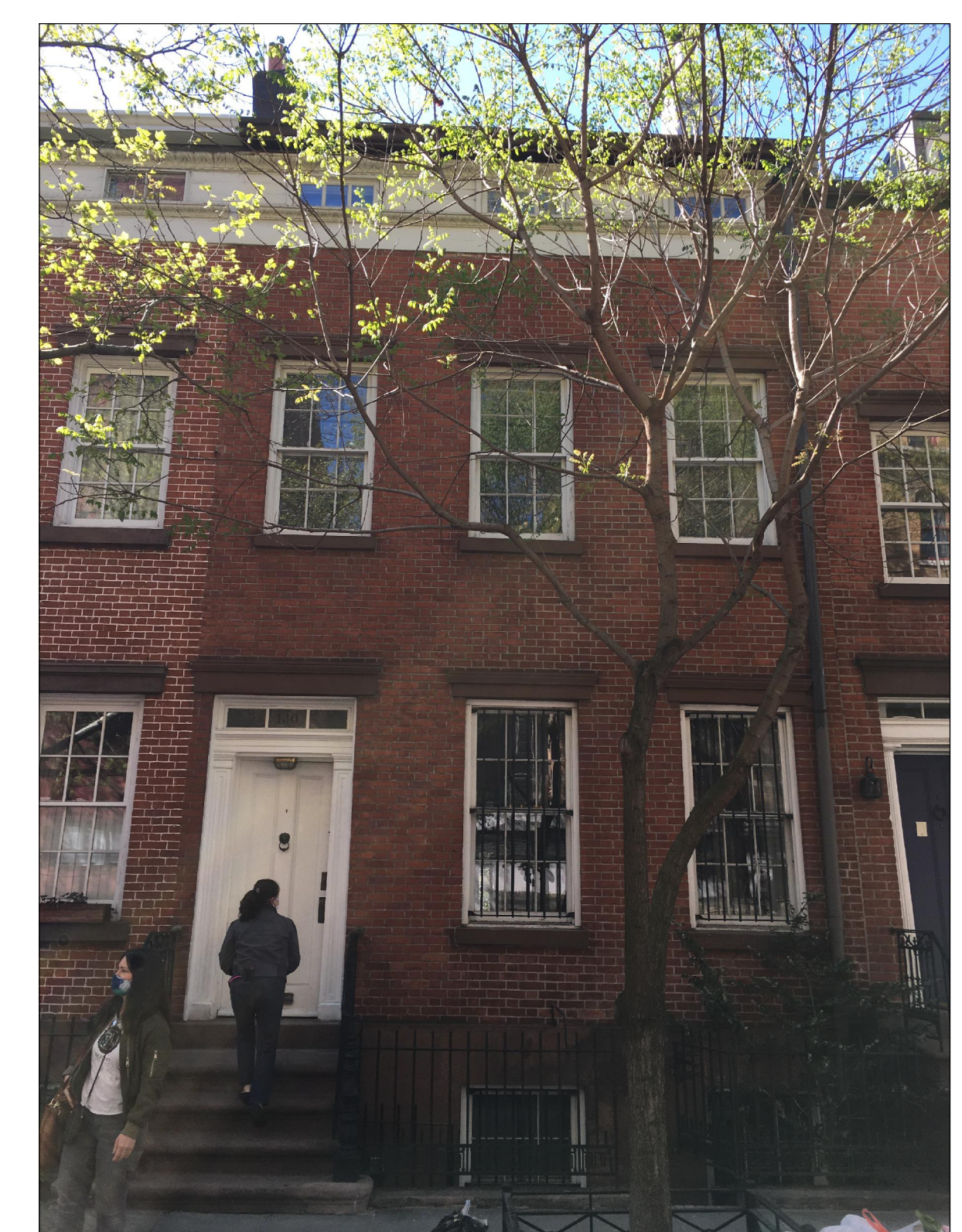
5 130 BANK ST. CURRENT STREET FACADE
