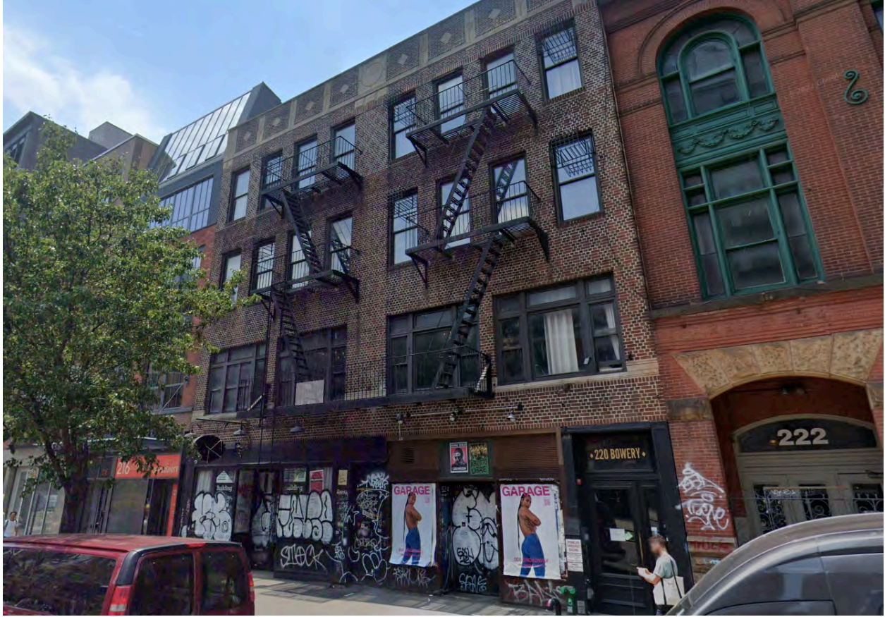
218-220 BOWERY (BEHIND APPLICANT PREMISE) *REFERENCE FOR COURTYARD PHOTO
