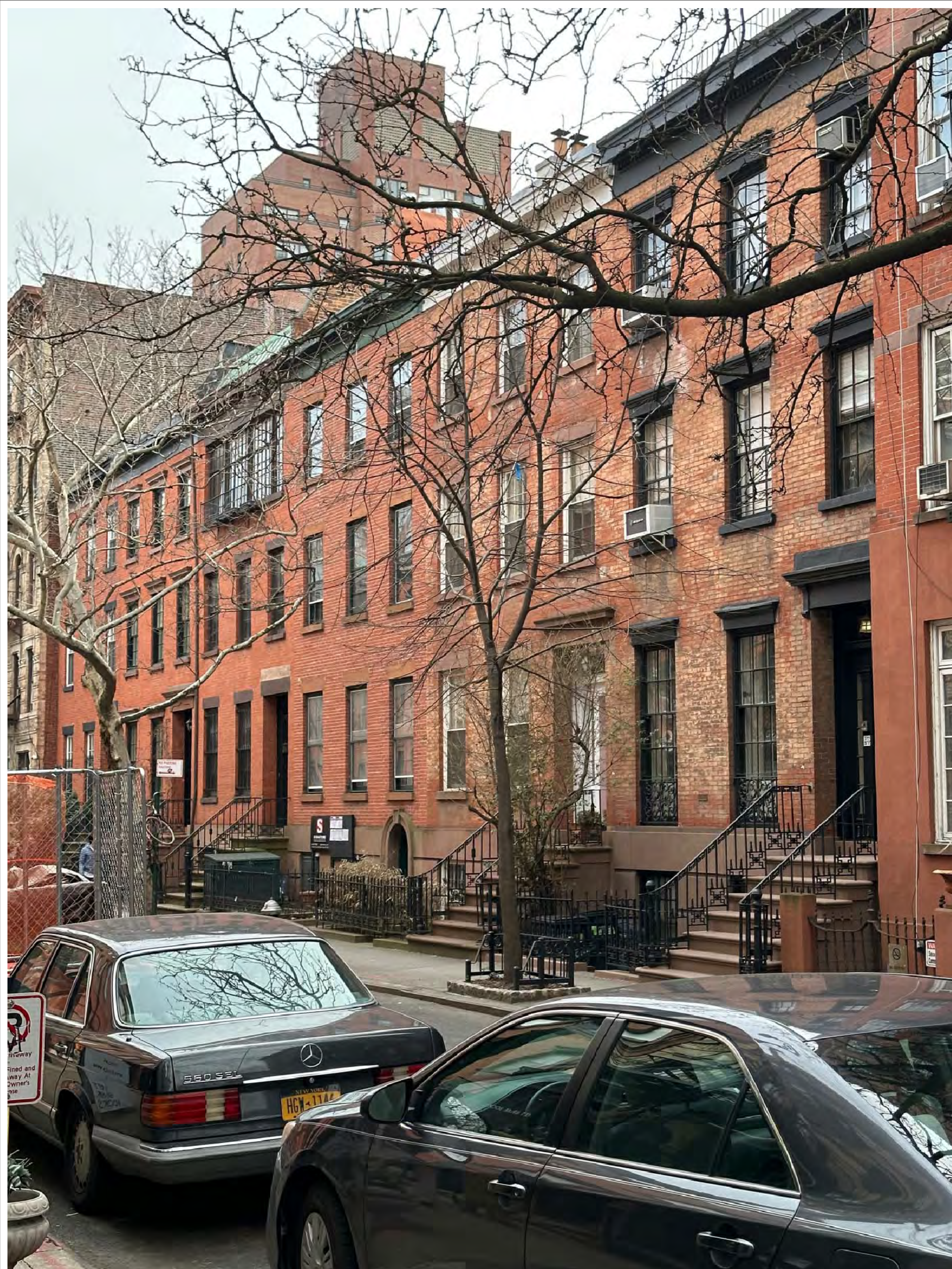
EXISTING CONDITIONS – FRONT ELEVATION LOOKING EAST
