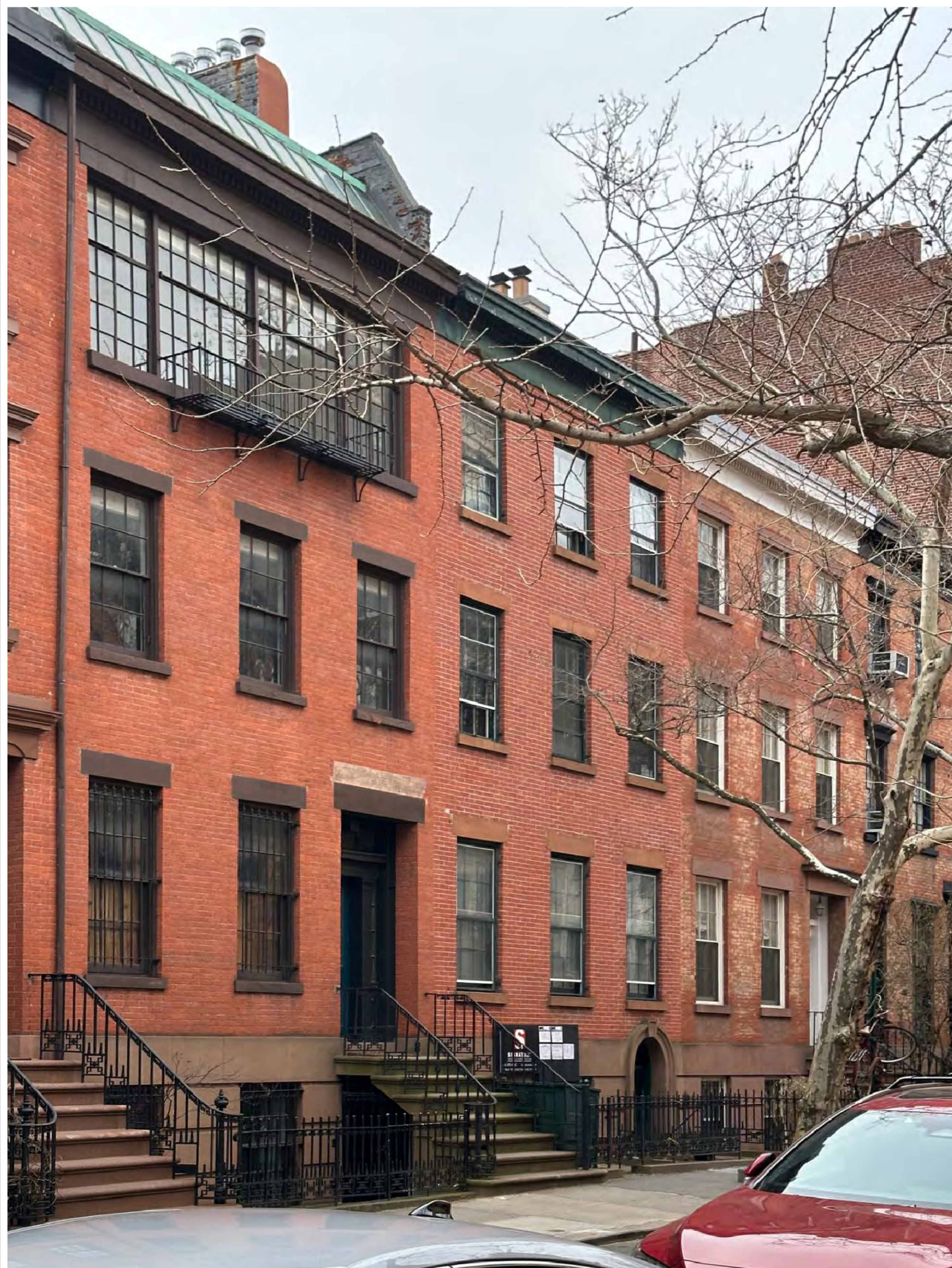
EXISTING CONDITIONS – FRONT ELEVATION LOOKING WEST
