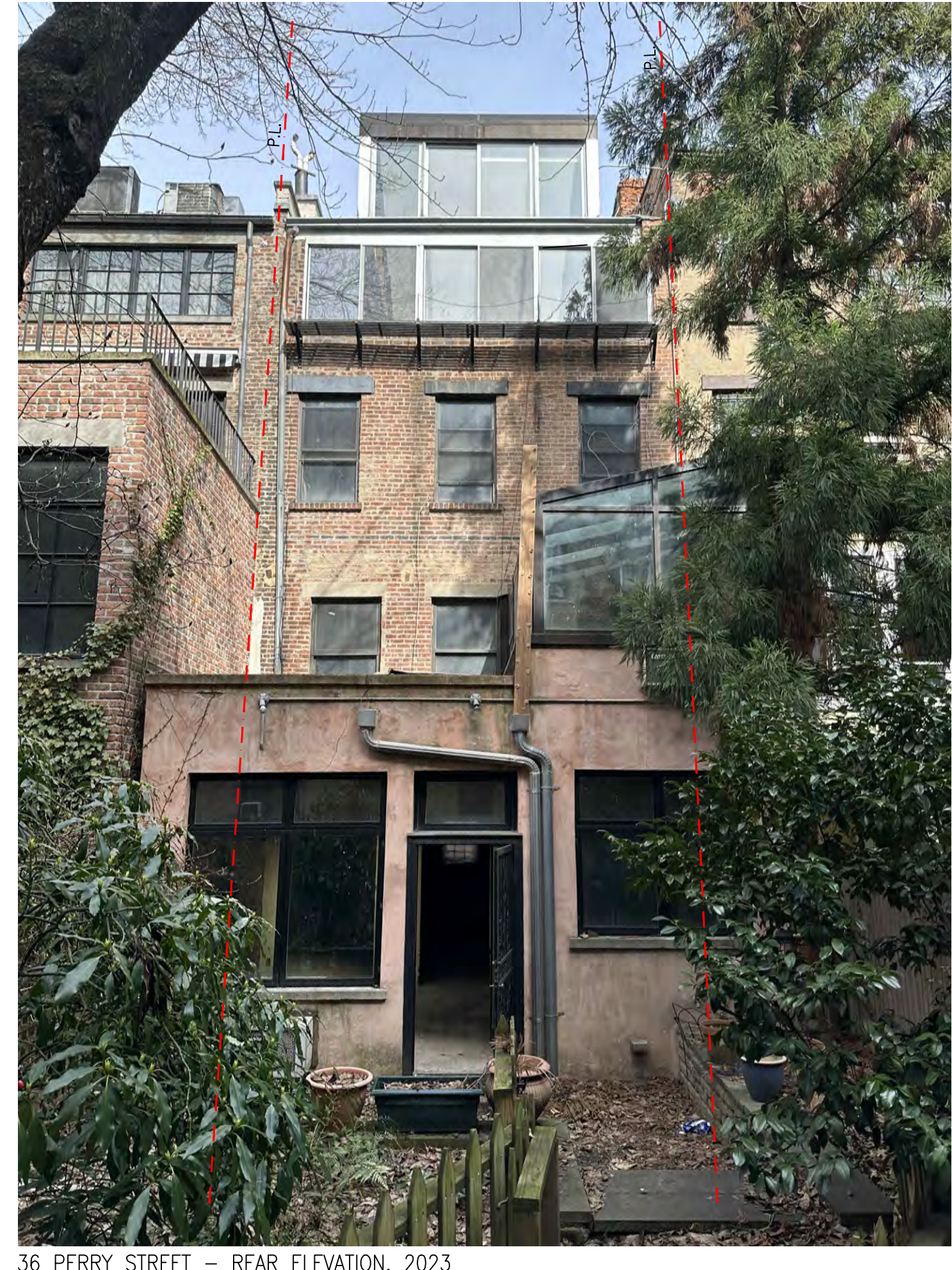
36 PERRY STREET - REAR ELEVATION, 2023
