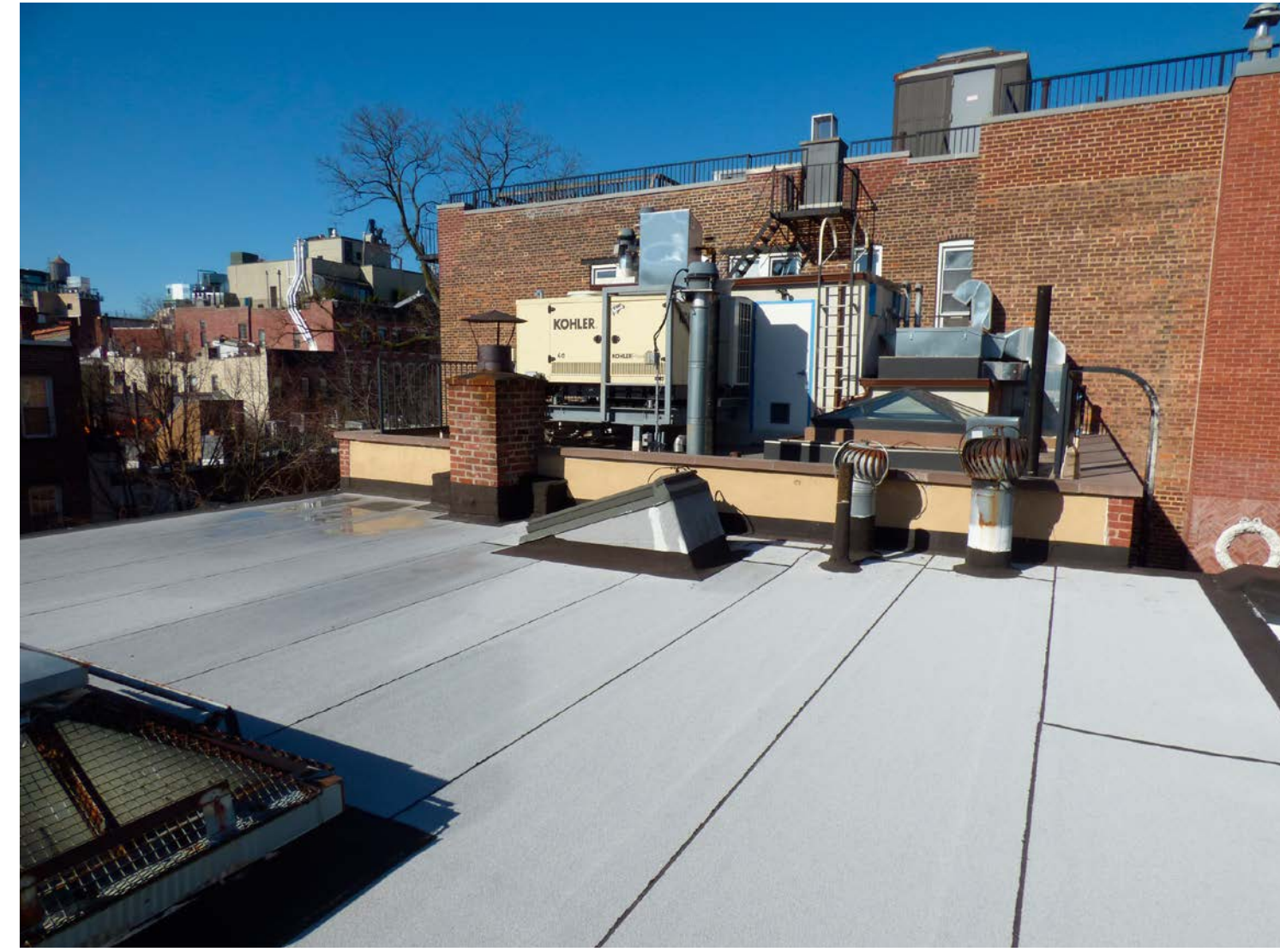
Roof (HQP, 2023), Looking West
