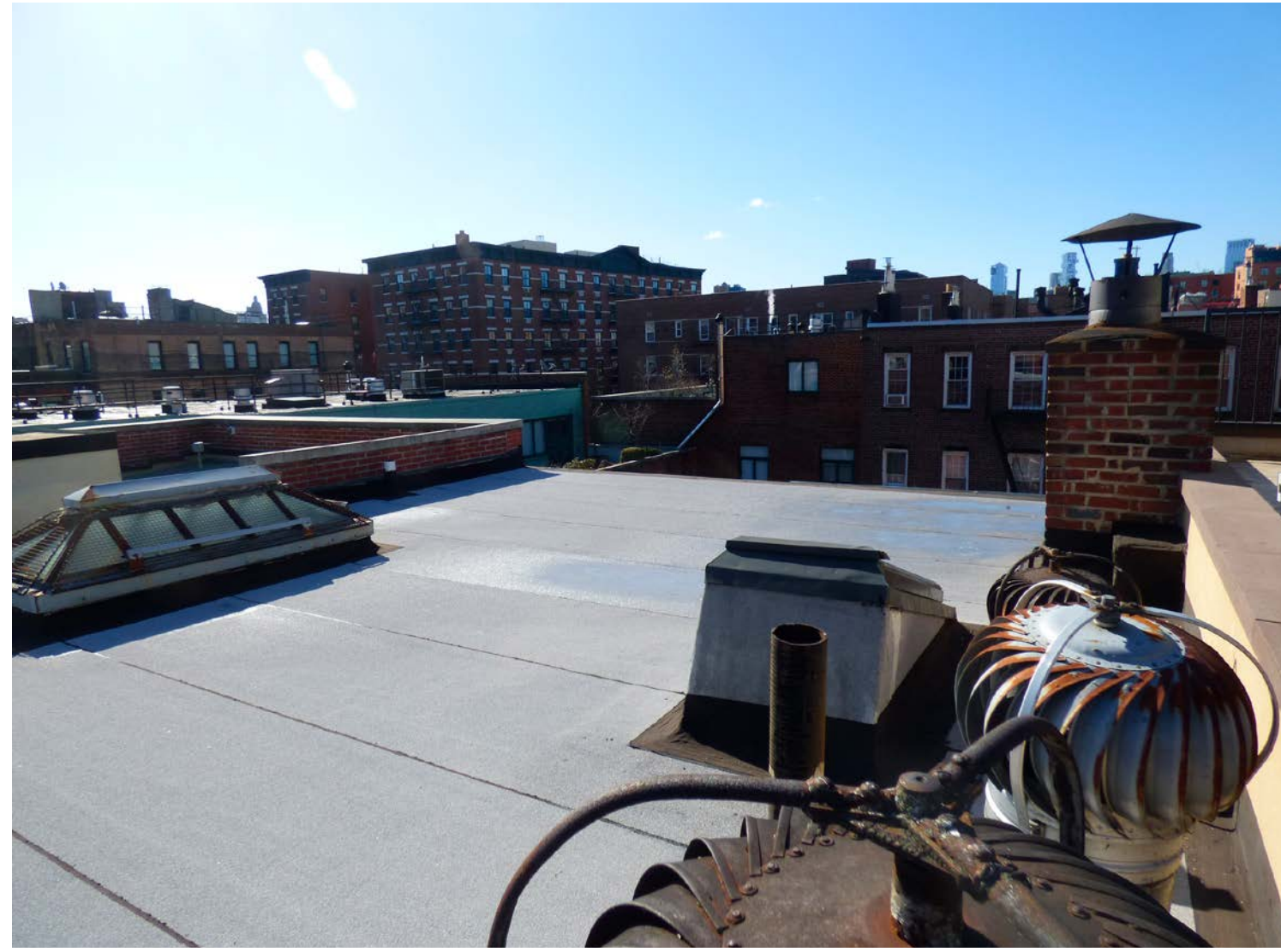
Roof (HQP, 2023), Looking Southeast
