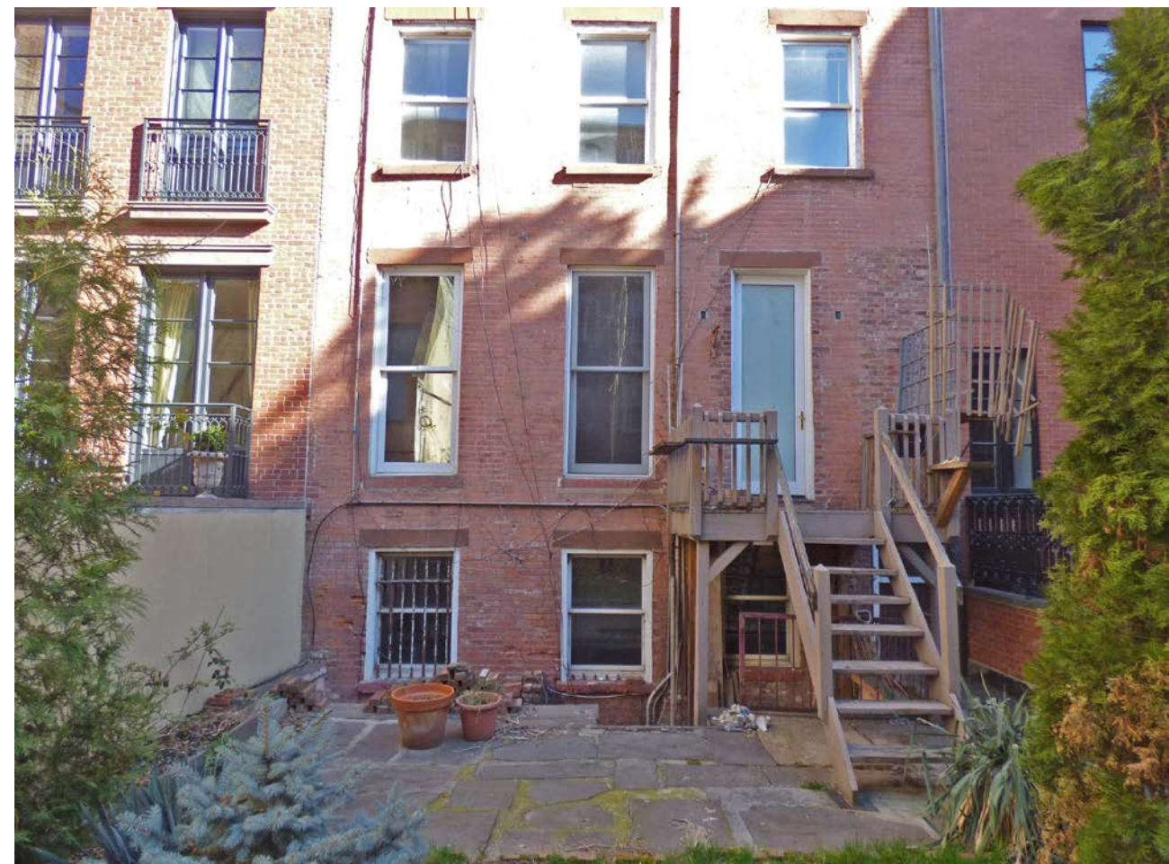
Rear Elevation, Garden Level (HQP, 2023)
