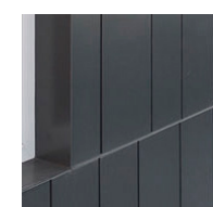
Metal paneled wall to match aluminum framed door system
