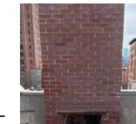
Existing brick chimney
