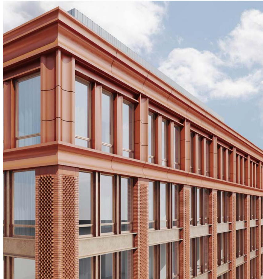
Terracotta Cornice, Framed Metal Spandrels, Framed Column with Terracotta Capital and Base
