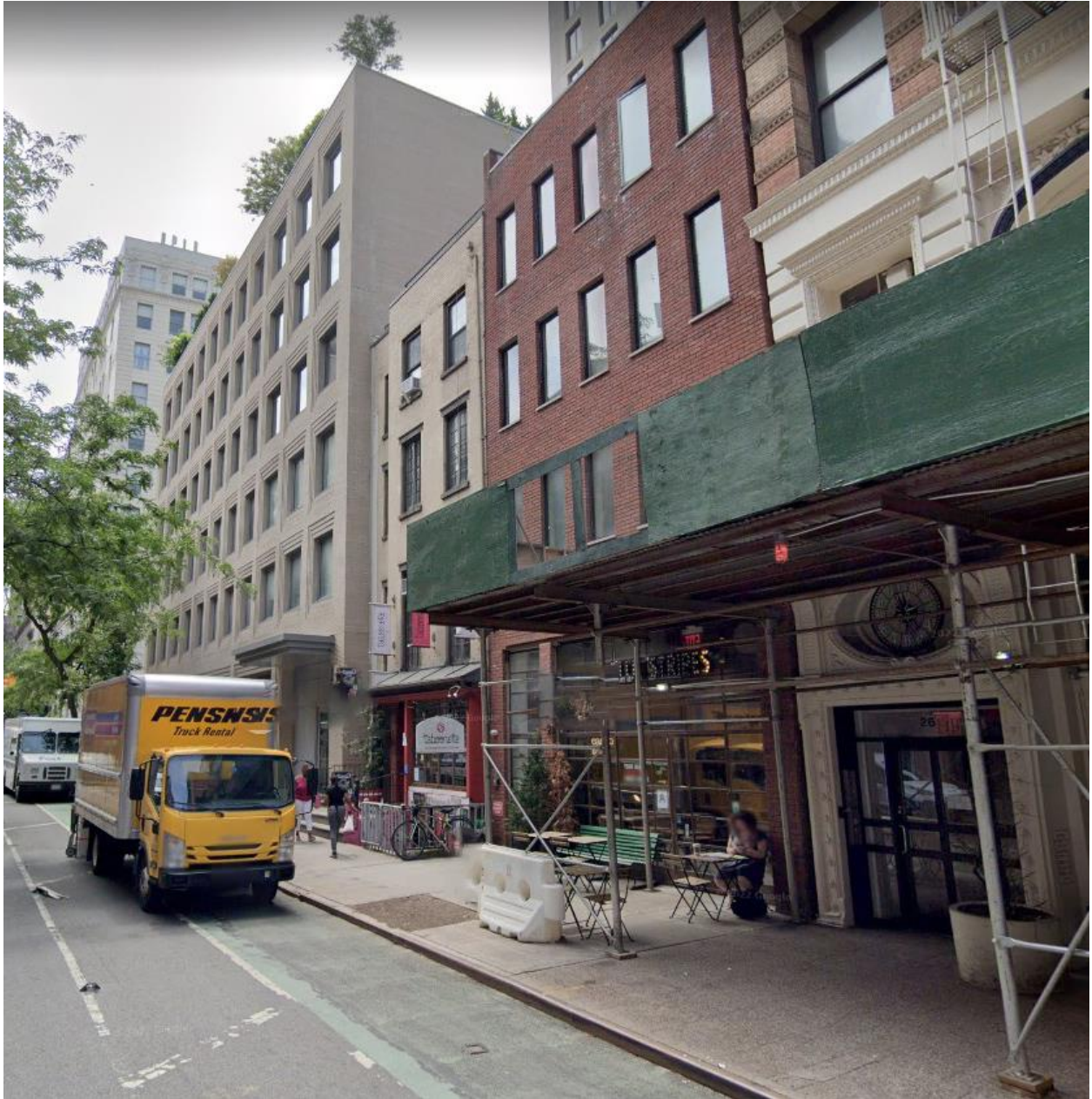
SIDEWALK VIEW AND ENTRANCE
