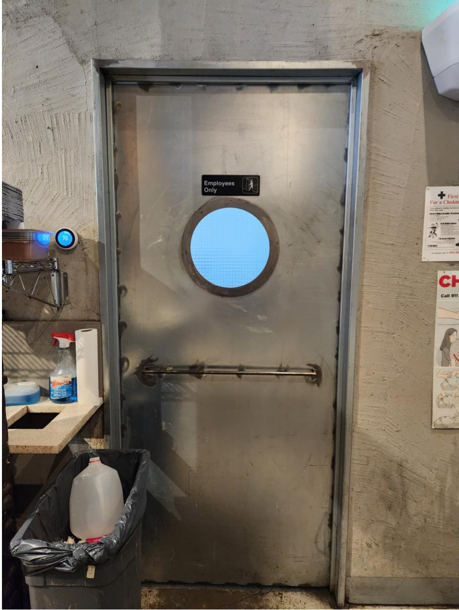
ACCESS TO THE BASEMENT STAIRS
