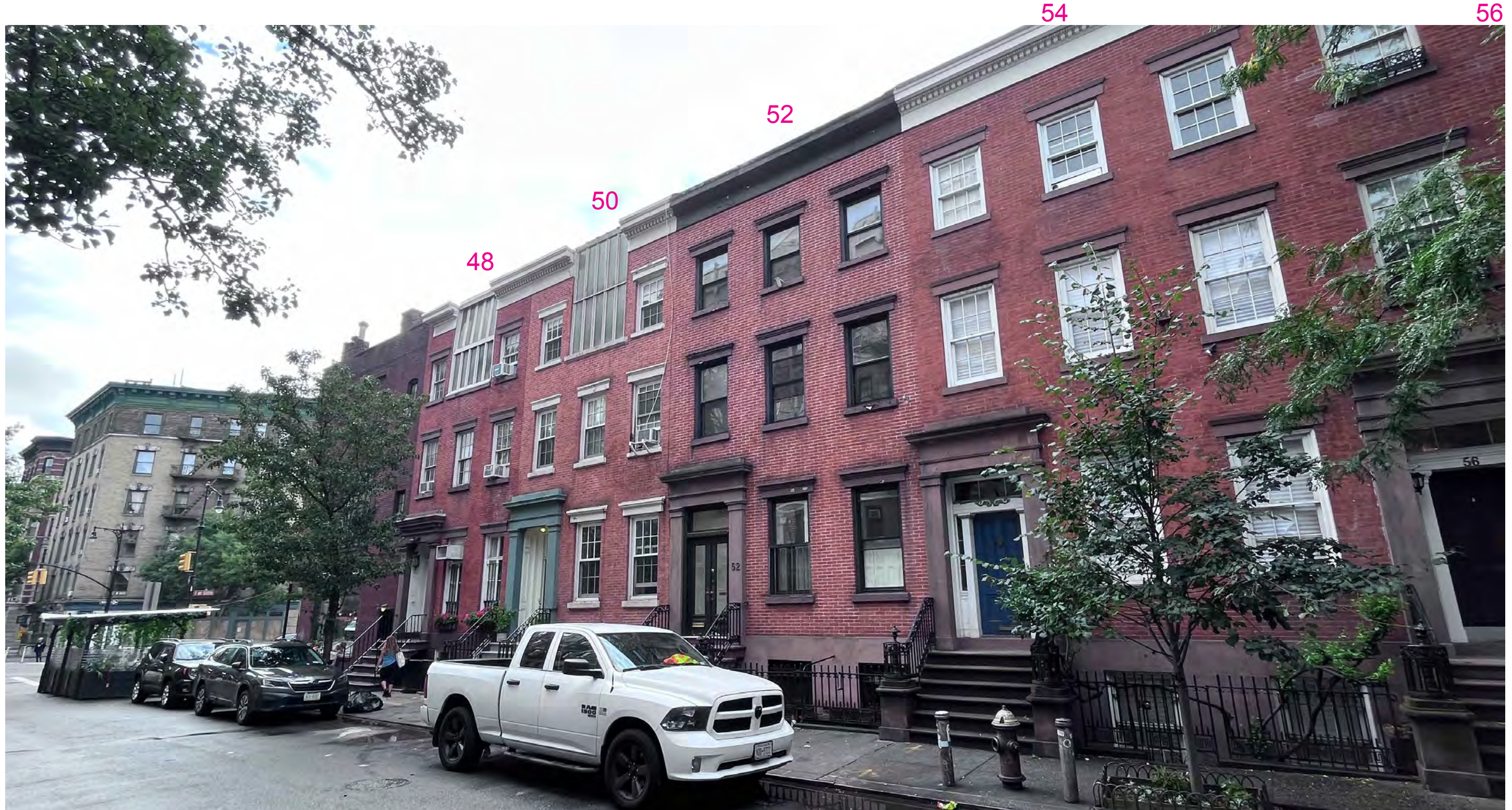
52 Charles Street in its row context, looking southeast toward Seventh Avenue South.
