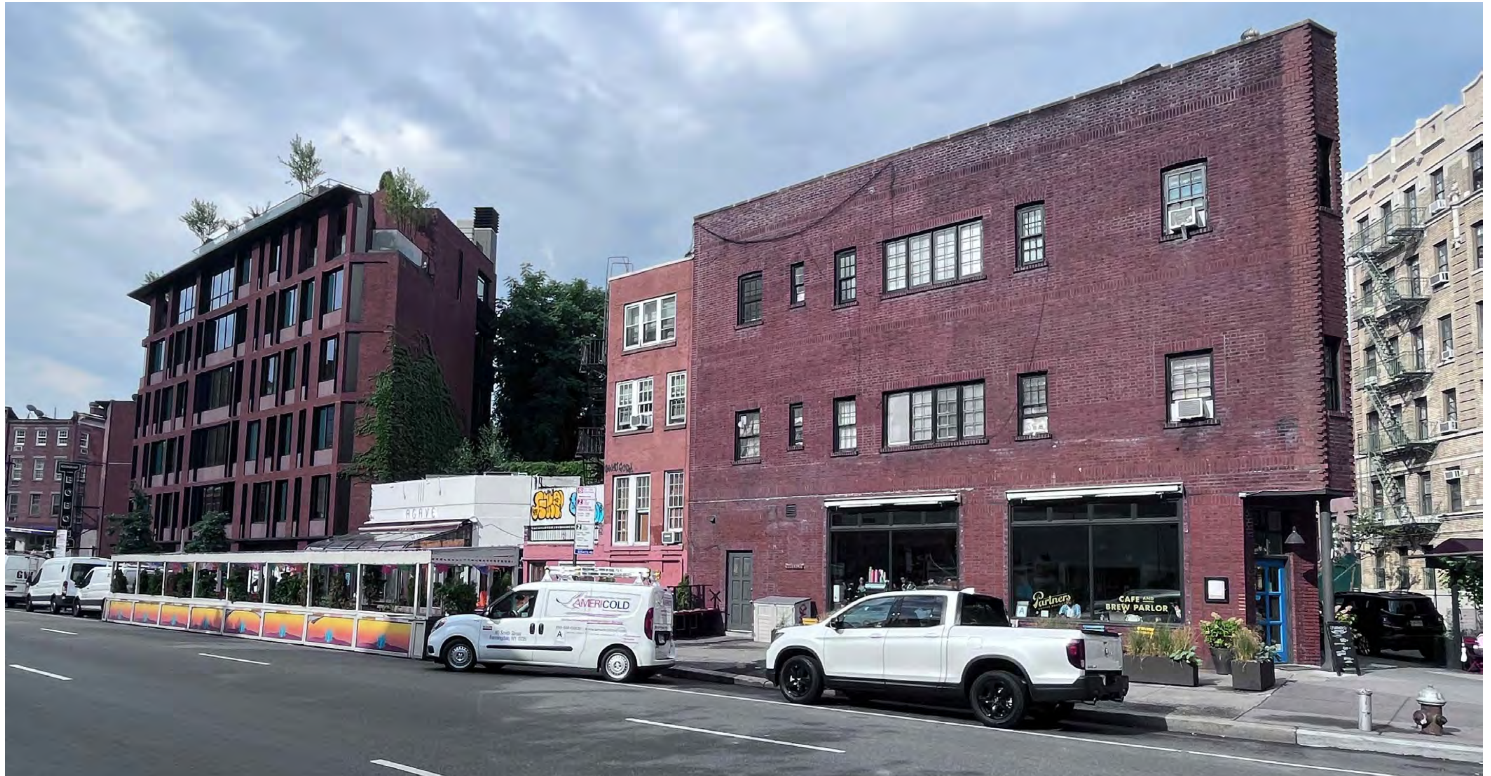
View to west side of Seventh Avenue South from corner of Charles Street. At right is 46 Charles Street, abutted by the altered rear of the row house at 48 Charles Street.
