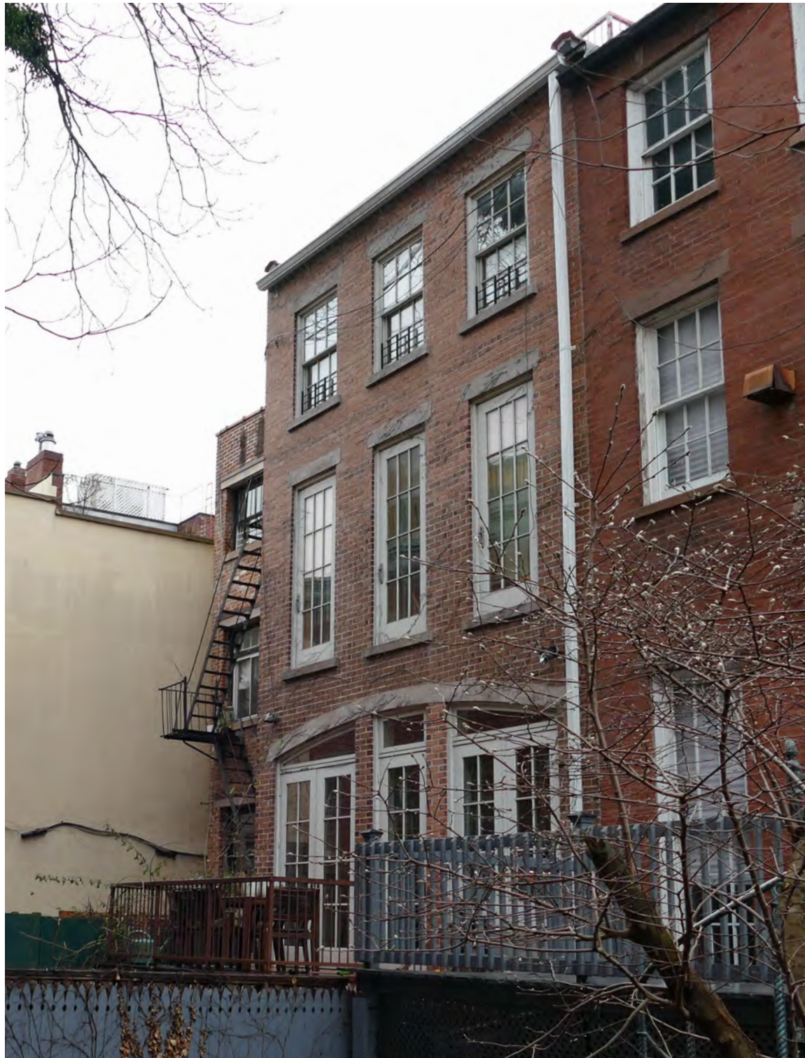
56 Charles Street: Rear addition, approved 2008.
