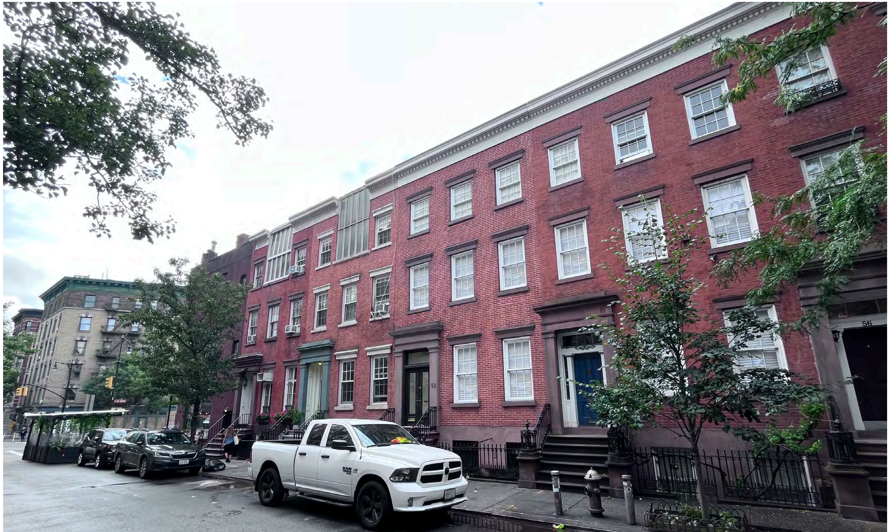
Rendering of proposed work at 52 Charles Street within its row, looking southeast toward Seventh Avenue South.
