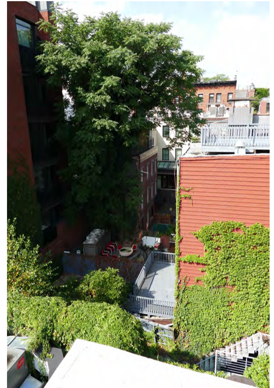
7 View to west of block interior from roof of 48 Charles Street.
