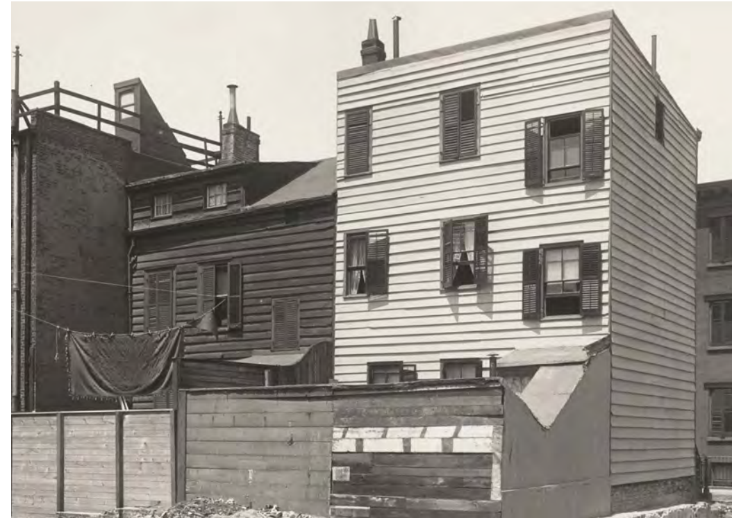
39-41 Barrow Street during the construction of Seventh Avenue South in 1914, prior to alteration. (New-York Historical Society)
