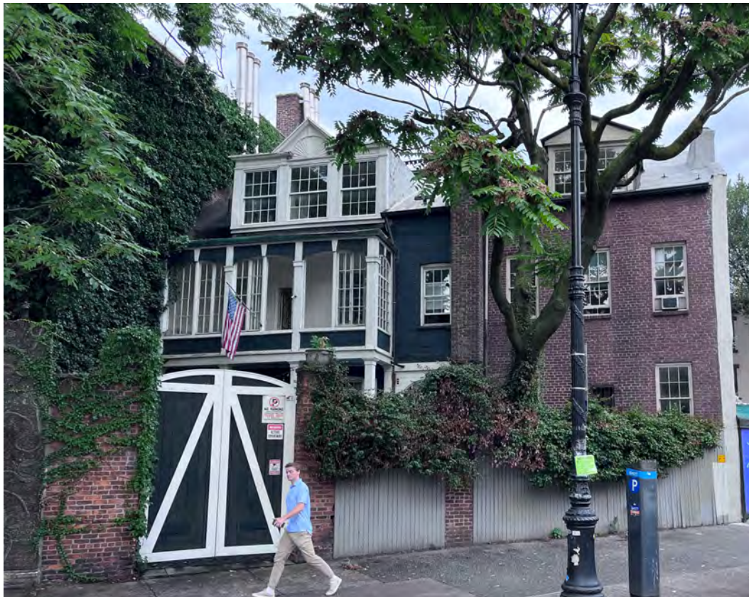
18 Commerce Street in 2023, with 1920 rear Colonial Revival alteration.
