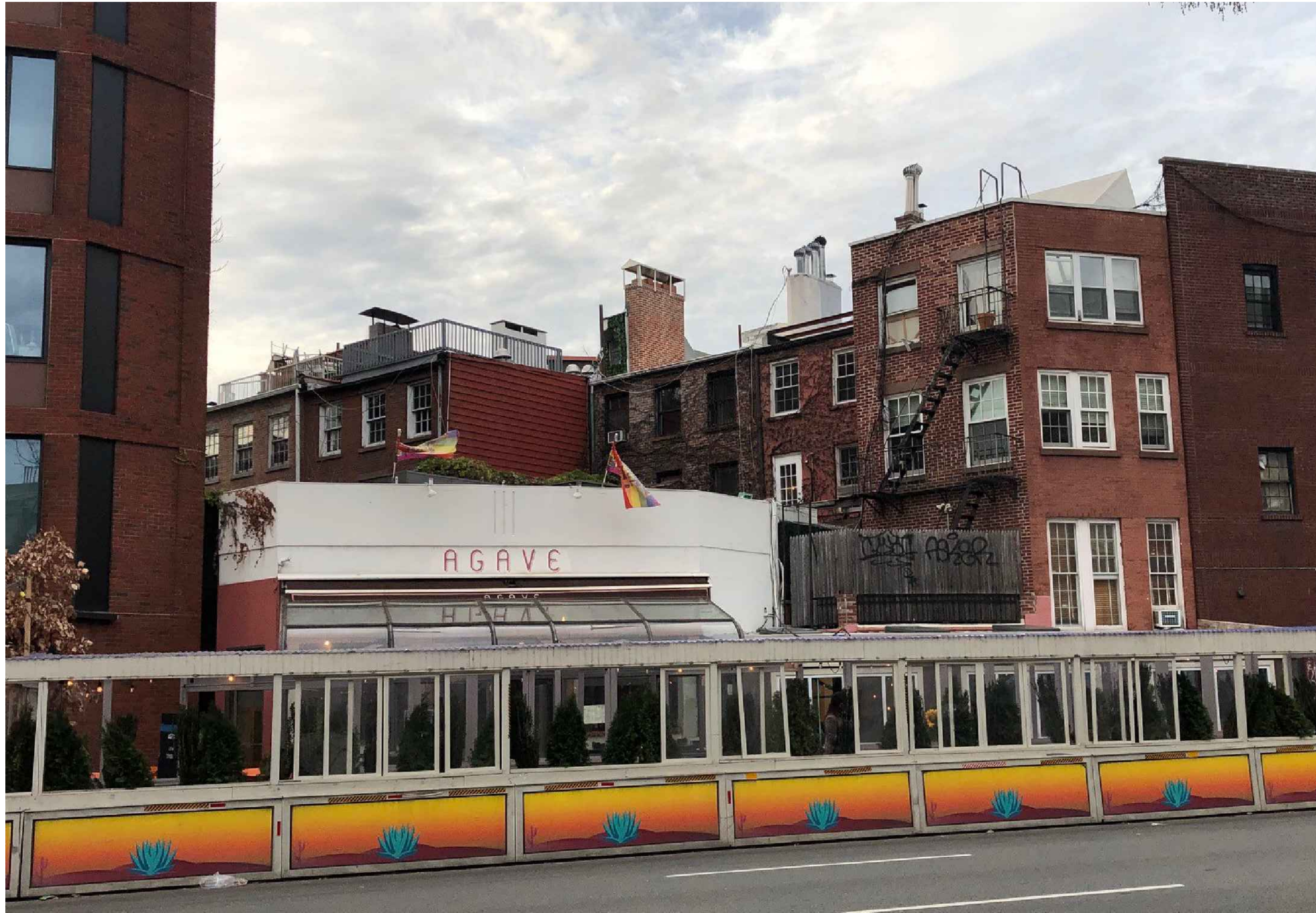
1 EXISTING: 7TH AVE PHOTO N.T.S.
