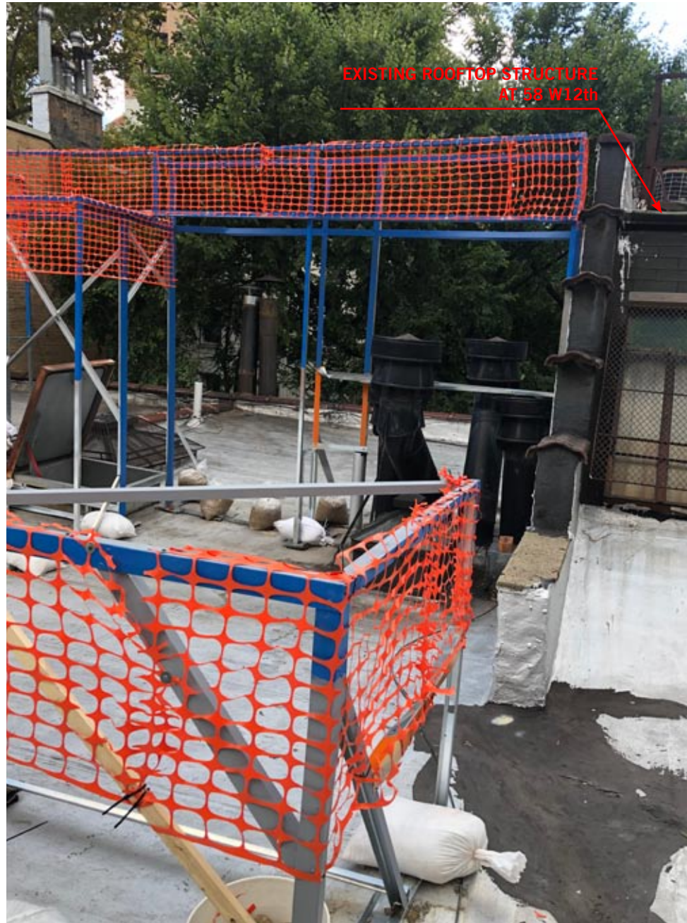
VIEW FROM ROOF LOOKING SOUTH
