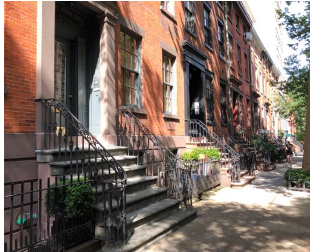
4: ROWHOUSES ON W11th STREET
