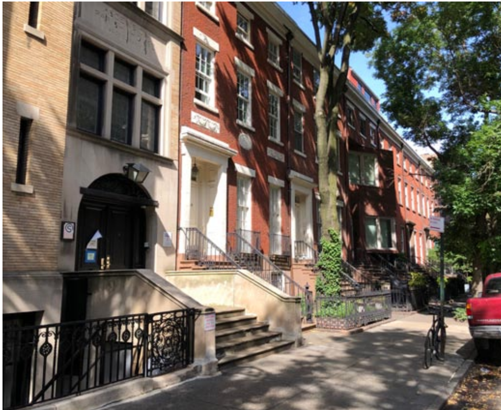
3: ROWHOUSES ON W11th STREET
