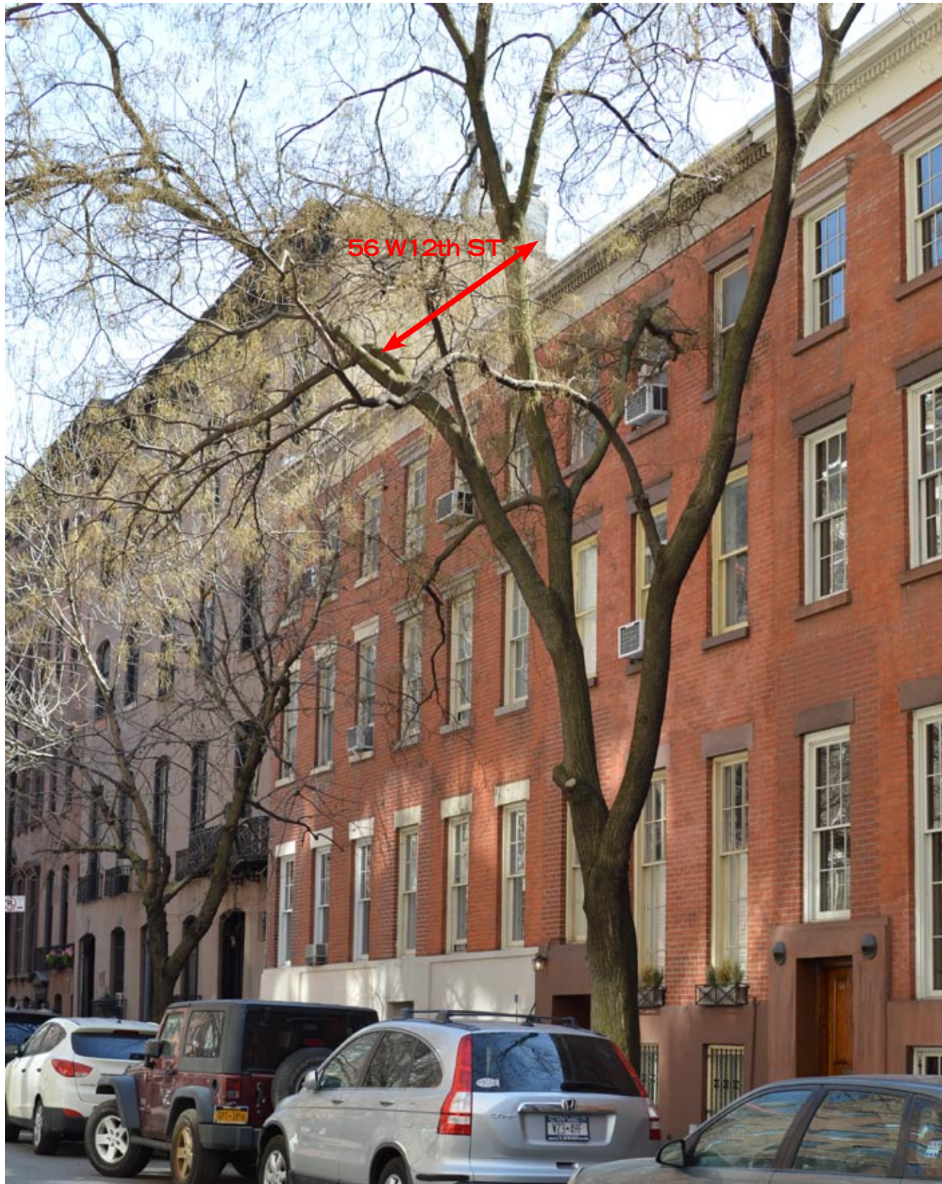
EXISTING BUILDING - VIEW FROM W12th STREET LOOKING SOUTHEAST
