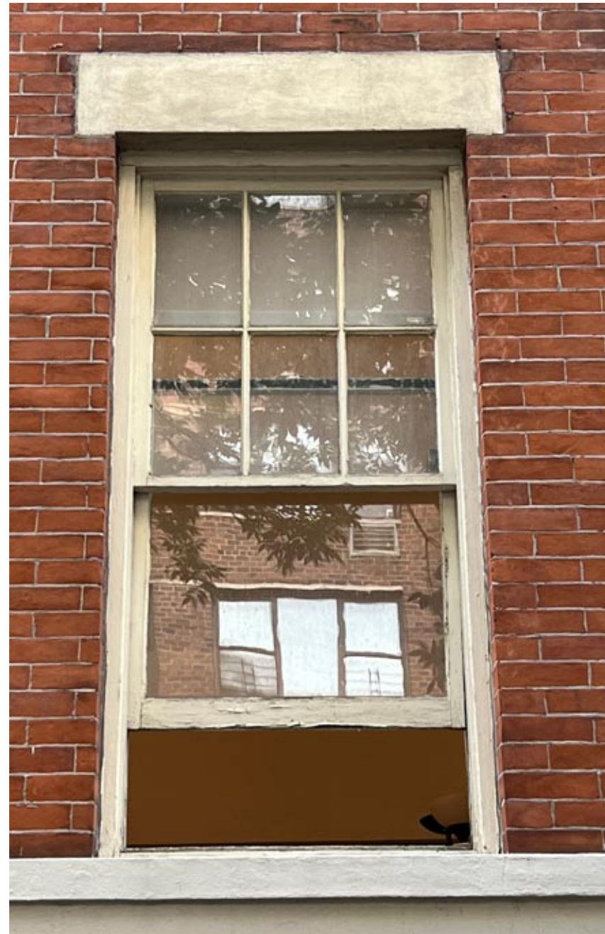
EXISTING FRONT FACADE WOOD WINDOW
