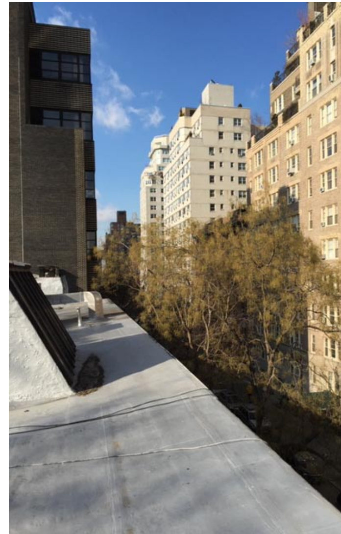
VIEW ACROSS STREET LOOKING WEST
