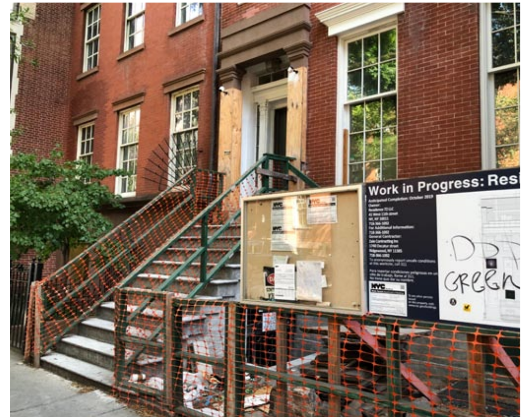
12: 41 WEST 11th STREET - UNDER CONSTRUCTION
