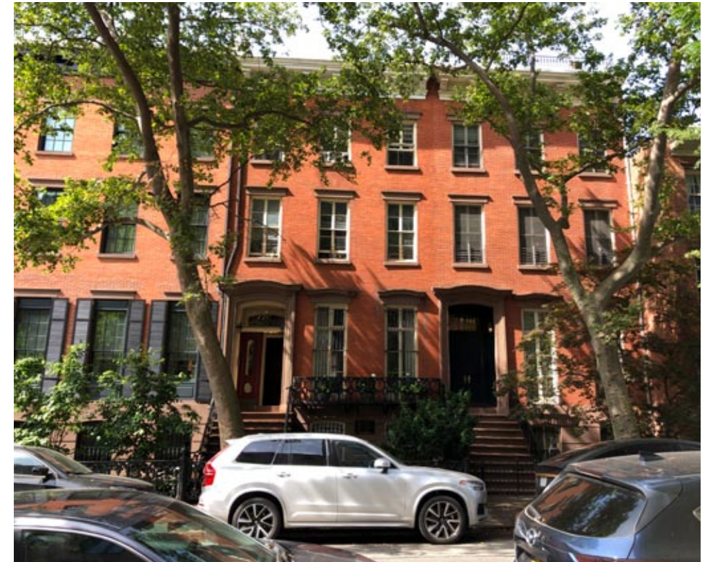
5: ROWHOUSES ON W11th STREET
