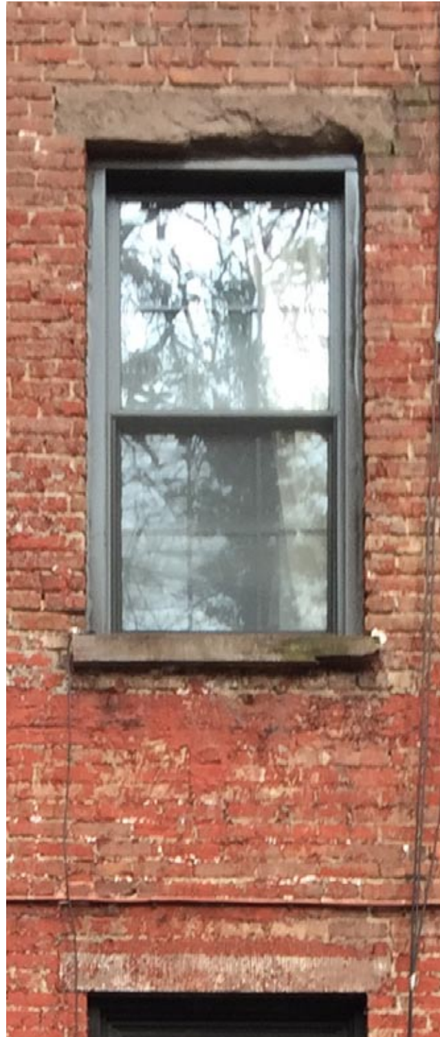
56 W12th - EXISTING ALUMINUM WINDOWS
