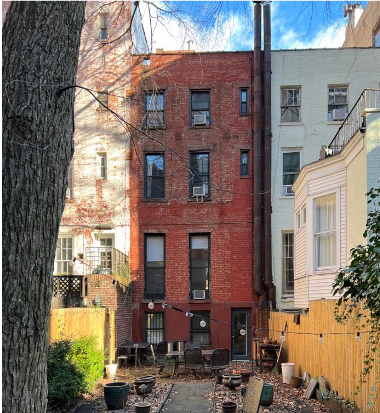
EXISTING REAR FACADE
