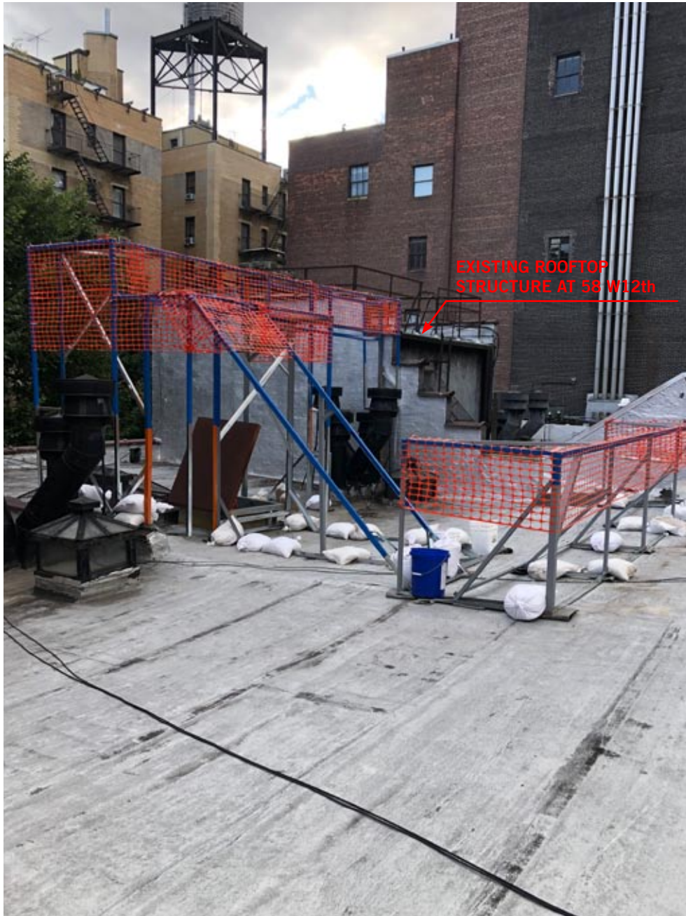
VIEW FROM ROOF LOOKING WEST
