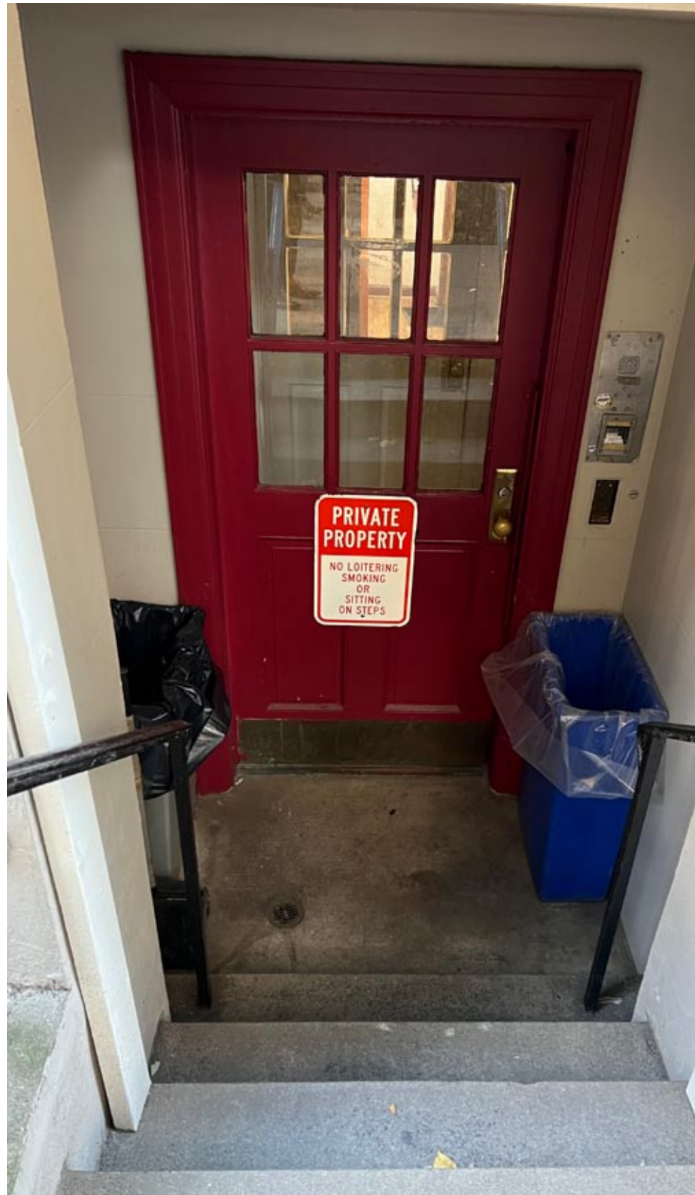
EXISTING ENTRY AND STEPS
