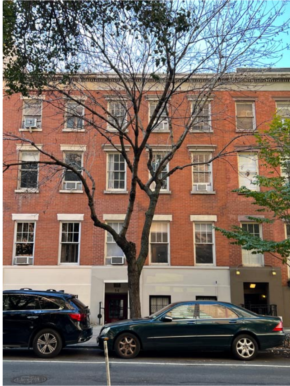
LOCATION D VIEW FROM 49 W 12th STREET LOOKING SOUTH
