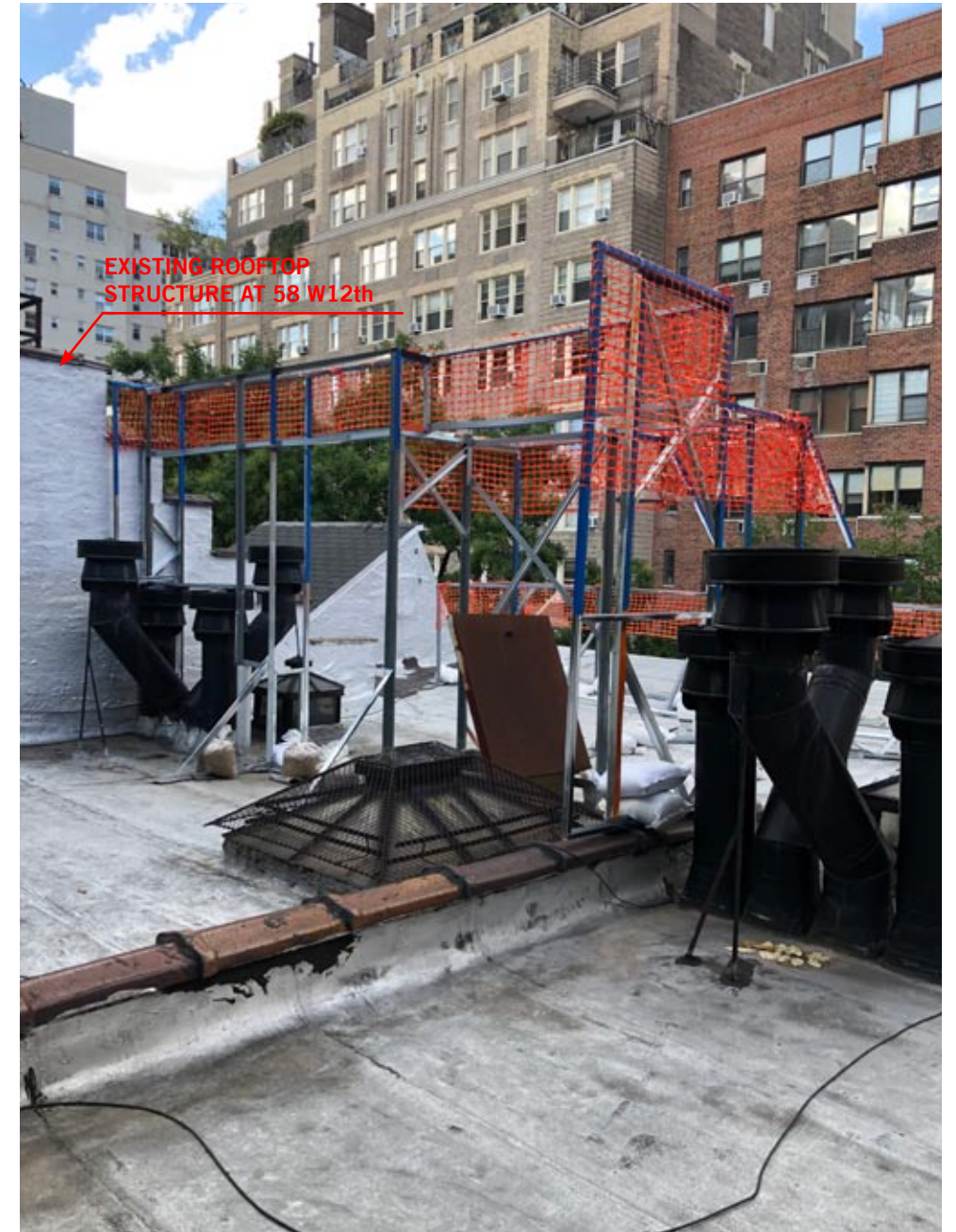
VIEW FROM ROOF LOOKING NORTHWEST
