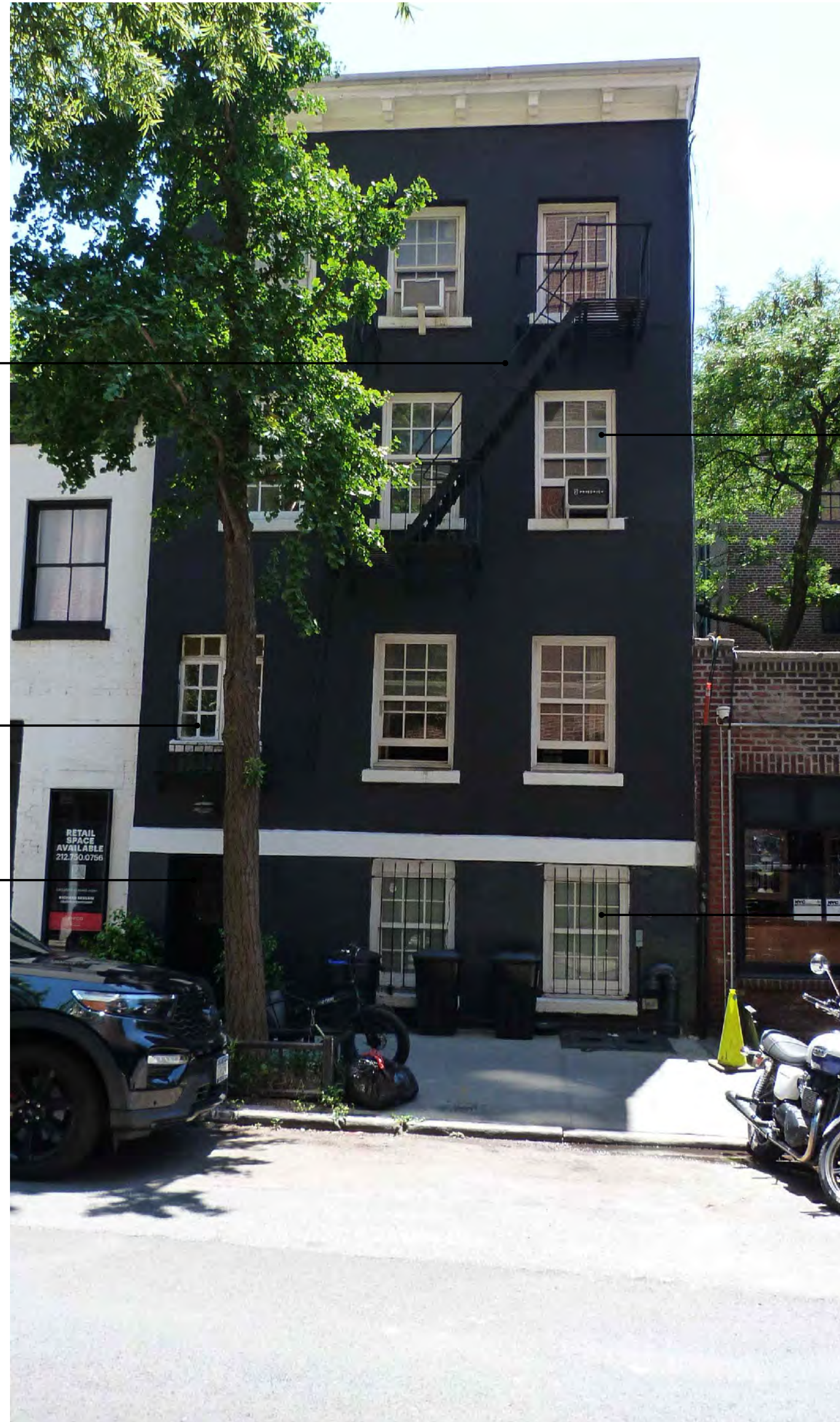
PHOTO EXISTING FACADE 32 JANE ST. N.T.S.
