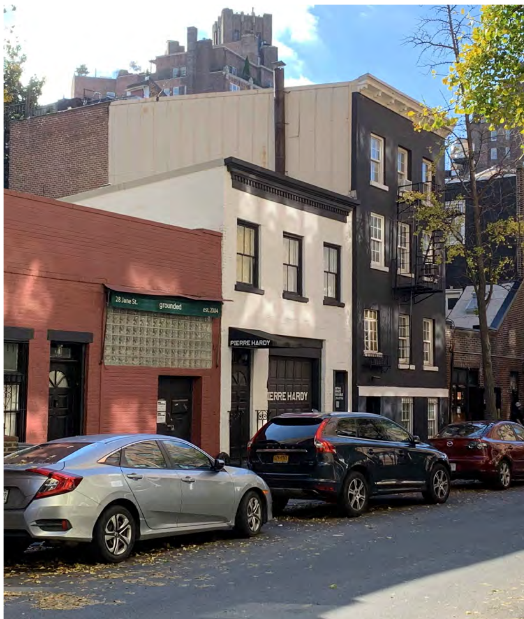
PHOTO 32 JANE ST. EAST FACADE REAR DETL. N.T.S.
