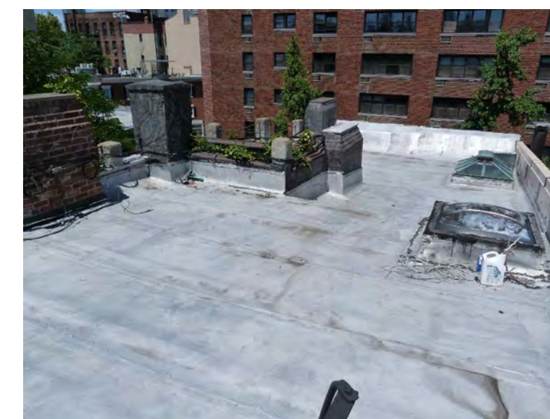
PHOTO 32 JANE ST. ROOF FACING NORTH N.T.S.
