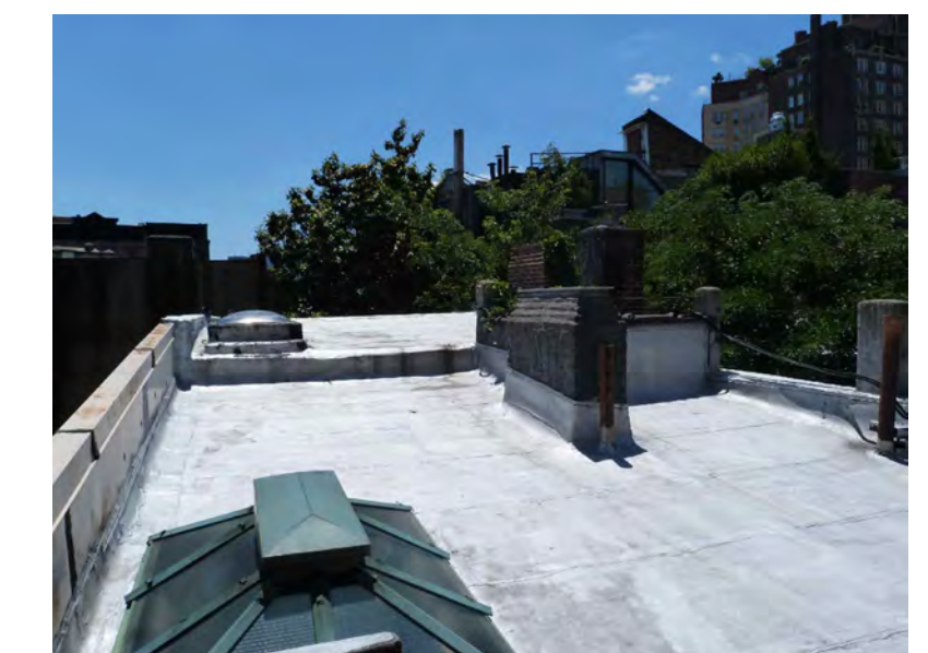
PHOTO 32 JANE ST. ROOF FACING SOUTH N.T.S.
