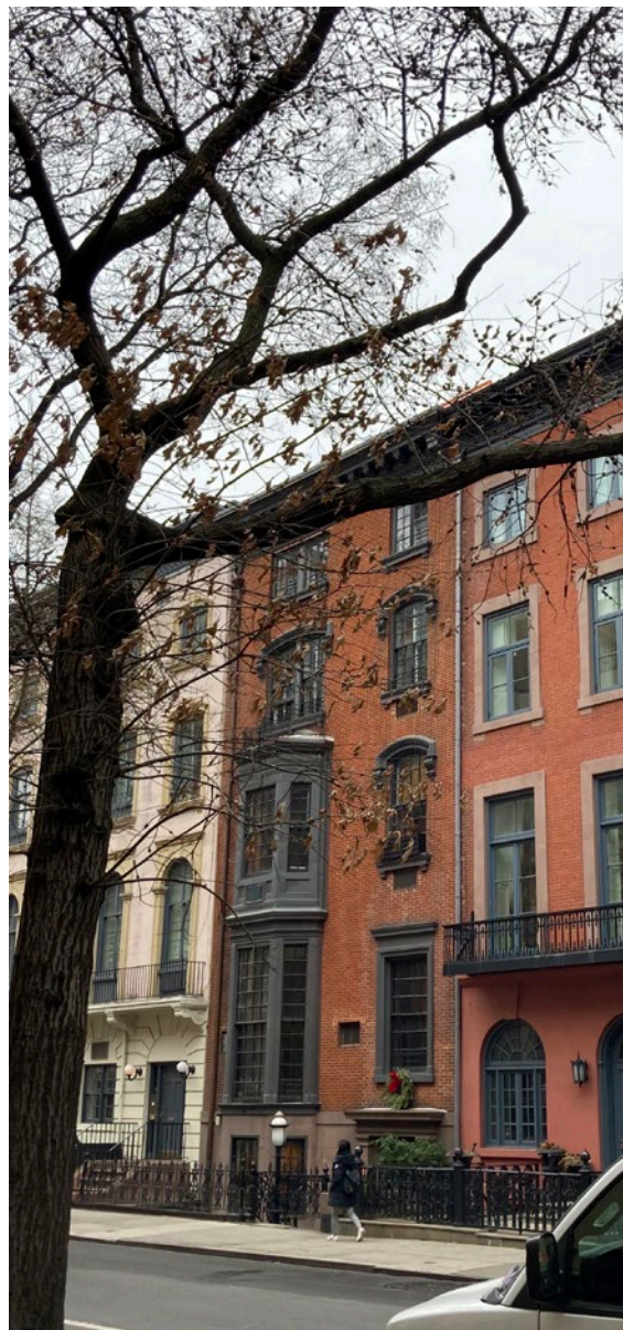
Location 4 Taken from 12 West 9th Street
