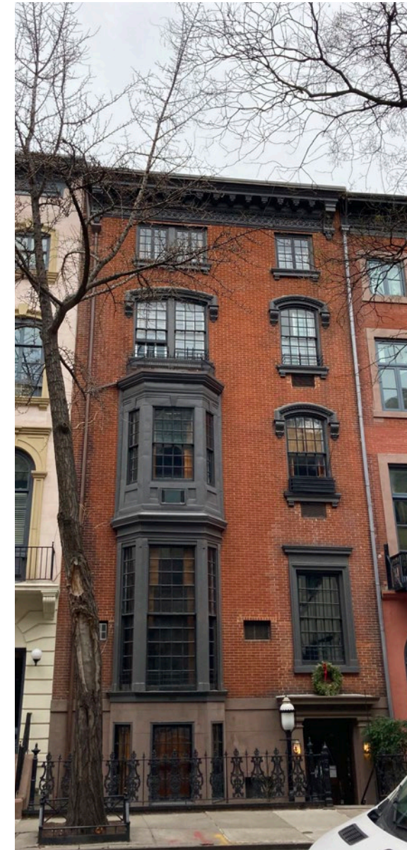
Location 3 Taken from 18 West 9th Street
